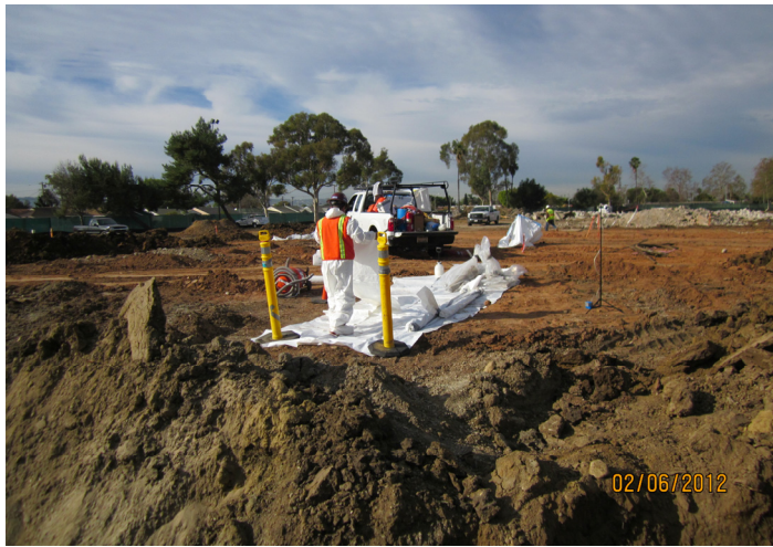
Transite Pipe Removal
