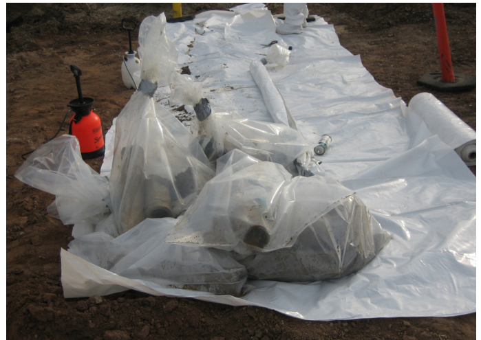
Secured Transite Pipe
