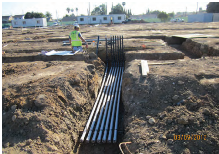
Underground Electrical Installation
