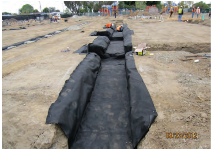
Methane Felt Installation
