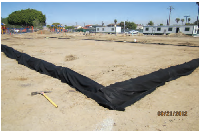
Methane Perforated Pipe Installation
