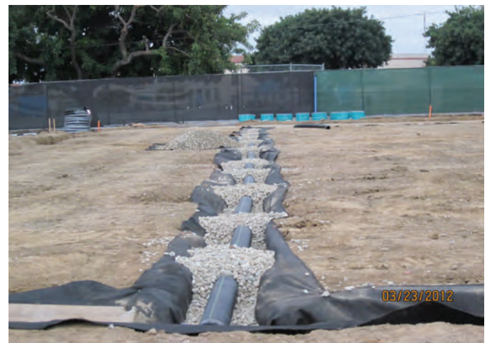
Methane Perforated Pipe Installation
