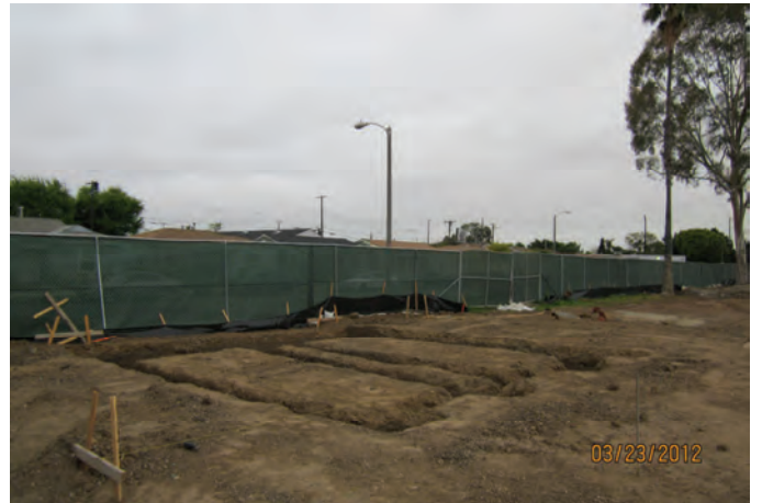
Remote Restroom Footing Excavation
