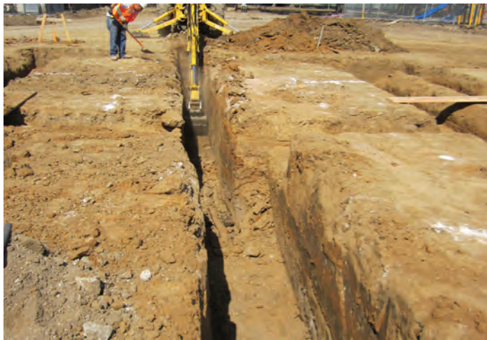
Methane Gas Mitigation Trenching
