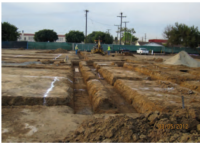
Recreation Building Footings
