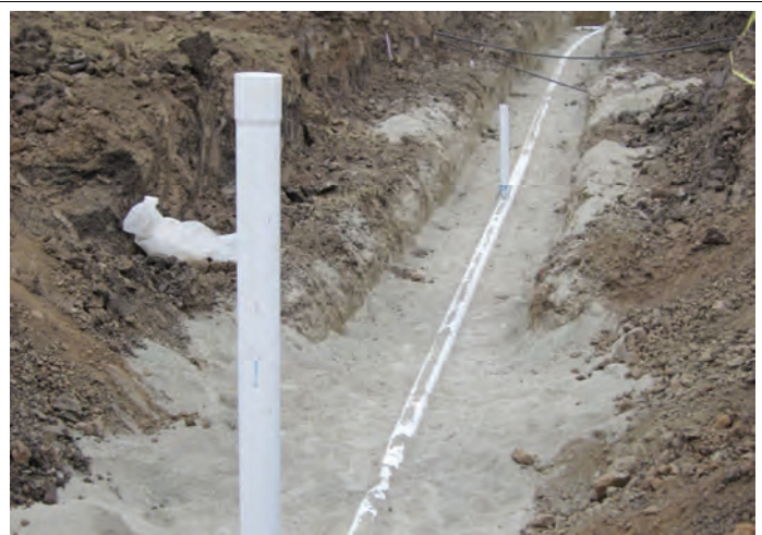
Main Sewer Pipe Installation
