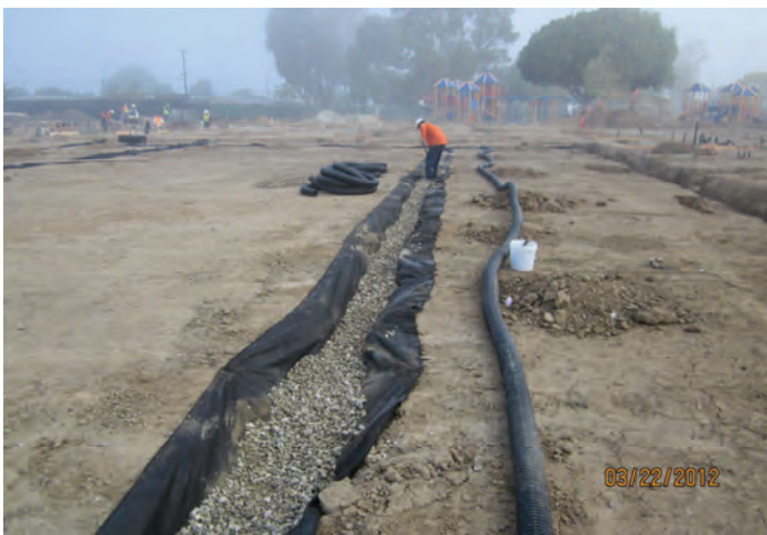
Methane Perforated Pipe Installation
