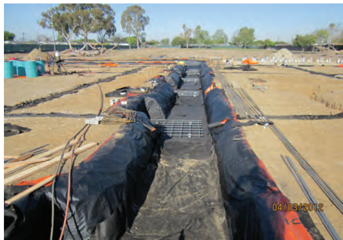
Reinforcement of Recreation Bldg Footings
