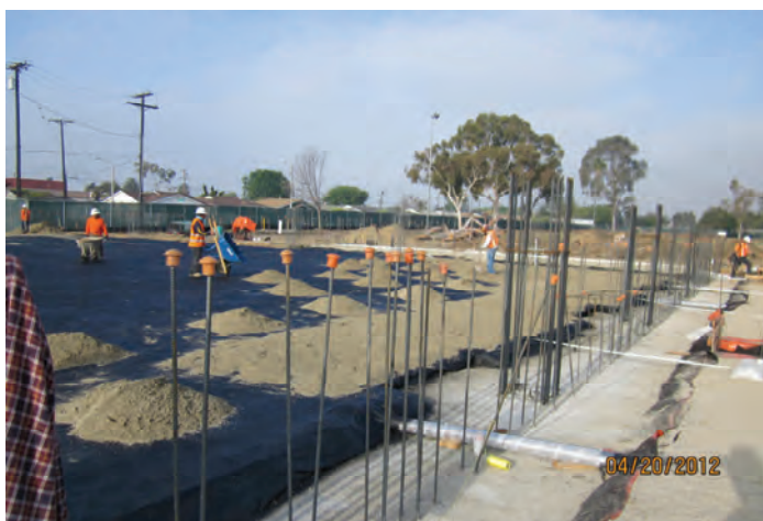
Sand Layer & Concrete Footings @ Gym Area
