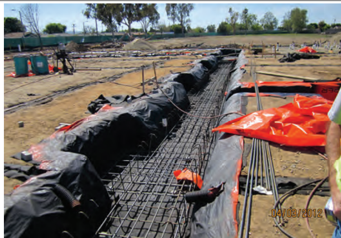
Reinforcement of Recreation Bldg Footings
