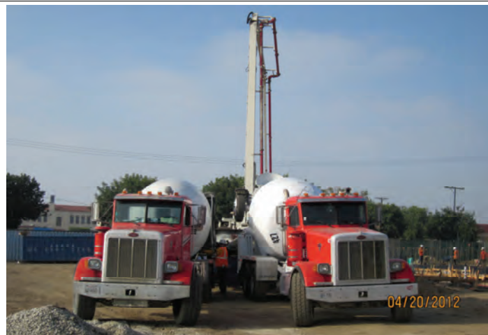
Concrete Footings Being Poured at Recreation Bldg
