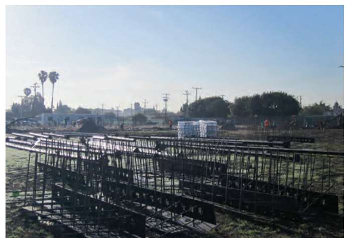
Structural Steel Delivered for Rec. Bldg
