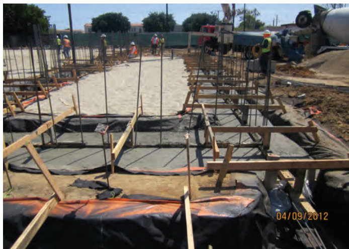
Concrete Footings Poured at Recreation Bldg
