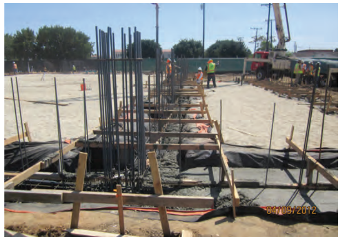
Concrete Footings Being Poured at Recreation Bldg
