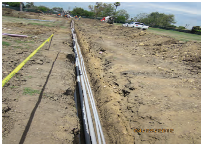
Field Underground Electrical Installation
