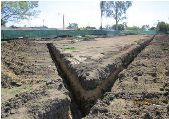
Field Underground Electrical Trenching
