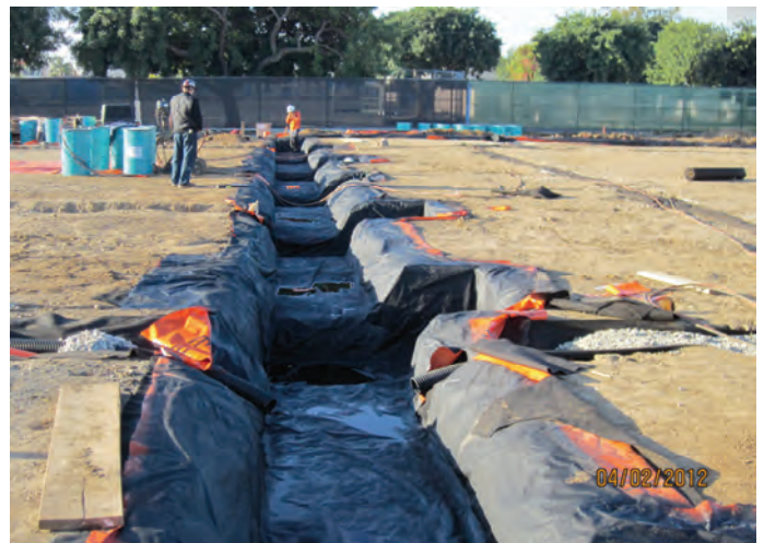
Methane Gas Mitigation in Recreation Bldg Footings
