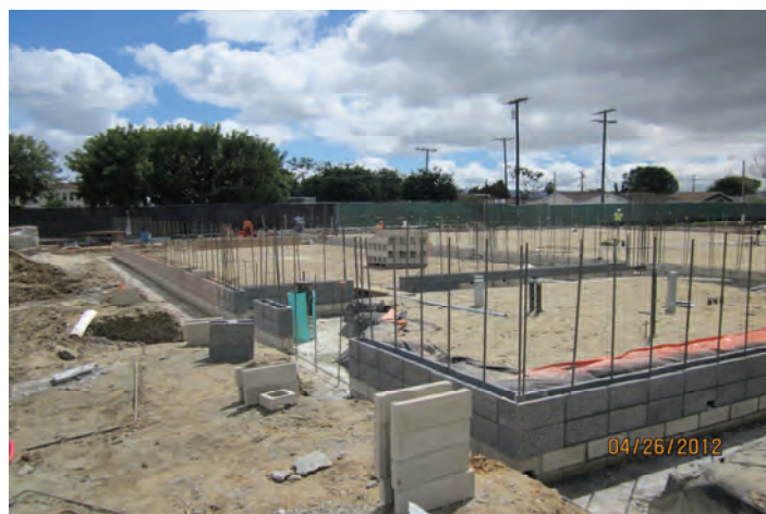
CMU Starter Walls (Recreation Bldg)
