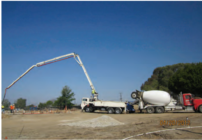
Concrete Footings Being Poured at Recreation Bldg
