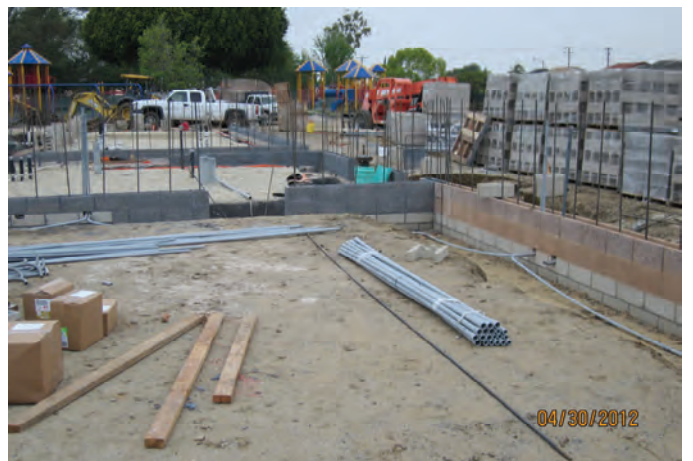
CMU Starter Walls (Recreation Bldg)
