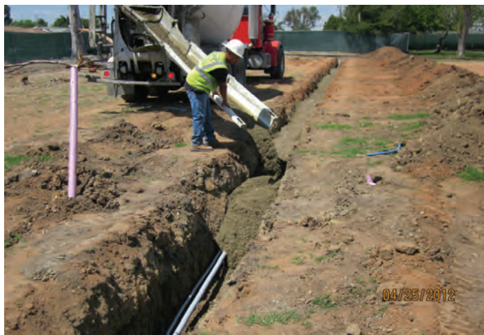
Backfill of Field Underground Electrical Trench
