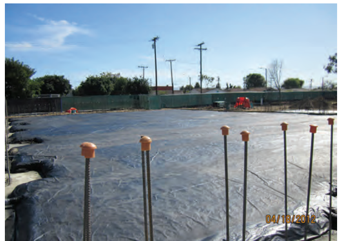
Asphaltic Layer of Methane Mitigation Syst. (Rec. Bldg)
