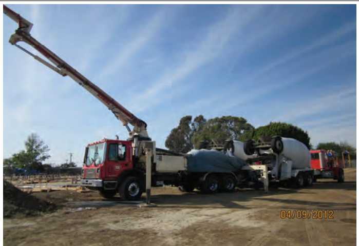
Concrete Footings Being Poured at Recreation Bldg
