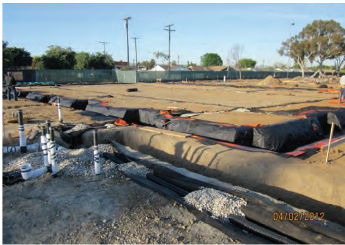
Methane Gas Mitigation in Recreation Bldg Footings
