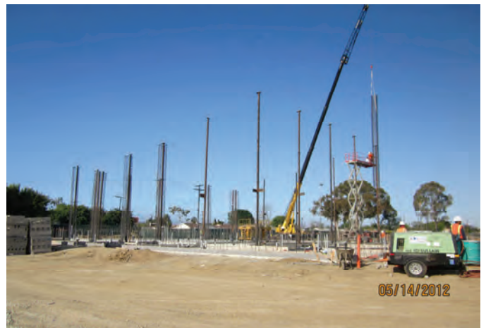
Rebar Cage Installation (Gym Area)
