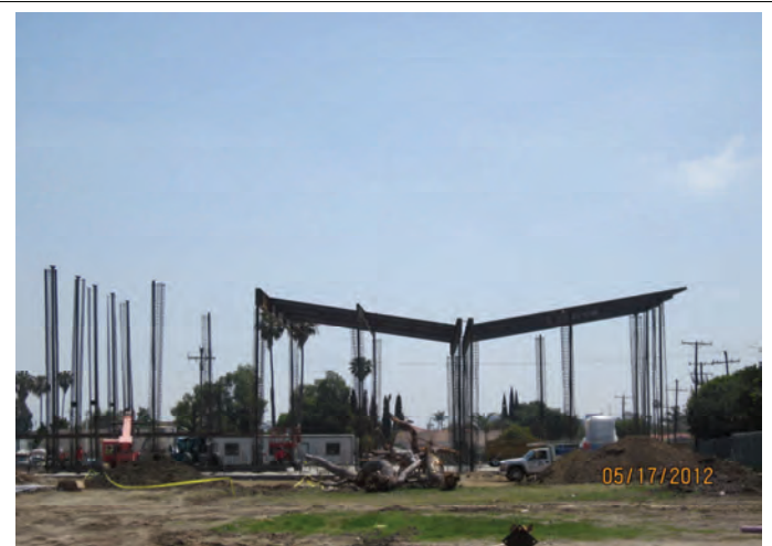
Beam Installation (High Roof)
