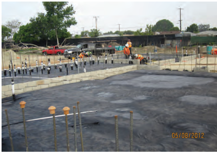
Felt Layer over Methane System (Remaining Areas)
