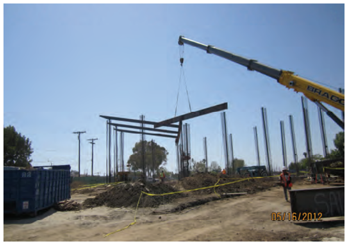
Beam Installation (High Roof)
