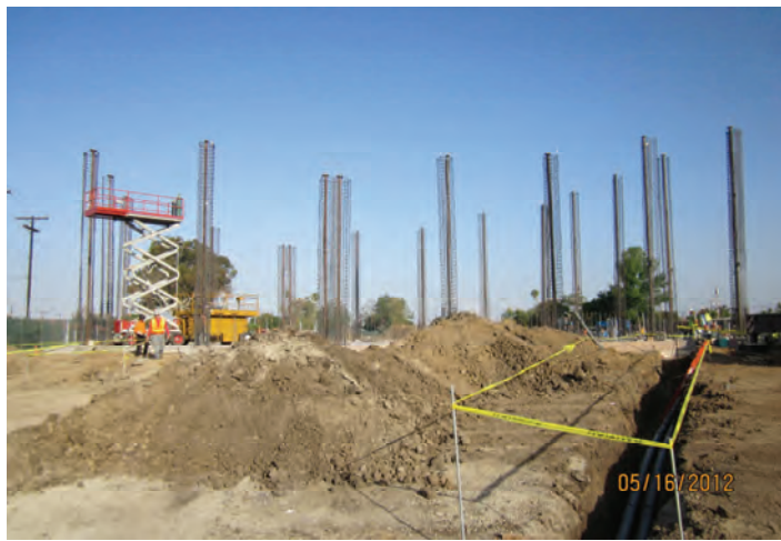
Completed Rebar Cage Installation (Gym Area)
