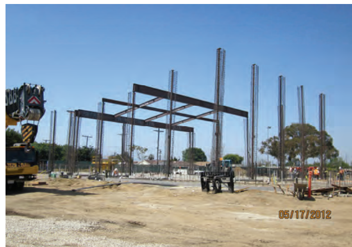
Beam Installation (High Roof)
