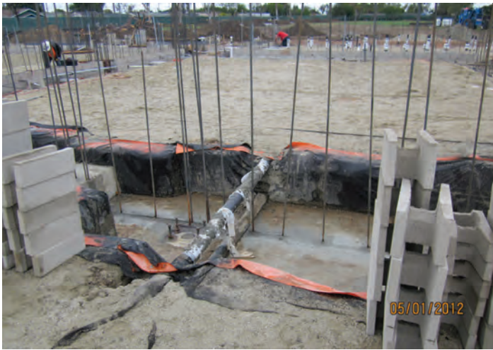
Sand Layer over Methane System (Remaining Areas)
