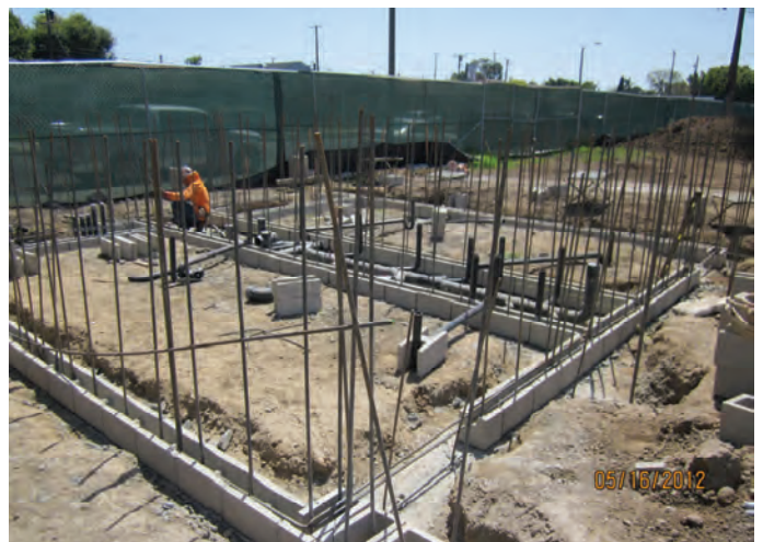
Restroom Bldg — Begin CMU Installation
