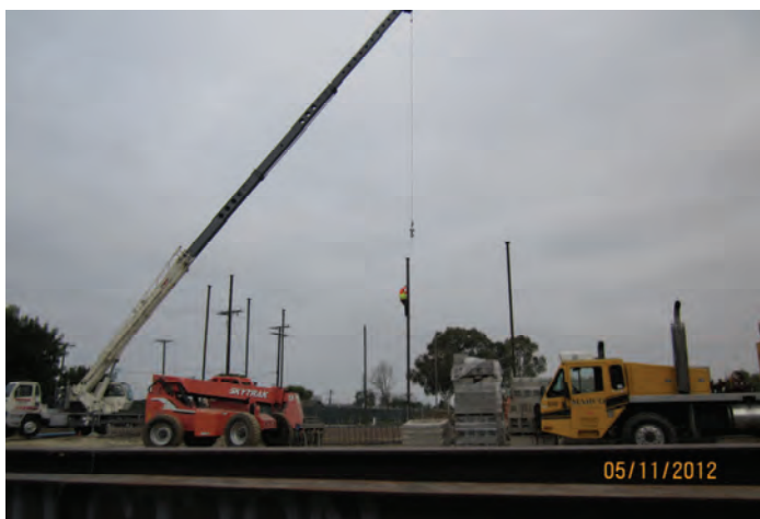
Column Installation (Gym Area)
