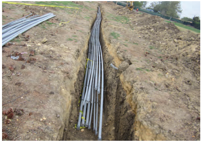
Site Underground Electrical Installation
