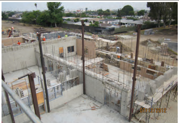
CMU Installation (Remaining Areas)
