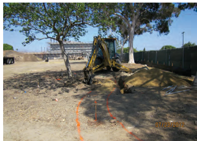
Seat Wall Trenching
