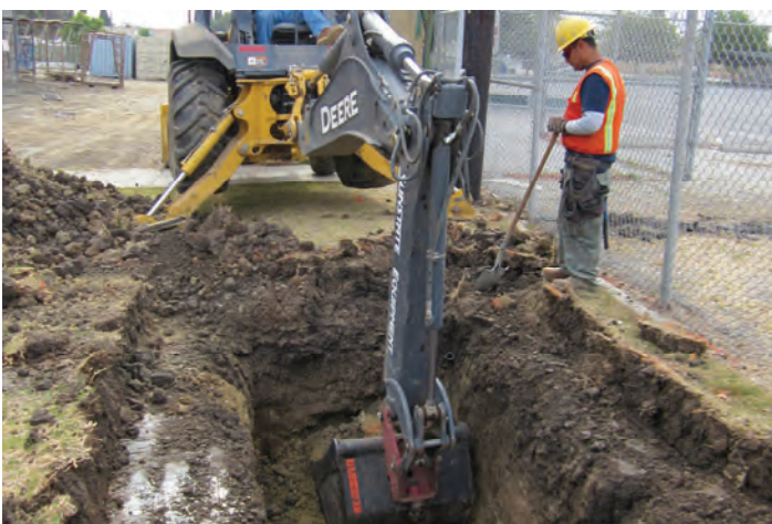
Catch Basin Trenching
