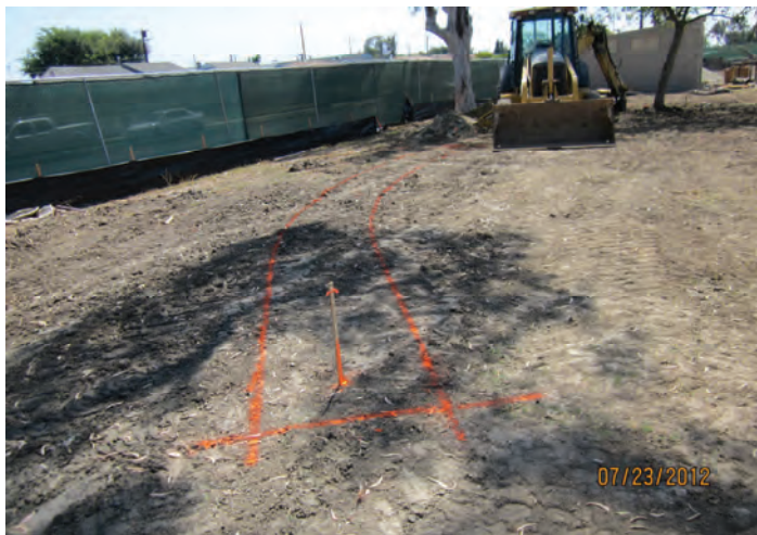
Seat Wall Preparations
