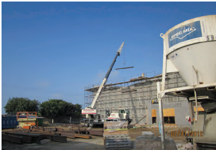
Steel for Roof Installation (Gym Area)
