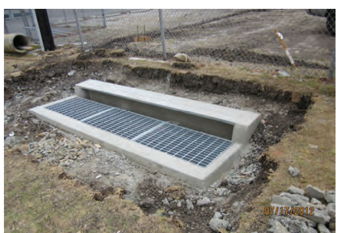
Completed Catch Basin Installation
