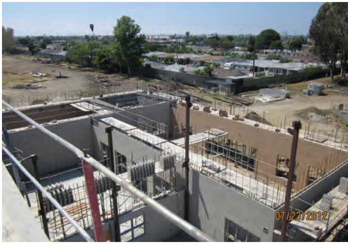
CMU Installation (Remaining Areas)
