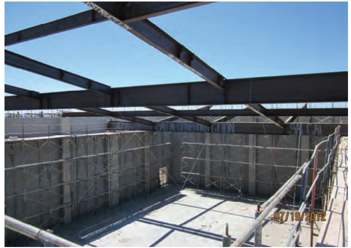
CMU Installation (Gym Area)
