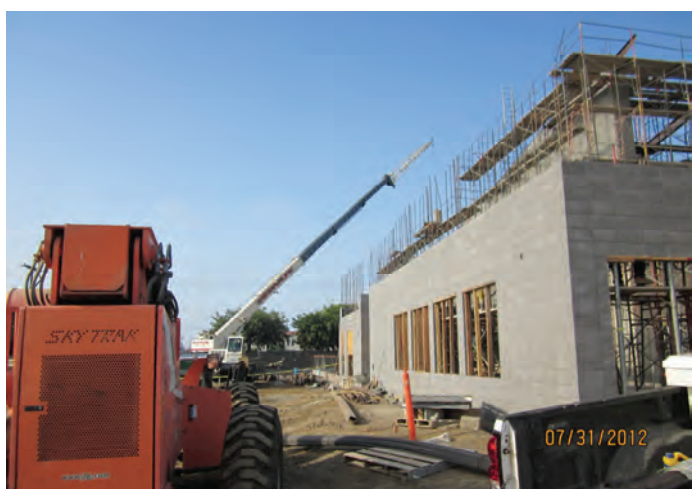
Steel for Roof Installation (Gym Area)
