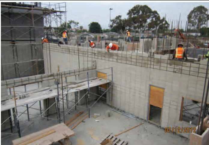
CMU Installation (Remaining Areas)
