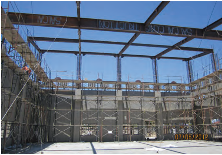
CMU Installation (Gym Area)
