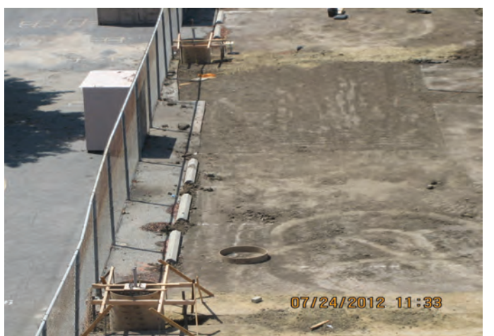
School Parking Lot Forming for New Lights
