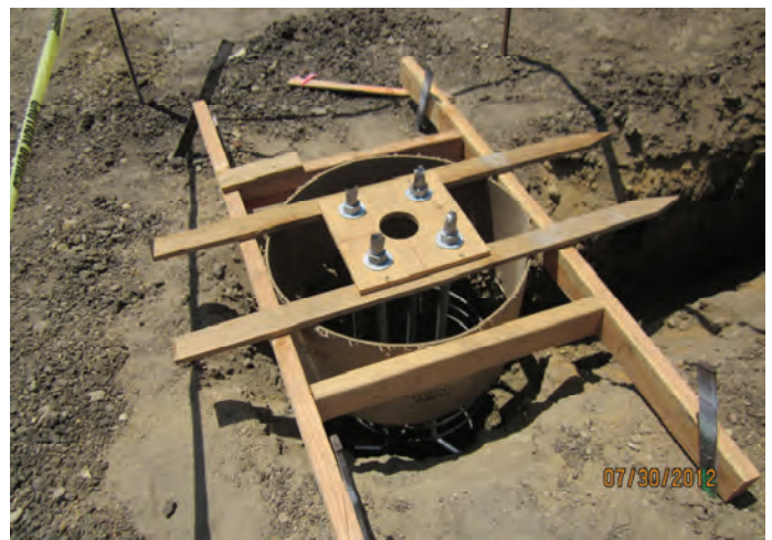
Forming for Light Pole Standards
