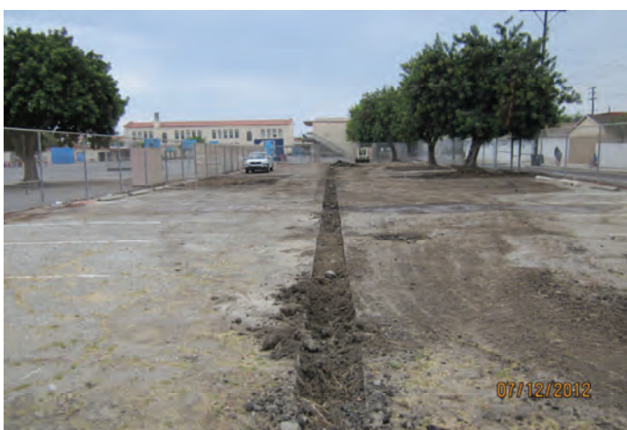
School Parking Lot Trenching for New Lights
