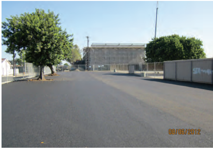
Paving Complete (School Parking Lot)
