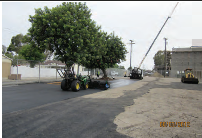
School Parking Lot Paving
