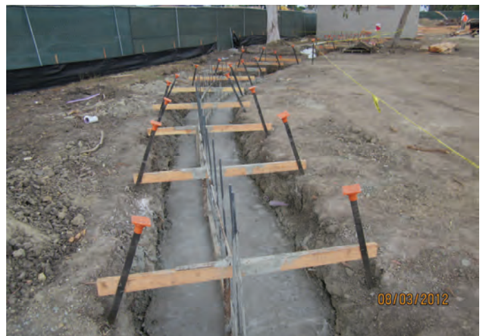
Poured Seat Wall Footings
