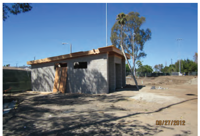
Completed Roof Framing (Restroom Building)
