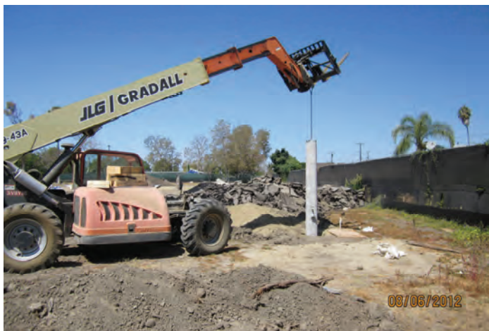
Musco Light Pole Base Installation
