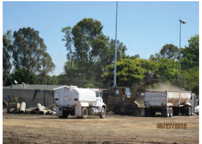
Debris Removal (Field)
