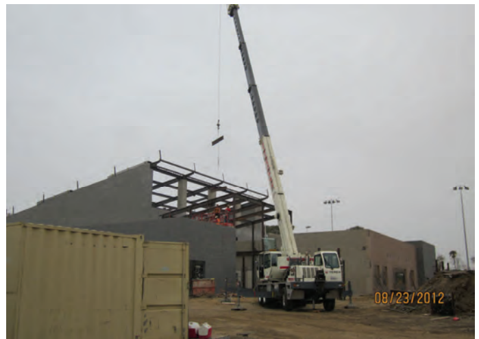
Beam Installation (Gym Area)
