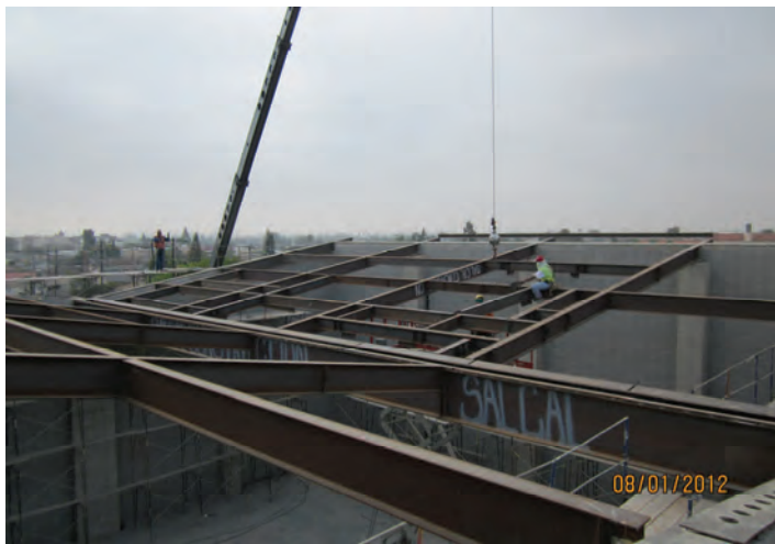
Beam Installation (Gym Area)
