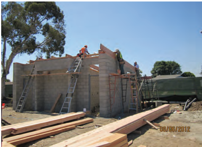
Roof Framing (Restroom Building)
