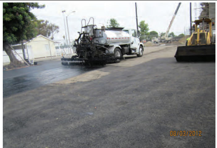
School Parking Lot Paving
