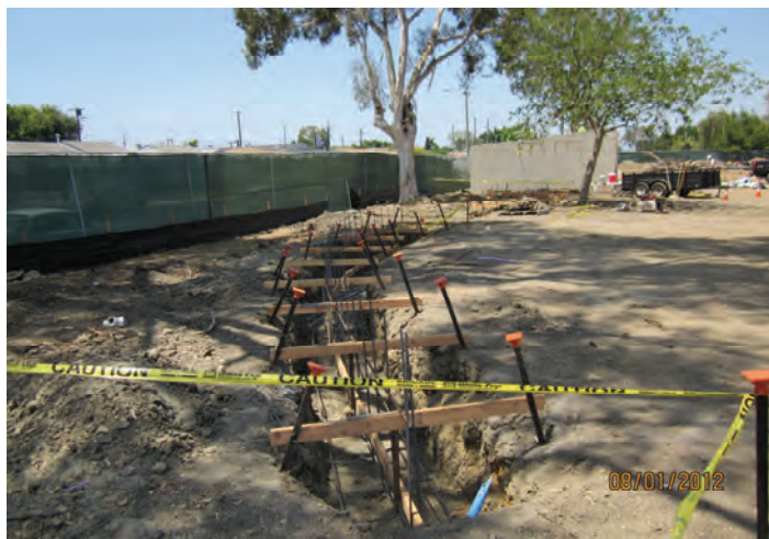
Seat Wall Preparation for Footings
