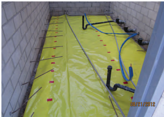
Vapor Barrier (Restroom Building)
