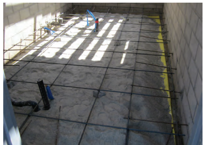
Sand / Rebar Over Vapor Barrier (Restroom Building)
