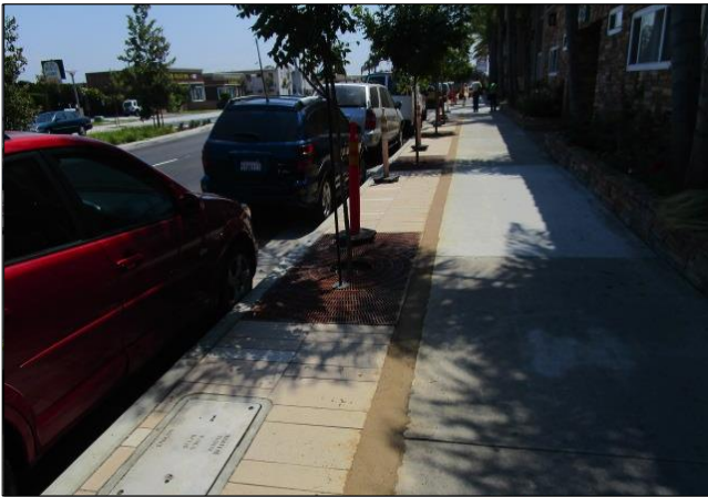
Placing decomposed granite in sidewalk of 1405k gaps.
