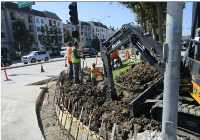
Trenching for traffic signal conduit relocation.
