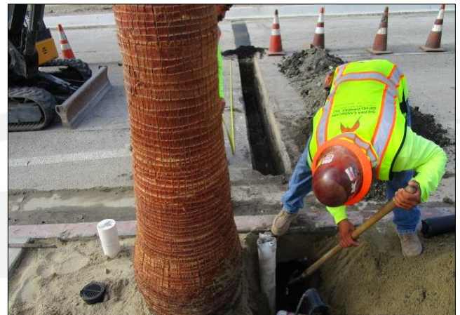
Connecting irrigation mainline crossing Carson.
