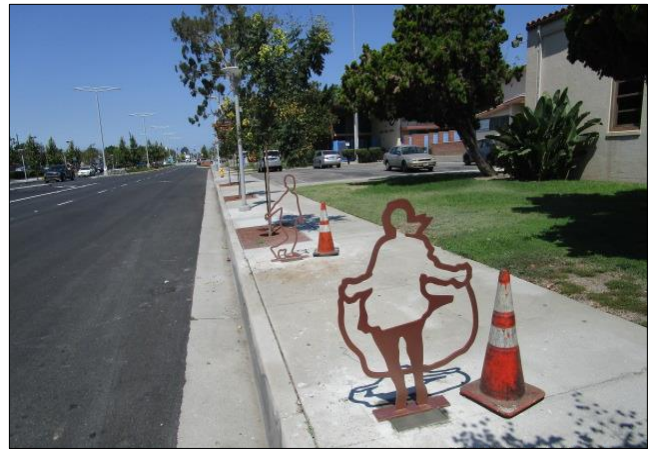
Bicycle racks installed in front of school.
