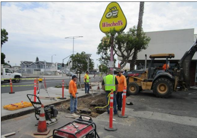
Removing section of driveway, crossgutter at Winchell's.
