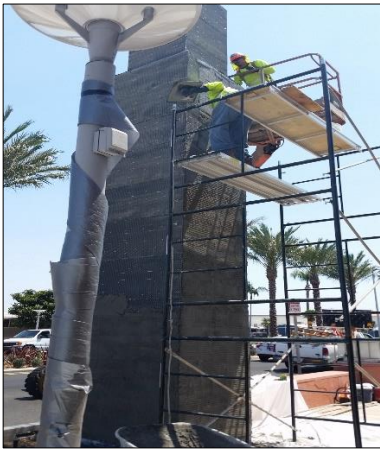
Eastbound Carson St. monument tower applying mortar.
