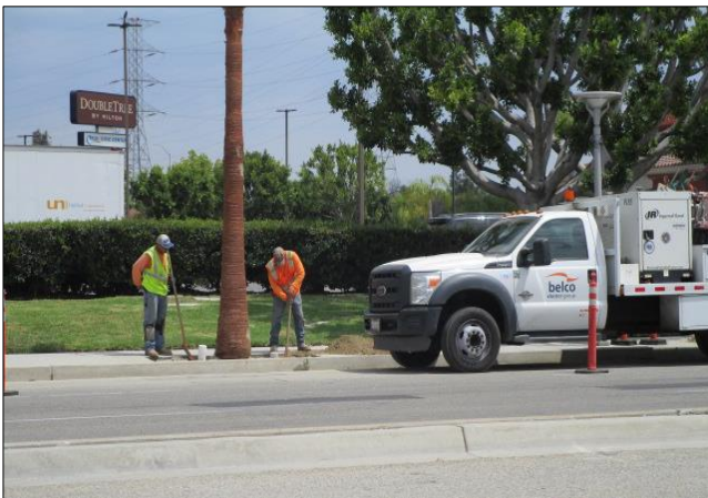
Belco installing uplighting for palm trees.
