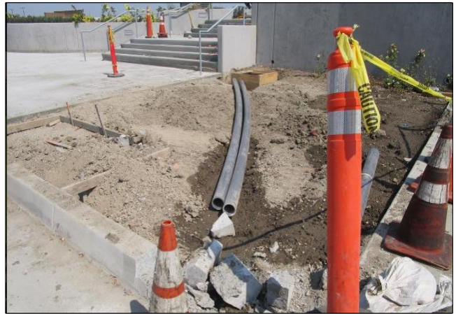
Trenching for pedestrian lighting at City Hall of Avalon.
