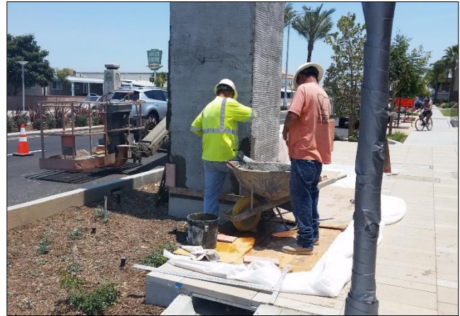
L. Johnson applies stone veneer to monument tower east bound Carson.
