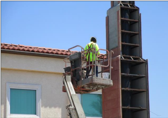
Placing stone tiles on monument tower.
