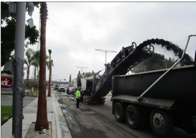
Coldmilling pavement east of Avalon.
