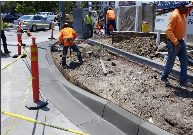
North west corner of Carson St. curb and gutter post placement.
