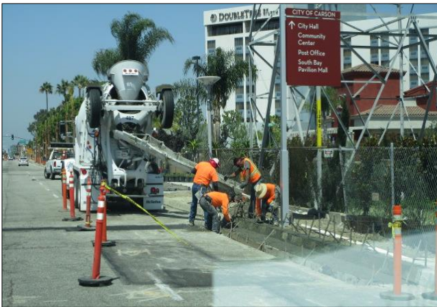
Placing curb and gutter west of I-405.
