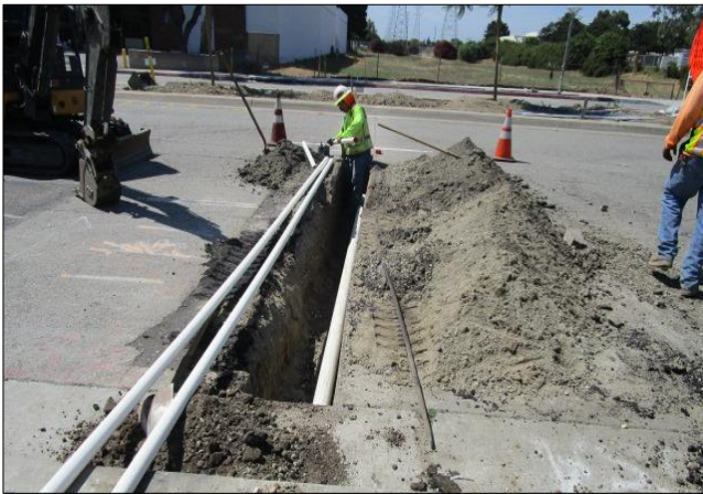
Installing irrigation mainline across Carson.
