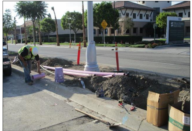
Installing irrigation mainline in median east of Avalon.
