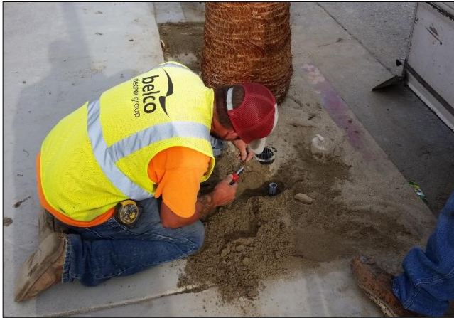
Palm tree upright installation.
