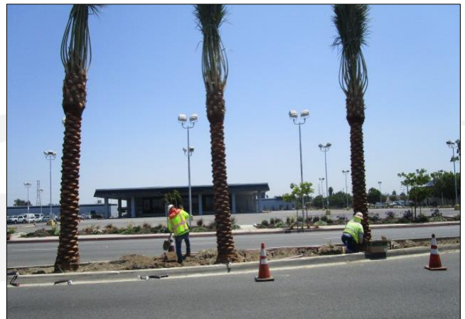
Installing sprinkler heads on Avalon median.
