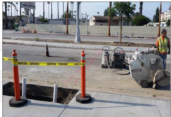
Sawcutting irrigation lateral at Carson St.
