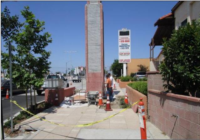
Placing stone on monument tower.
