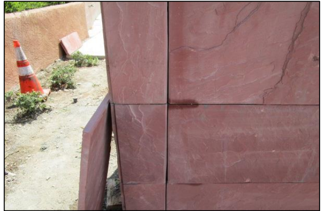
Joints between monument tower stone.
