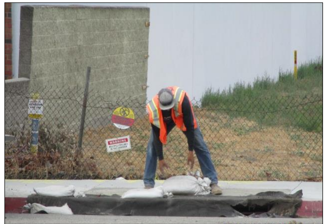
Placing fresh BMPs prior to cold mill and paving.
