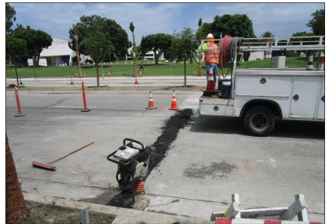
Trench across south side of Carson for irrigation mainline.
