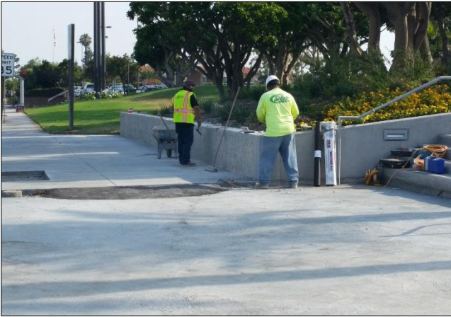
JBS Plaster established work area for stucco coat assembly.
