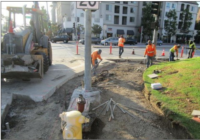
Grading and compacting for curb ramp south west corner of Carson and Avalon.
