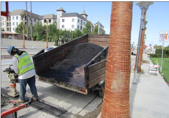
Permanent restoration to irrigation mainline trench.
