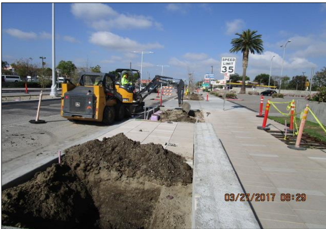
Excavating tree wells.
