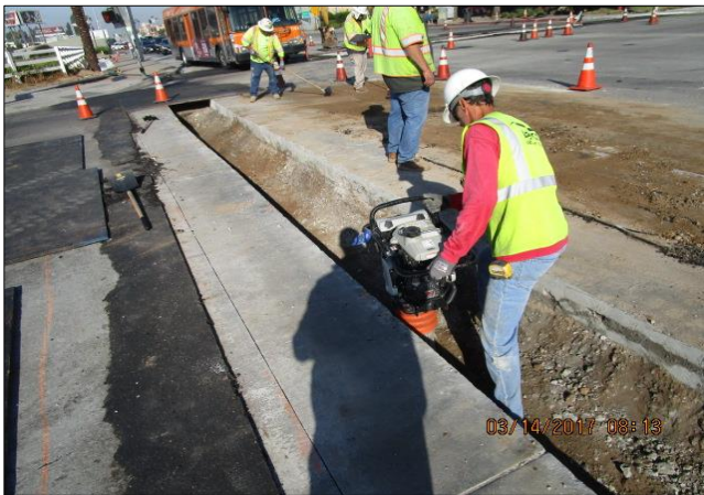
Compacting crushed misc. base in trench at Carson/Figueroa.
