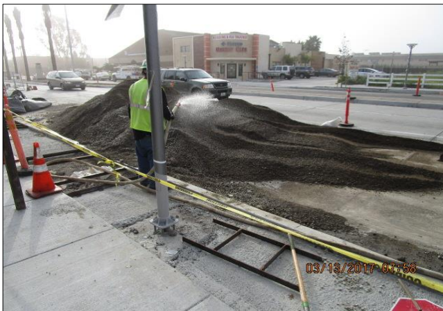
Powell stockpiling materials for Tuesday off-site haul.
