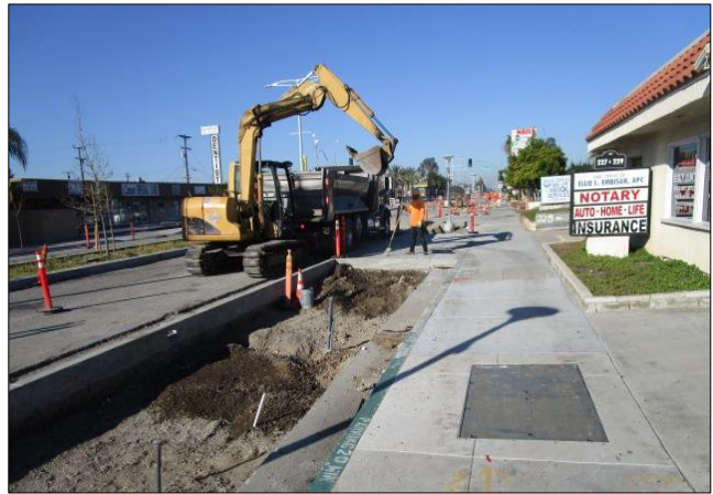
Removing unsuitable soil north side east of Moneta.
