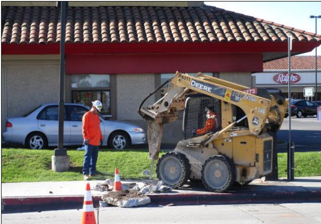
Demolition on southwest corner of Carson/Avalon.
