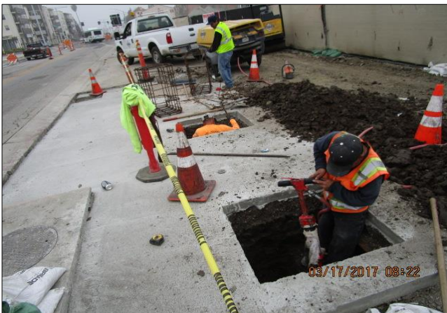
Excavating transit shelter foundation west of Avalon.
