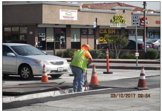
Potholing for utilities at Carson/Figueroa.
