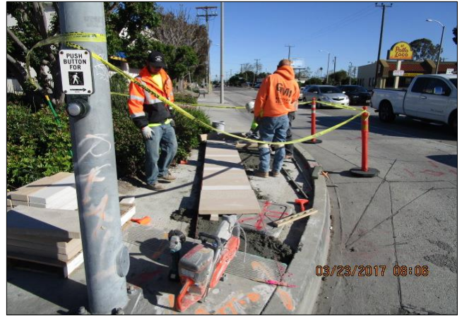
Placing architectural pavers north west corner of Carson/Main.
