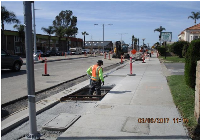
Placing tree well grates on north side west of Main.
