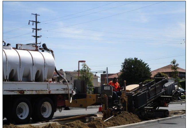
Directional boring for irrigation on Avalon.
