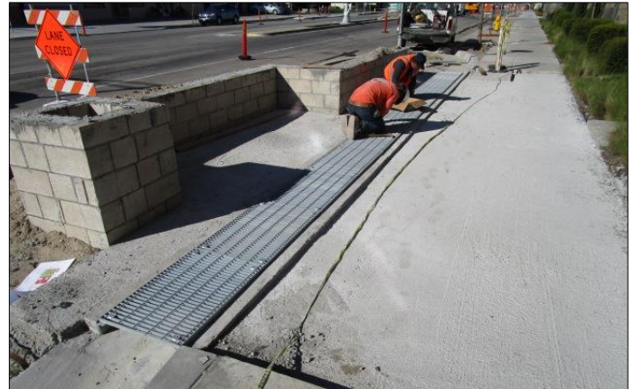
Placing pedestrian culvert grates north side.
