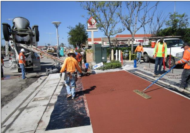
Placing private driveway west of Main.
