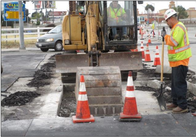
Removing concrete in intersection of Figueroa/Carson.
