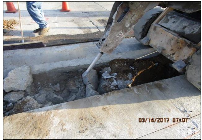
Breaking slurry in trench across Figueroa.
