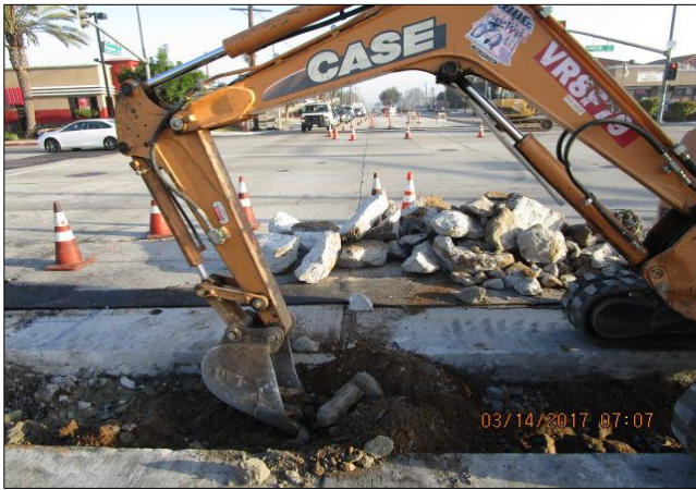
Removing slurry trench across Figueroa.
