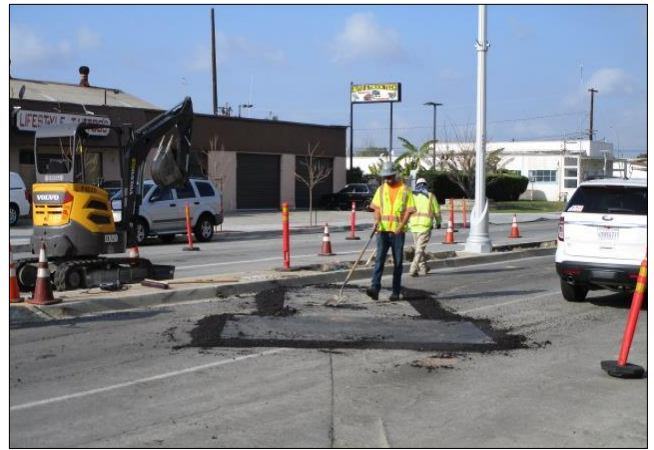
Plating trench to be paved this week.
