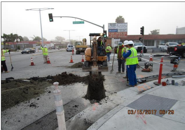
Belco trenching across Dolores for fiber optic.
