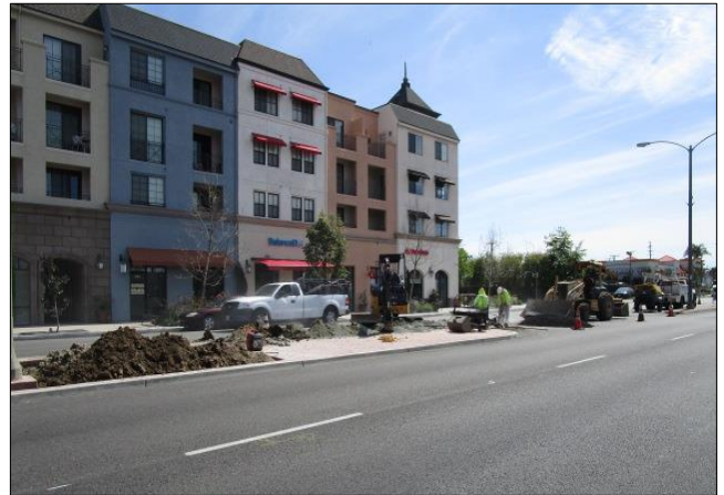
Trenching for irrigation on Avalon south of Carson.
