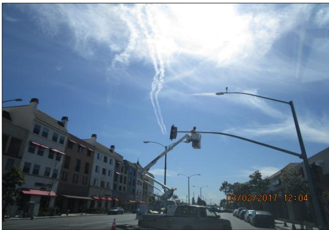
Wiring new traffic signal at Avalon Ralph's.
