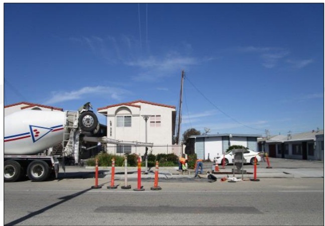
Placing sidewalk on north side west of Moneta.
