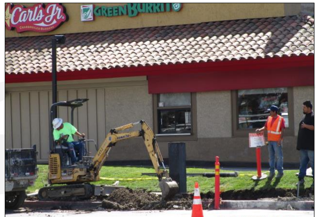
Sidewalk demolition southwest corner of Carson/Avalon.
