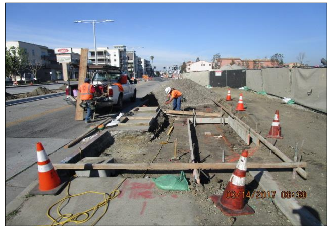
Forming transit station foundation north side west of Avalon.
