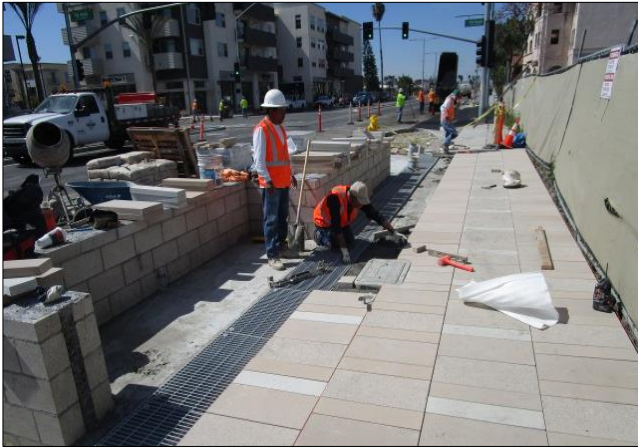
Installing pedestrian culvert grates on north side of Carson.
