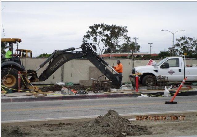
Excavating transit shelter foundation west of Avalon.
