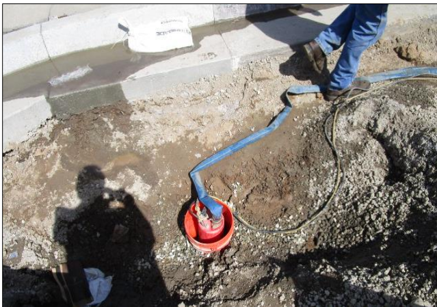
Pumping groundwater between Moneta Ave. and Figueroa St.
