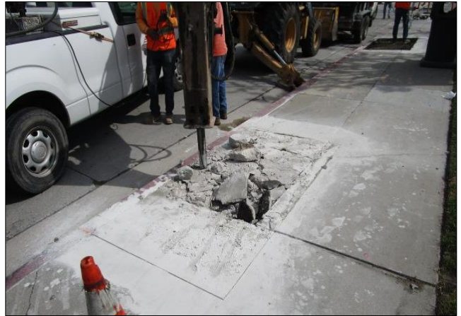
Sidewalk demolition south side west of Avalon.
