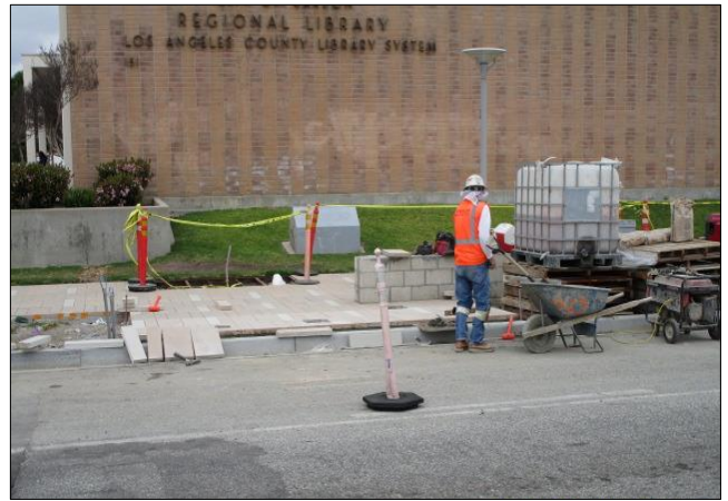
Placing architectural pavers east of Main.
