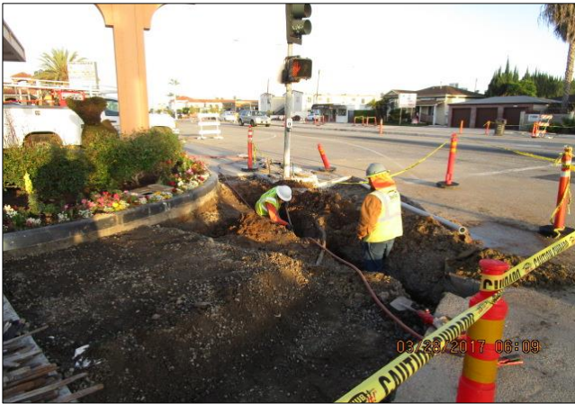
Placing fiber optic conduit southwest corner of Carson/Moneta.
