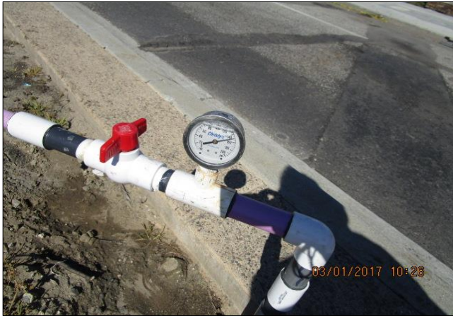
Irrigation pressure test on Carson median.
