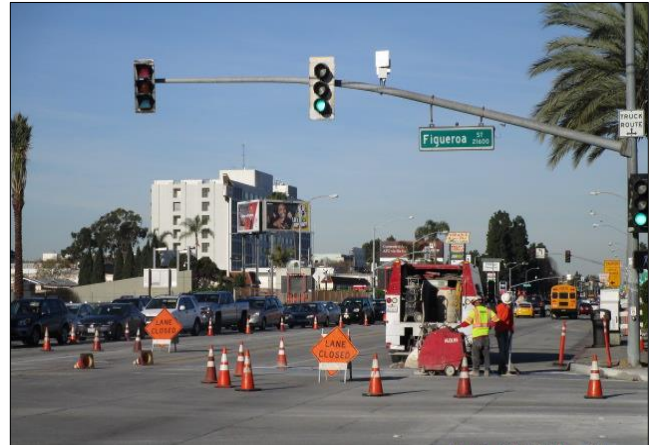
Sawcutting for electrical conduit Carson/Figueroa.
