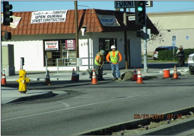
Belco placing slurry over shallow conduit on Grace.
