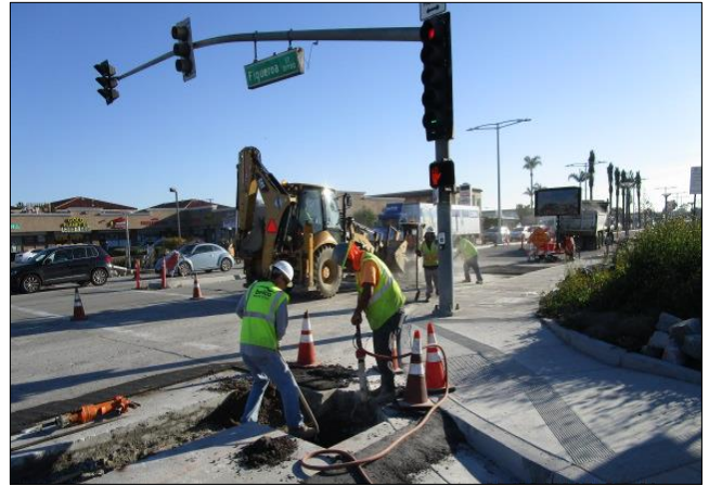
Potholing through slag for trench across Figueroa.
