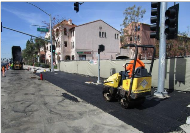
Temporary paving north side of Carson/Via Verde.
