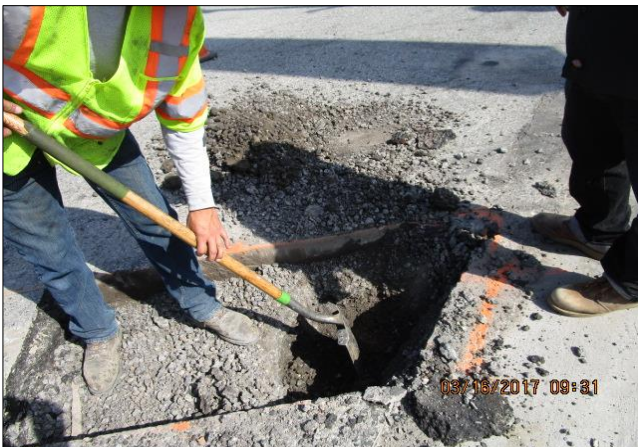
Potholing Moneta to determine thickness of slag.
