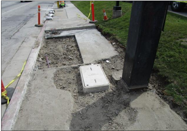
Demolition and forming sidewalk southwest corner of Carson/Avalon.
