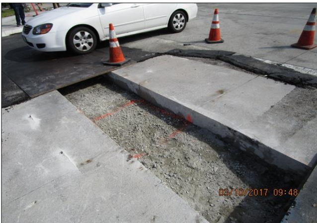
Plates moved for potholing trench across Figueroa.
