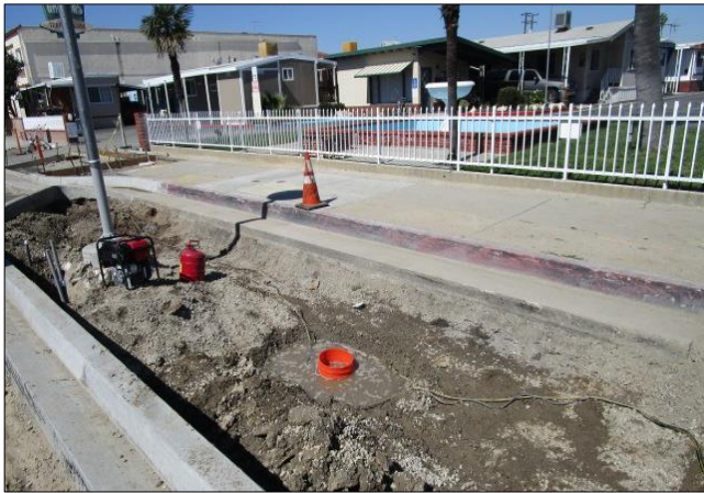
Pumping groundwater at Mobile Home Park.
