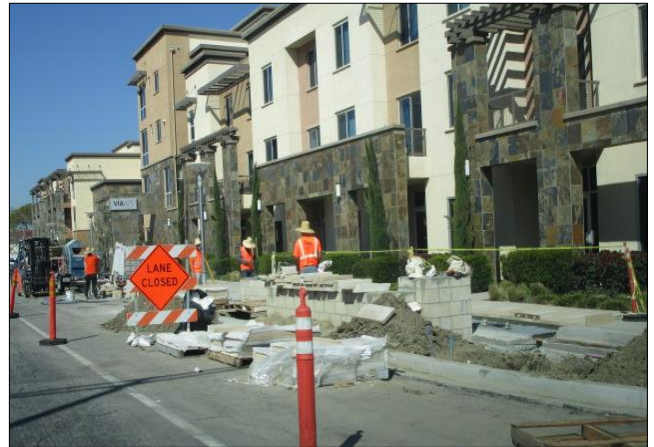
Installing architectural pavers on north side west of Grace.
