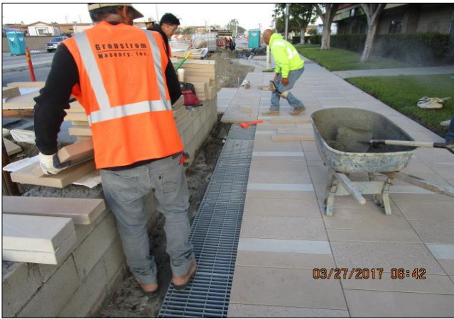
Placing pavers on north side west of Main.
