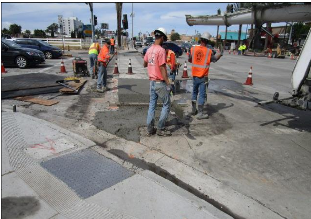
Placing concrete in trench Figueroa/Carson.
