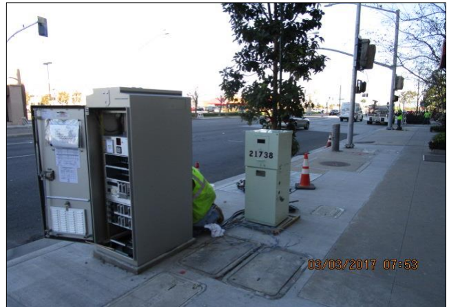
Wiring new traffic signal controller at Avalon Ralph's.
