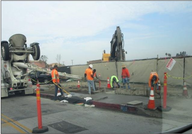
Placing concrete for transit shelter east of Avalon.
