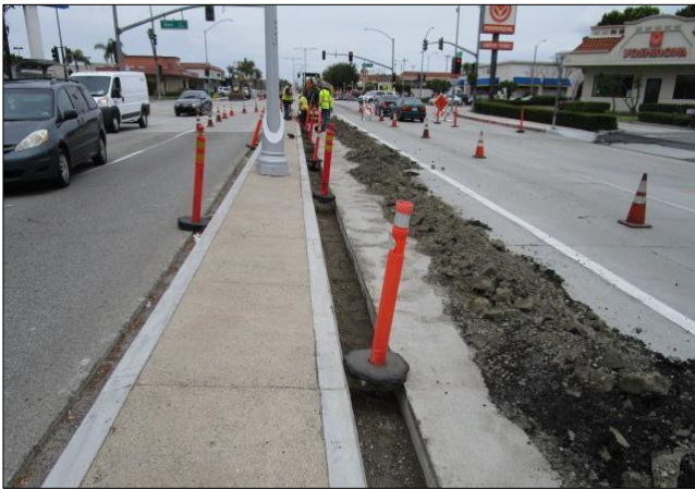
Removing slurry from curb slots on Carson median.
