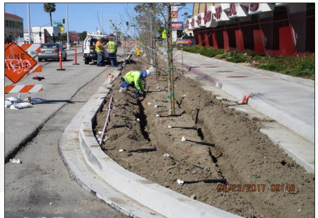
Installing sprinkler heads on north side west of Main.
