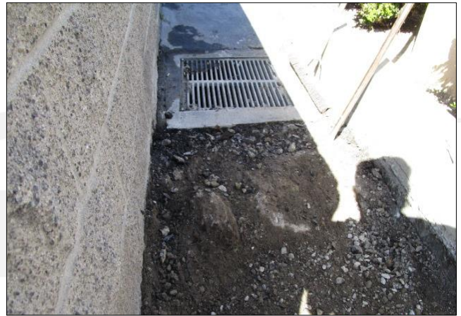
Grading drain for private driveway west of Main.
