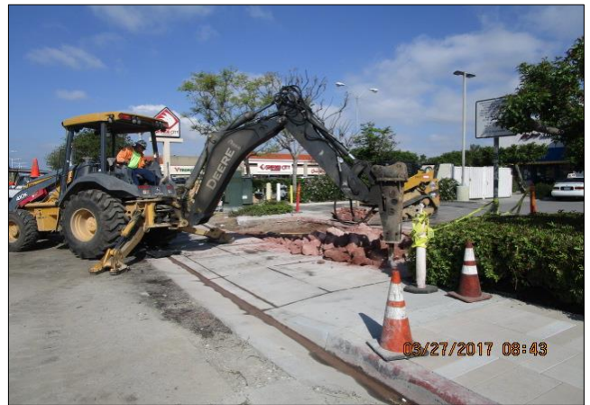
Removing private driveway west of Main.
