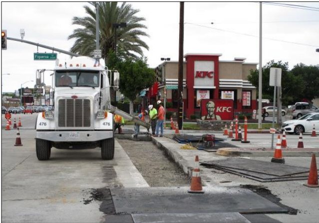
Placing concrete Figueroa/Carson.
