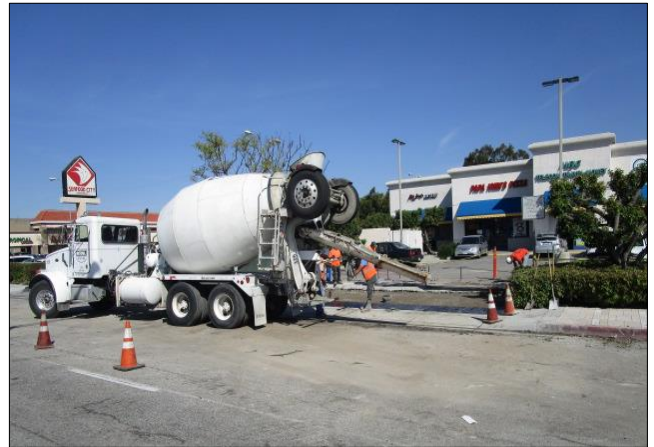
Placing private driveway west of Main.
