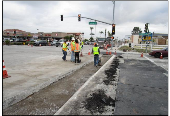
Compacting trench for concrete placement.
