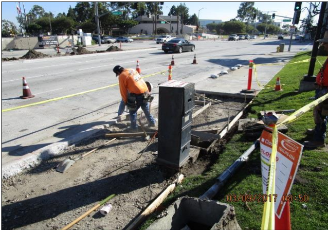
Forming sidewalk southwest corner Carson/Avalon.
