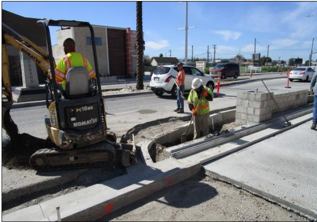
Excavating unsuitable soil on north side east of Figueroa.
