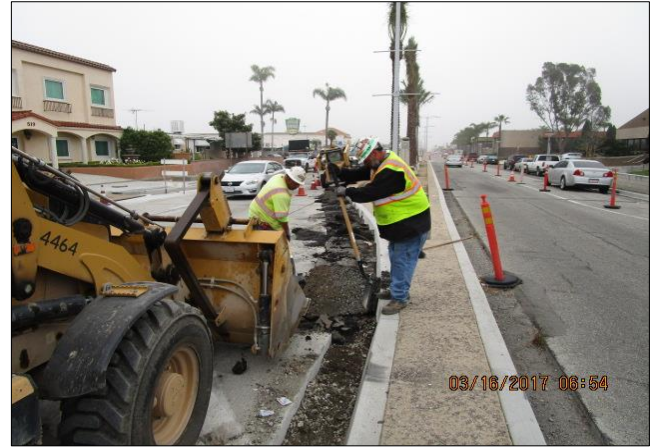
Removing slurry from curb slots on Carson median.
