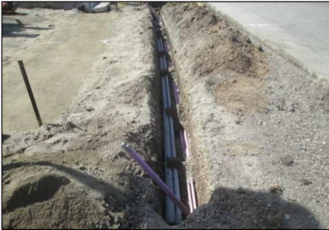
Sharing Trench Electrical and Irrigation
