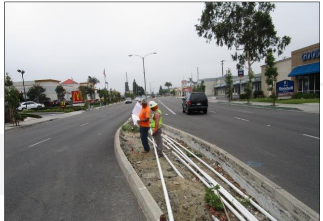
Installing irrigation mainline on Avalon median.
