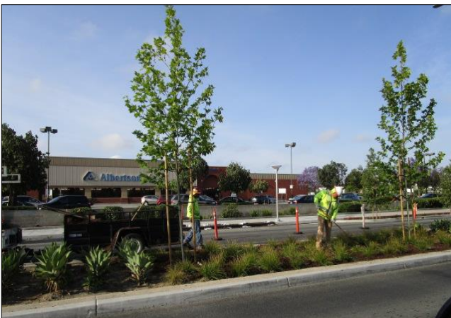
Placing 2" mulch in median east of Main.
