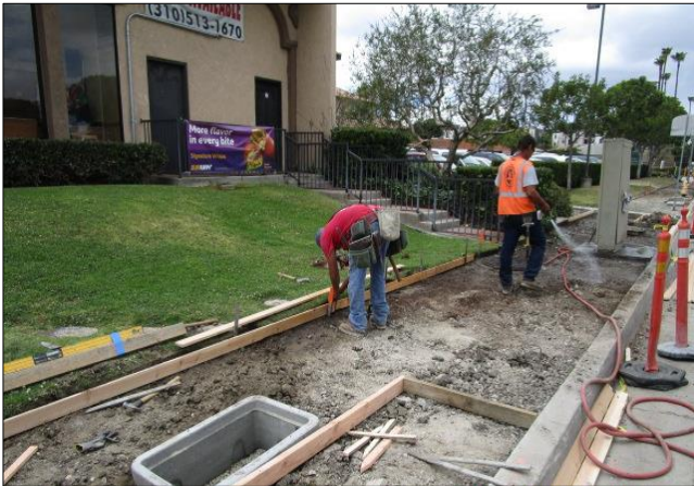
Forming sidewalk and tree wells south side east of Avalon.
