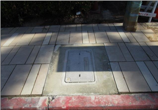
Pull box replace by SCE west Figueroa.
