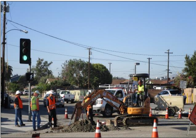
Excavating fiber optic trench across Moneta.
