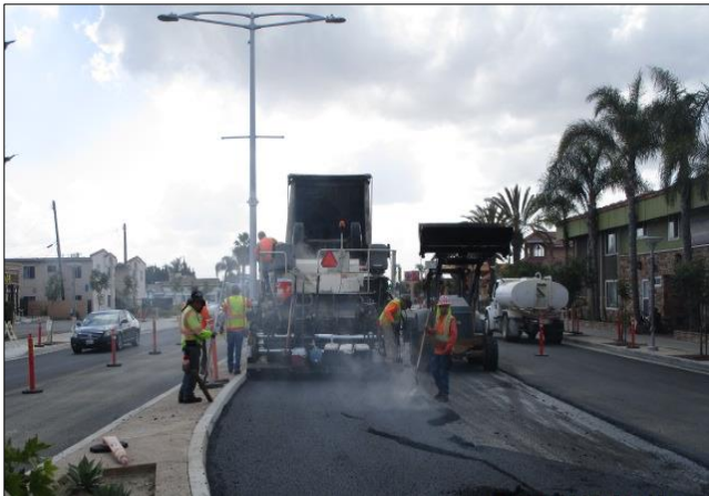
Paving Carson St. between Main and Figueroa.
