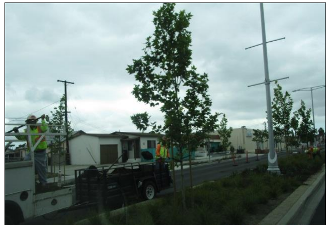
Placing 2" mulch on median islands.
