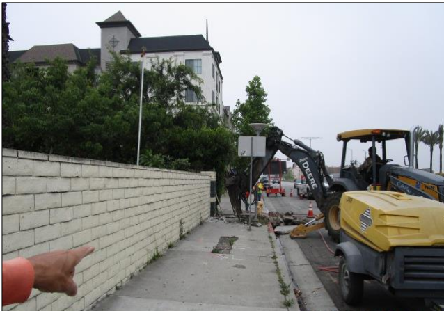
Removing sidewalk south side east of Avalon.
