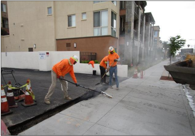
Placing asphalt in forming slots behind driveways.
