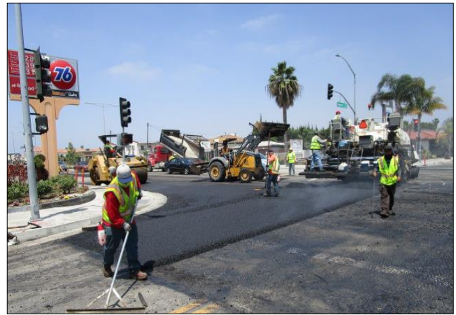
Paving intersection of Carson and Moneta.
