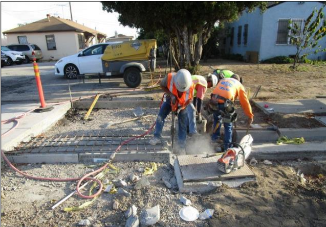
Altering drainage culvert to avoid SCE vault.
