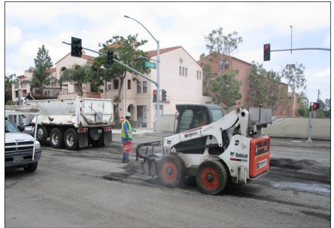
Small grinder trimming around valves and manholes.
