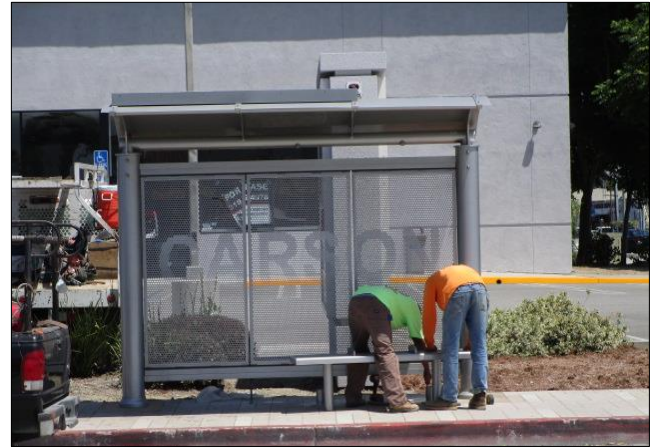
Installing bench in transit shelter west of Main.
