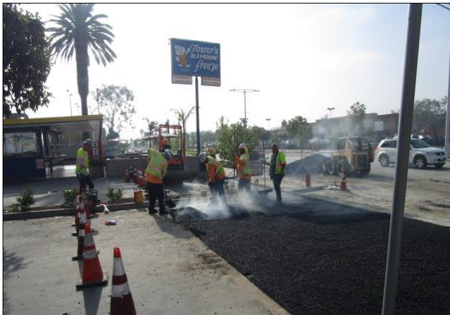
Placing asphalt concrete in private property driveway.
