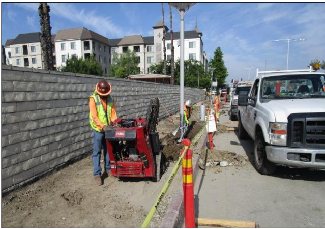
Trenching for irrigation south side east of Avalon.
