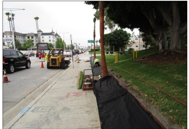
Placing fabric for decomposed concrete north side east of Avalon.
