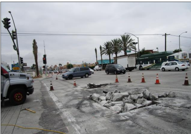
Pothole repair Figueroa intersection.
