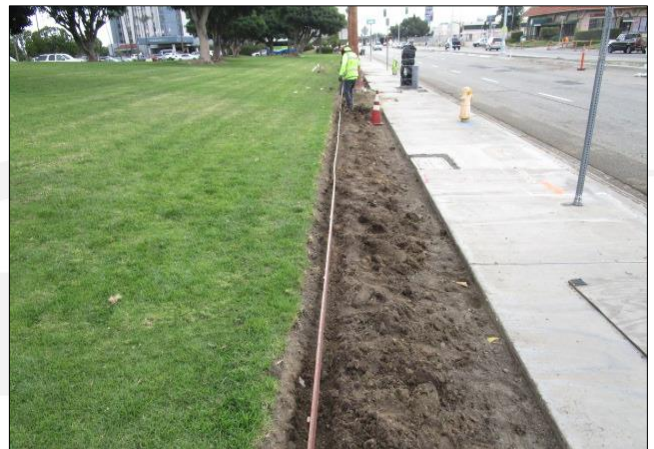
Installing header board for decomposed concrete east of Avalon.
