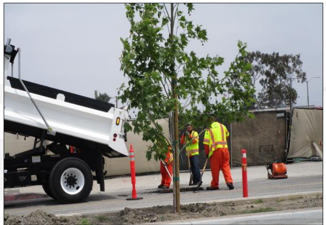
City crew patching recycled water potholes.
