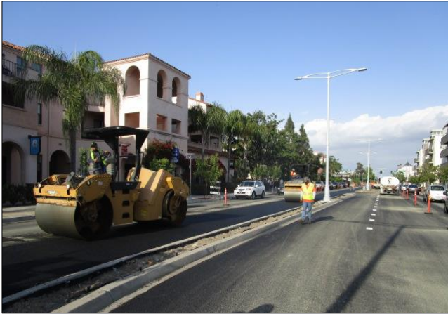
Compacting asphalt.
