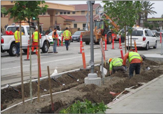
Installing irrigation laterals west of Main.
