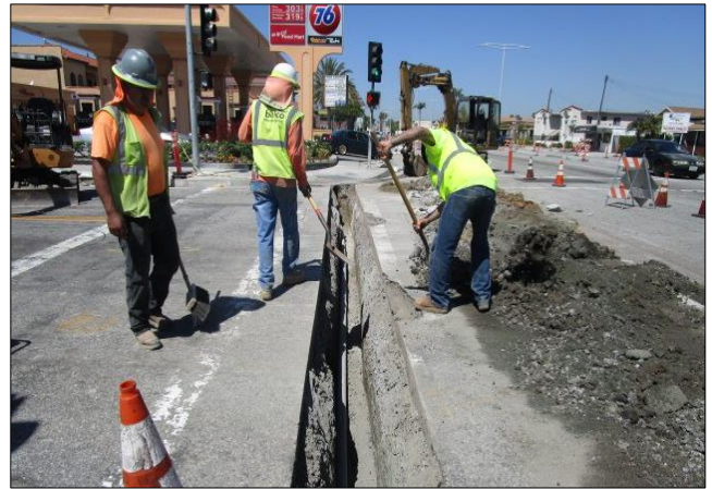
3" conduit placed across Moneta for fiber optic.
