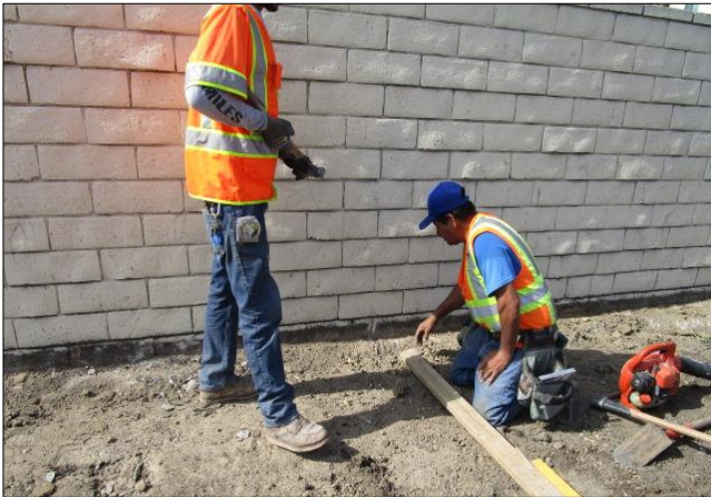
Grading for new sidewalk south side east of Avalon.
