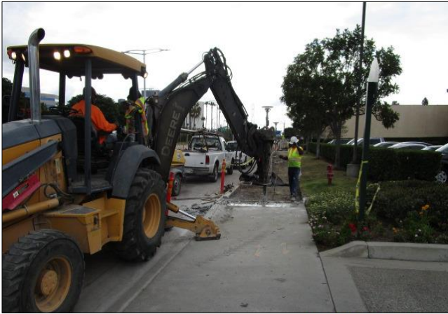
Removing sidewalk on south side east of Avalon.
