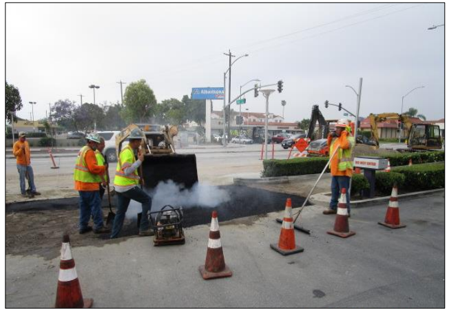
Placing asphalt concrete for driveway east of Main.
