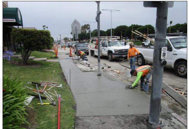
Finishing concrete on south side at Bonita.
