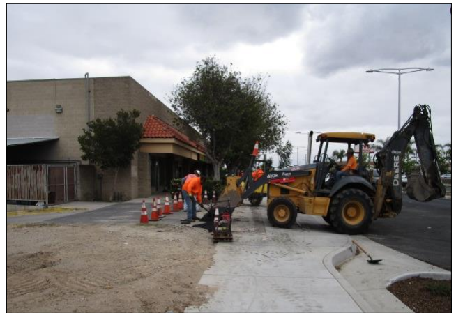
Paving driveway forming slots west of Main.
