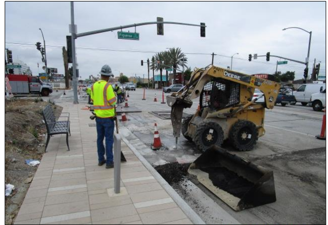
Breaking concrete for pothole repair.
