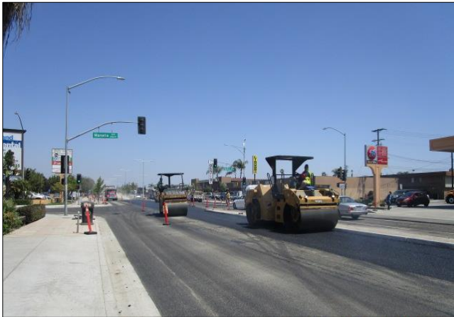
Compacting asphalt.
