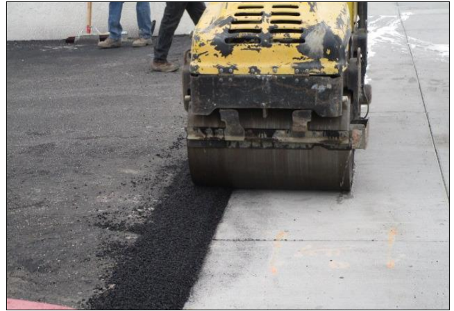
Compacting asphalt in forming slots.
