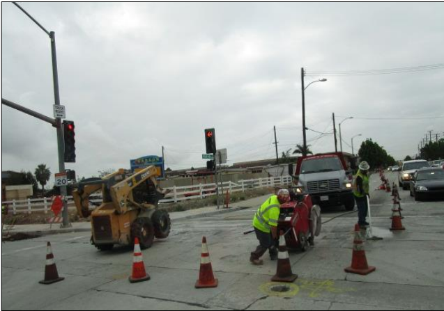
Sawcutting for pothole repair Figueroa intersection.
