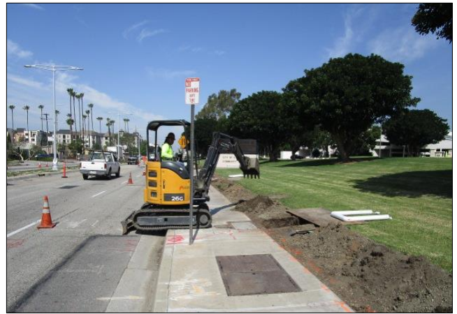
Excavating for palm trees in front of Civic Center.
