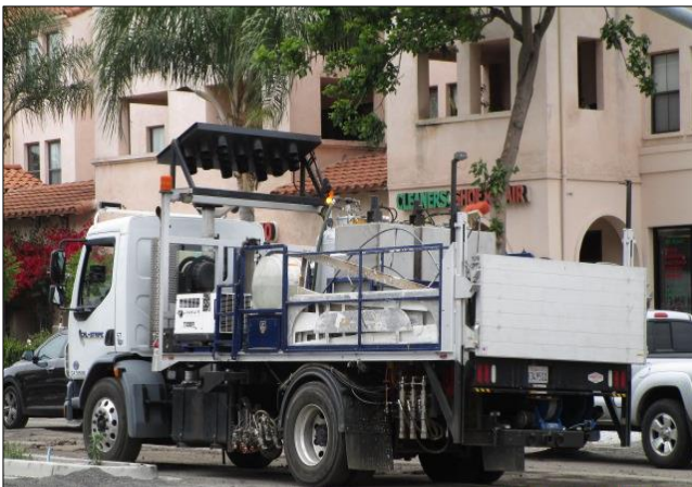
Cal Stripe applying temporary striping.
