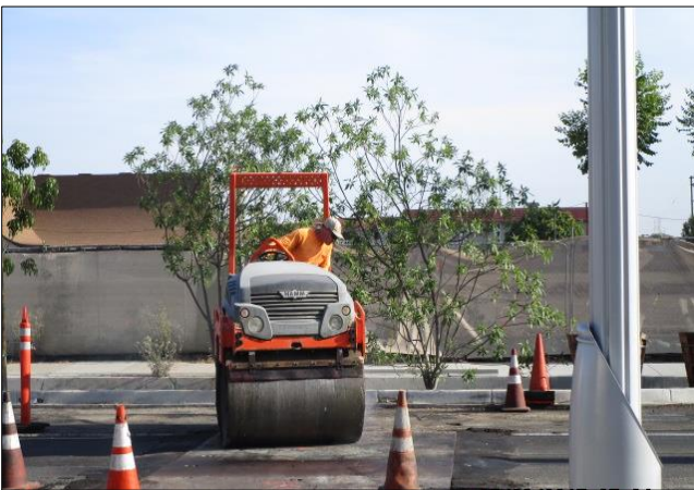
Restoring irrigation trench crossing Carson.
