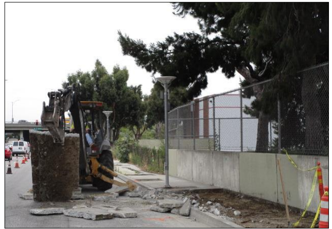
Removing concrete on south side of Carson east of Bonita.
