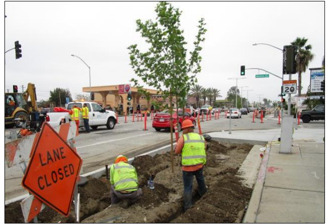
Installing irrigation west of Main.
