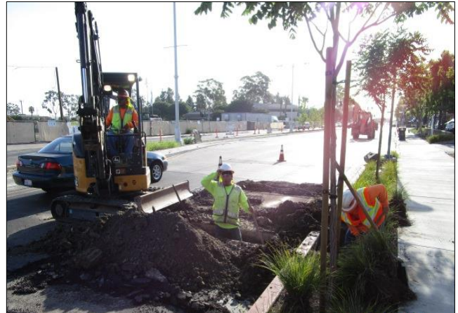
Excavating irrigation crossing east of Via Verde.
