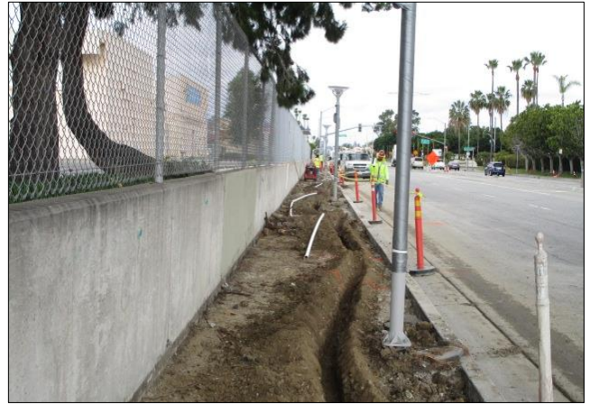
Trenching for irrigation south side east of Bonita.
