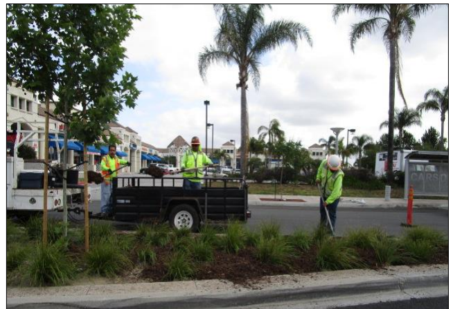
Placing mulch on median islands.
