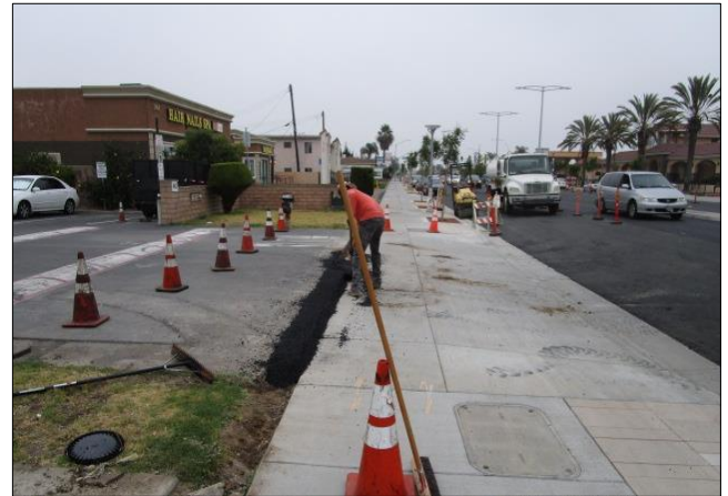
Paving forming slots on driveways west of Moneta.
