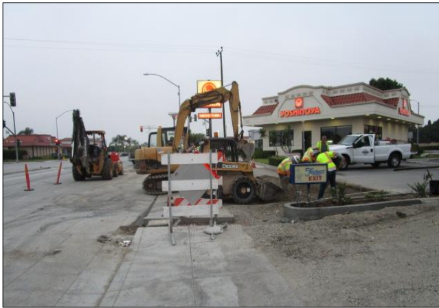
Grading private driveway east of Main.
