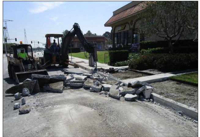
Removing sidewalk east of Avalon on south side.
