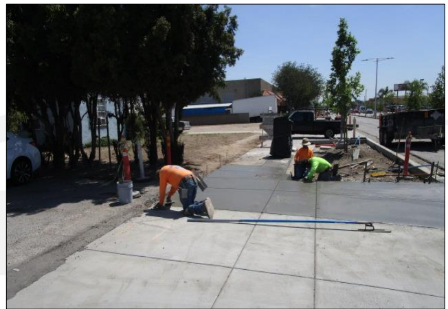
Finishing driveway north side west of Main.
