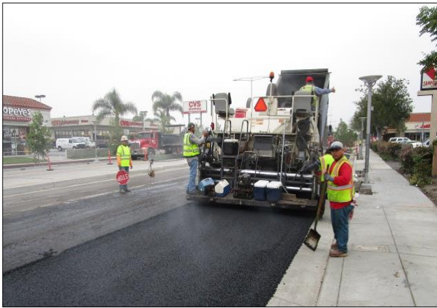
Paving Carson St. between Main and Figueroa.
