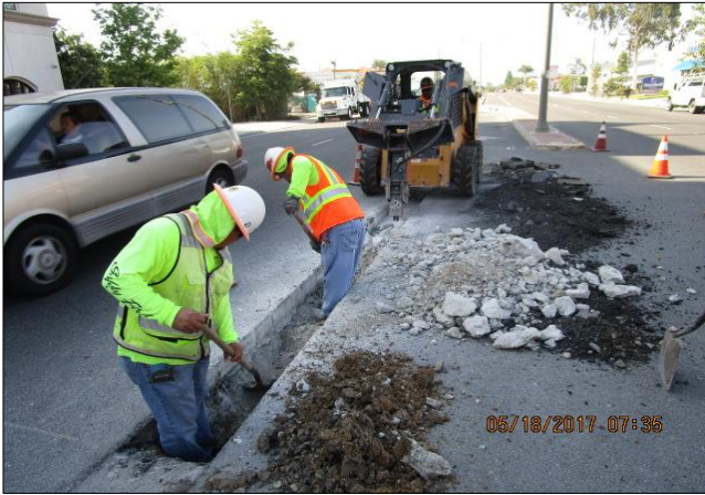
Trenching for irrigation on Avalon.
