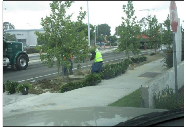
Planting five gallon plants on south side of Carson St.
