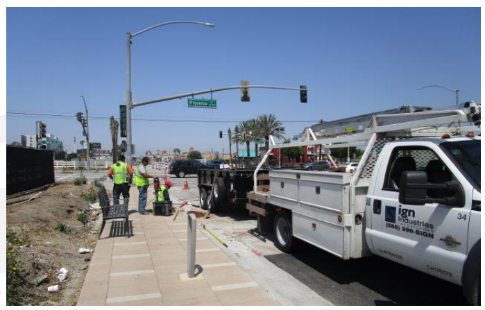
Excavating for wayfinding sign foundations.
