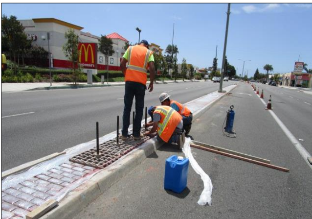
Placing red stamped concrete on Avalon media.
