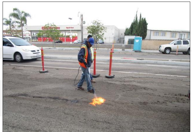
Burning edges of petromat following coldmill.
