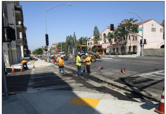
Permanent resurfacing of trench across Via Verde.
