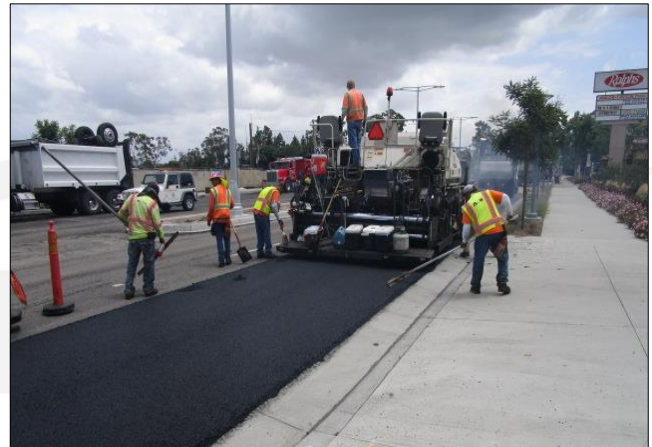
Paving eastbound Carson west of Avalon.
