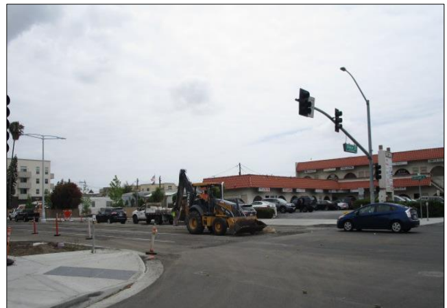
Trimming gutter edges following coldmill.
