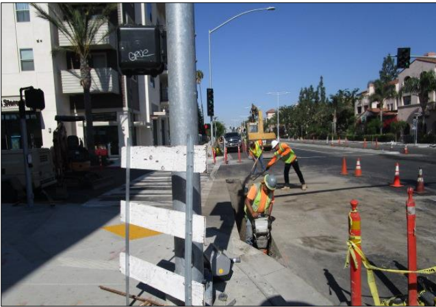
Restoring electrical trench across Via Verde.
