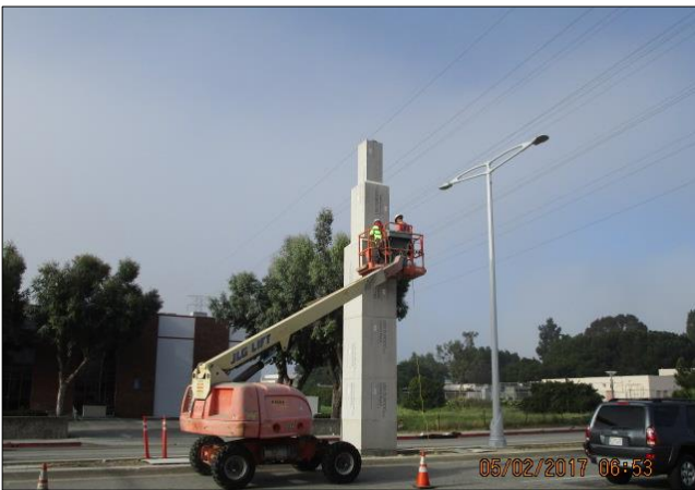
Installing backer board on monument.
