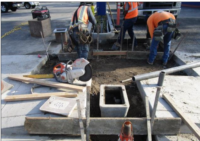
Installing parkway culvert north side east of Main.
