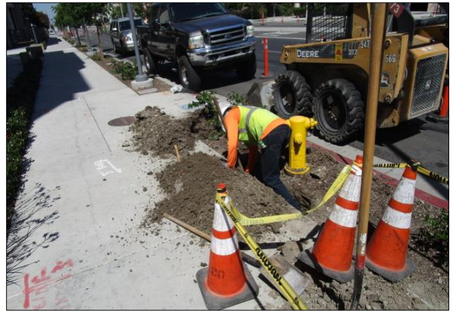
Installing electrical conduit under curb ramp.
