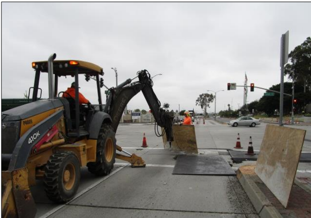
Trenching across south side for fiber optic.
