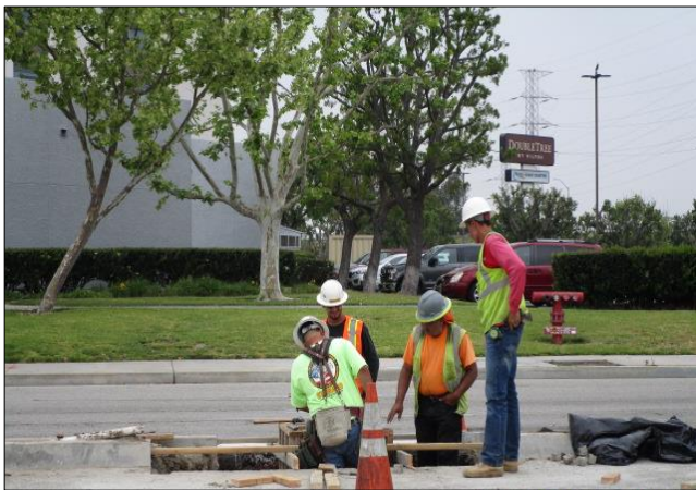
Forming and placing streetlight foundation east of Avalon.
