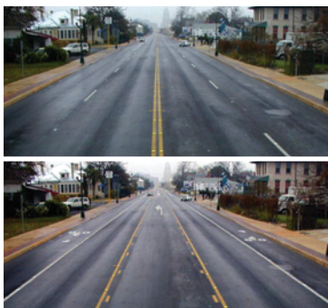
Road diet used to achieve bike lanes in Albuquerque, NM. Top: before. Bottom: after.
