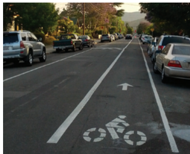
FIGURE 10.7 Bike lane striping and stencil.
