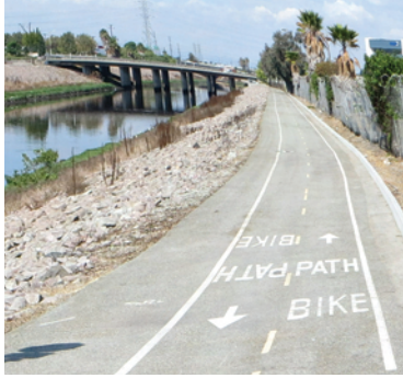
Dominguez Channel bicycle path in Carson.
