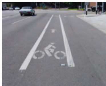
FIGURE 10.7 Bike lane striping and stencil.
