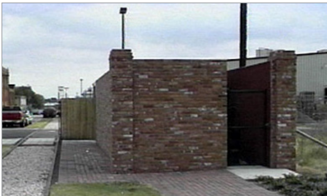
Site utility enclosure
