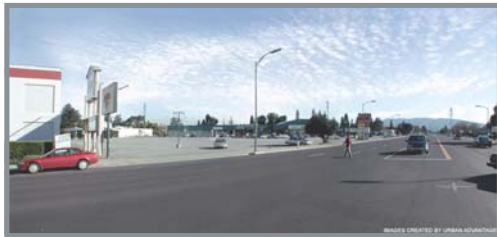
TYPICAL EXISTING CONDITION ALONG THE STREET
