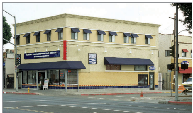
Facade after improvements
