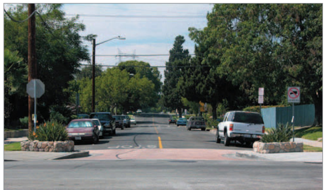
Landscaping in a side street curb extension creates a neighborhood gateway.
