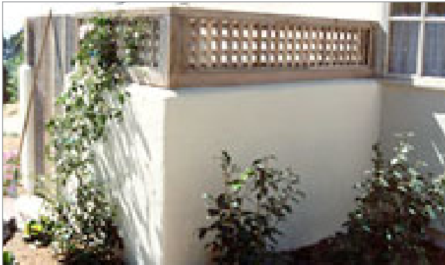
Trash enclosure wall and trellis
