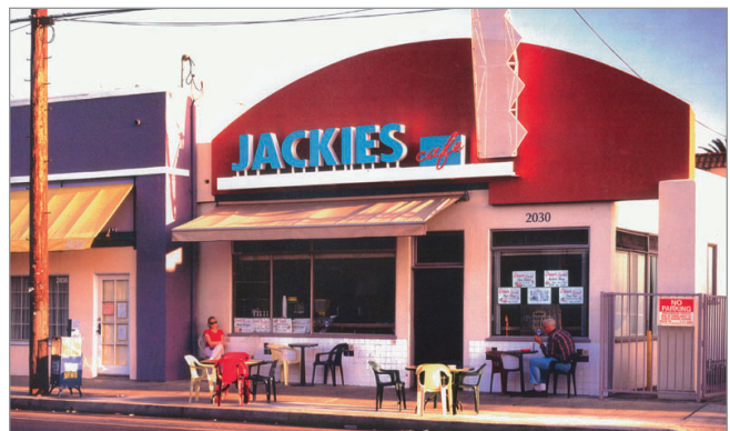
Facade after improvements
