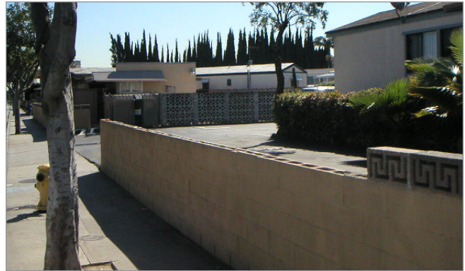
Existing block wall at mobile home park
