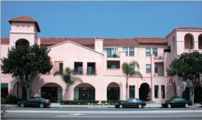
Typical existing conditions
