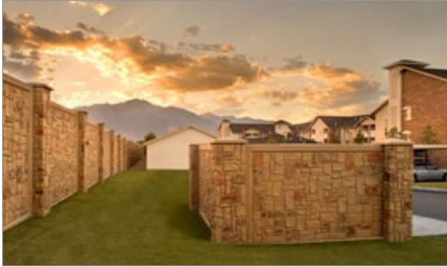
Trash enclosure screen wall
