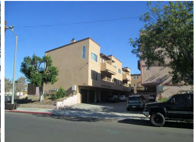
18. Eastern adjacent S Perry Street and residential properties.
