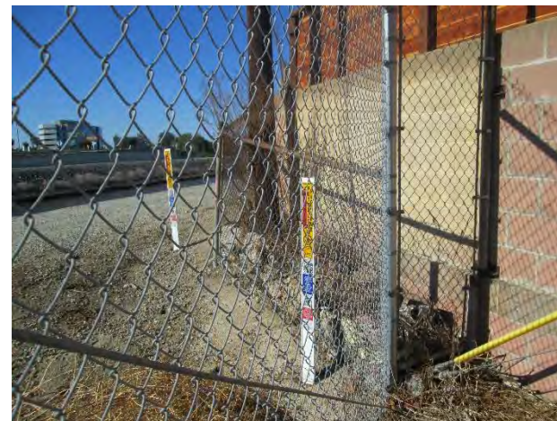
12. Underground pipeline indicator at northwest corner of the Site.
