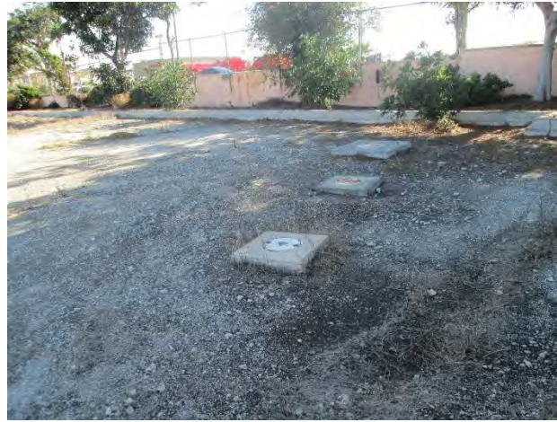
14. Typical groundwater monitoring wells.
