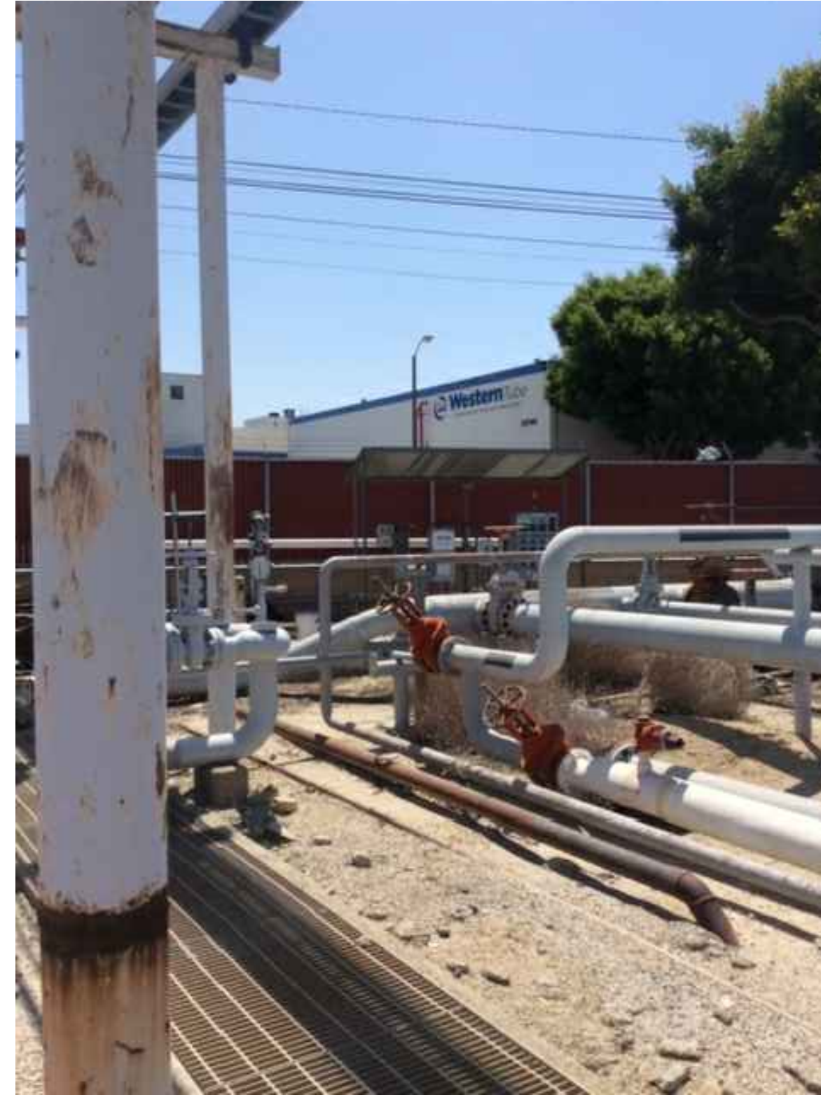
2 EASTERN TERMINUS OF EXISTING PIPE RACK NEAR WILMINGTON AVENUE, VIEW EAST
