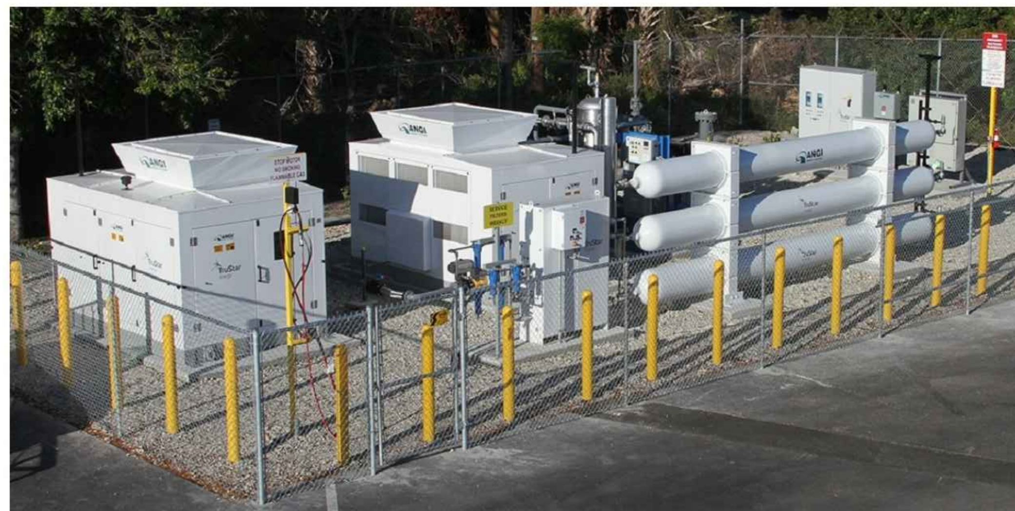
TYPICAL CNG SYSTEM COMPOUND, 2 COMPRESSORS AND 3 TANKS
