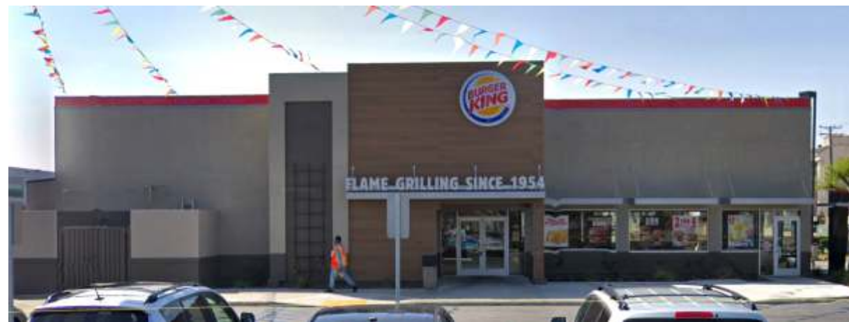
H 02 SINGLE FACE ILLUMINATED PAD TENANT I.D. - Typical South Elevation 20950 Figueroa St.
