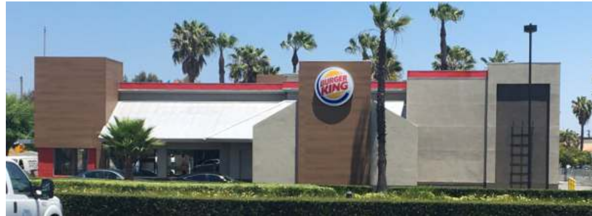
H 01 SINGLE FACE ILLUMINATED PAD TENANT I.D. - Typical North Elevation 20950 Figueroa St.
