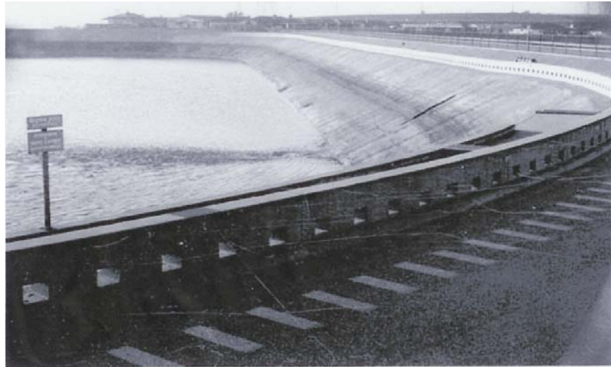
Baldwin Hills Dam - Dark spot in upper right hand quadrant shows the beginning of the break in the dam.
