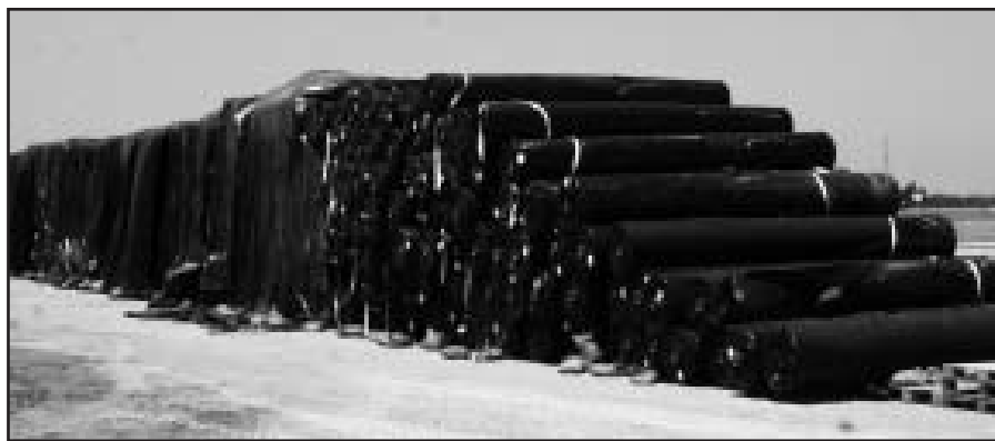
Rolls of geomembrane liner at the ready
