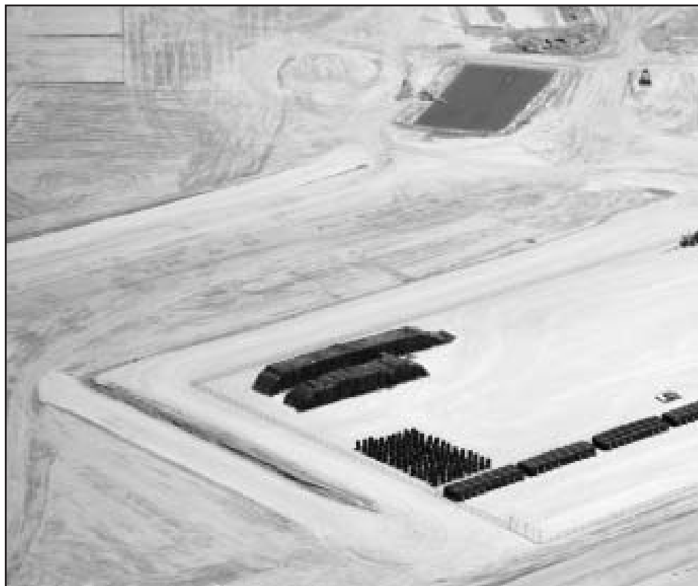
Helicopter view of liner and pipe being stored on the site
