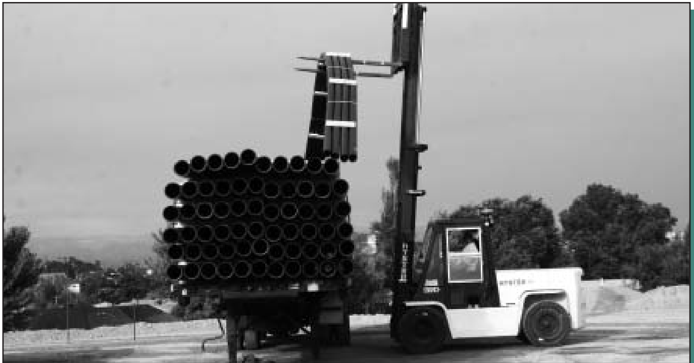
A forklift unloading polyethylene pipe for the landfill gas system
