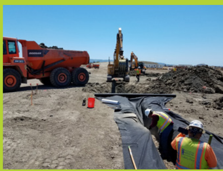
Installation of GCCS System
