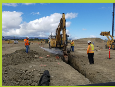
Installation of Horizontal Collector
