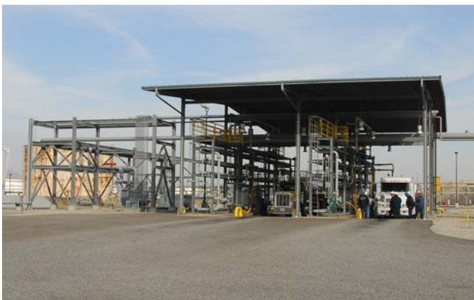
Ethanol and petroleum products loading racks.
