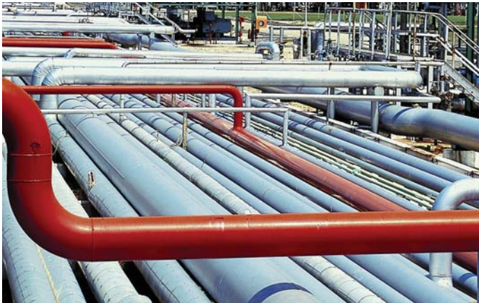
Ethanol is transferred by pipeline to storage tanks.
