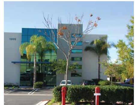
Examples of variation in vertical planes of the building include change in material, depth, and texture, as well as the use of canopies.
