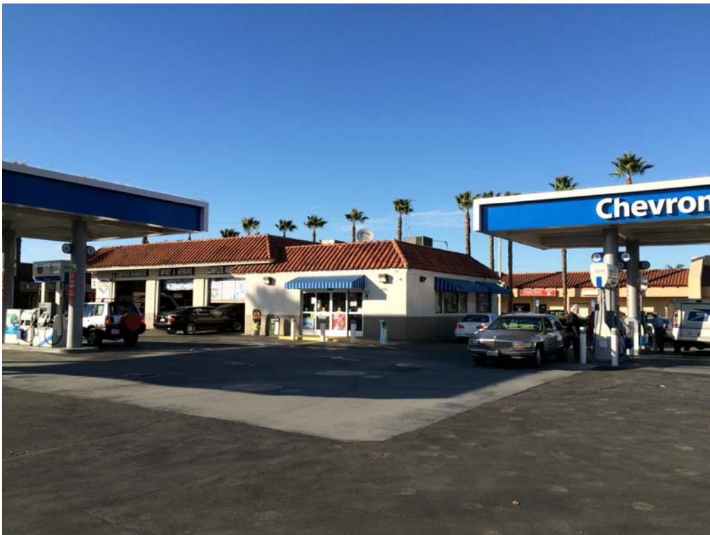
View of the Chevron station and automotive repair facility 21609-21635 Avalon Blvd. & 645-655 E Carson St.
