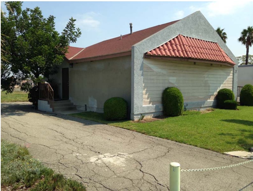
View of the front (south) of the subject property (looking NE) 625 E Carson St, Carson
