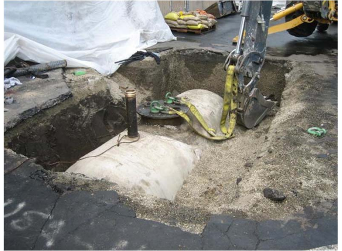
UST pre-rigged and pre-lifted prior to UST removal.
