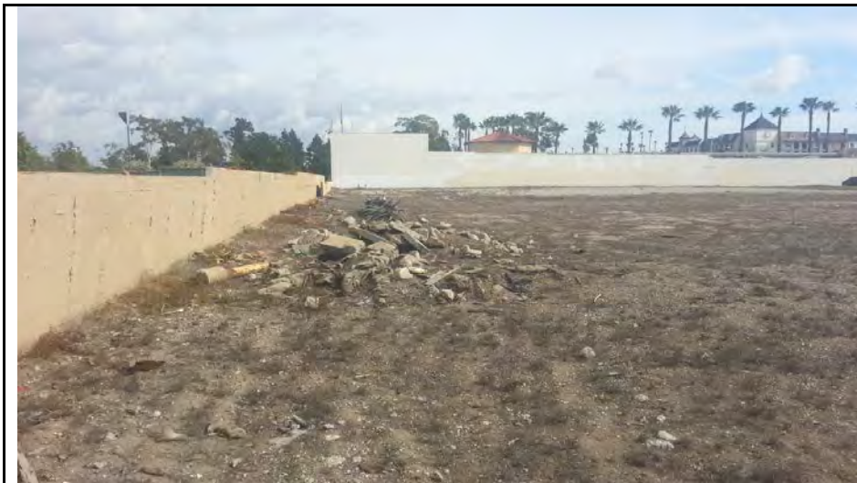
Photo No. 9: View of construction debris along northern border of 615 E. Carson Street parcel.
