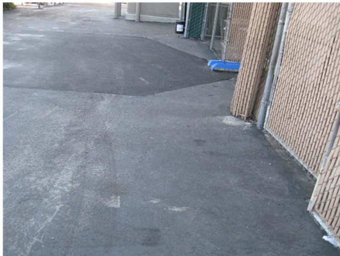
Used oil cavity final grade.
