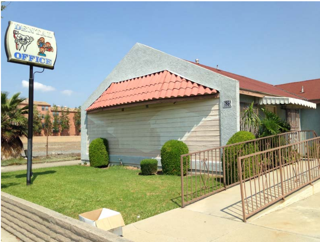
View of the front (south) of the subject property (looking NW) 625 E Carson St, Carson
