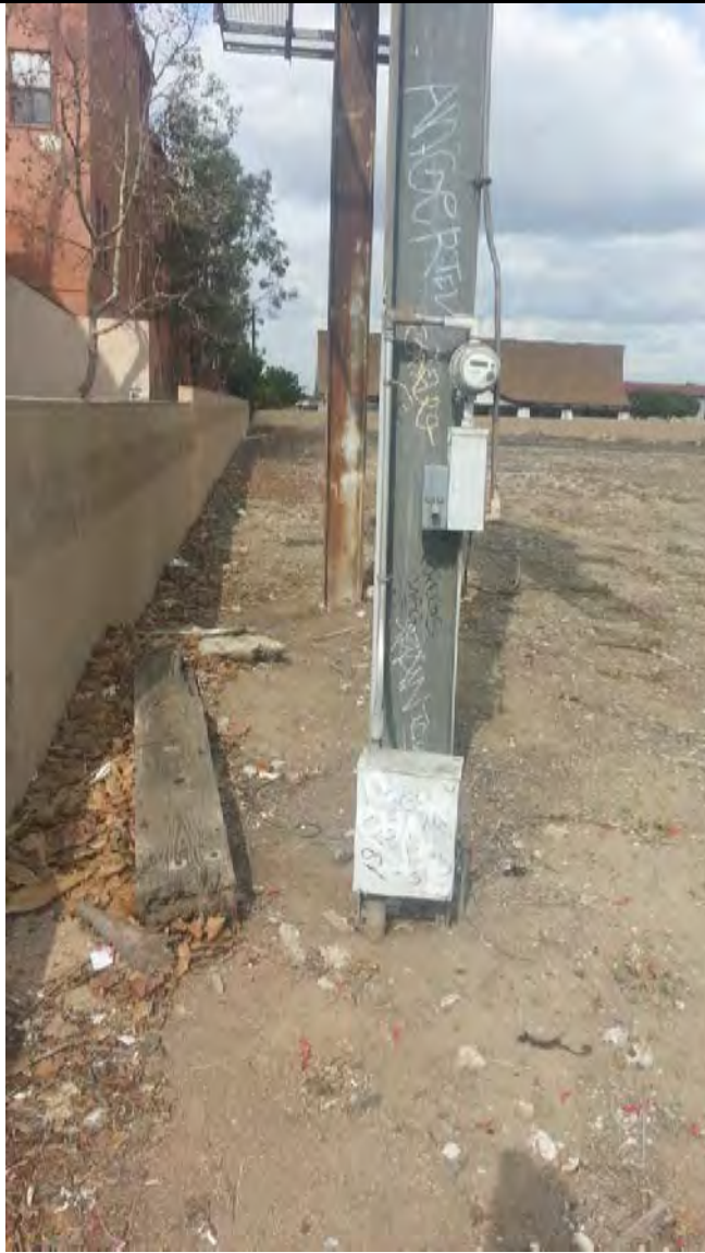
Photo No. 5: View of electrical equipment at base of billboard on southwest corner of 615 E. Carson Street parcel. Note trash and debris along western border of Site.
