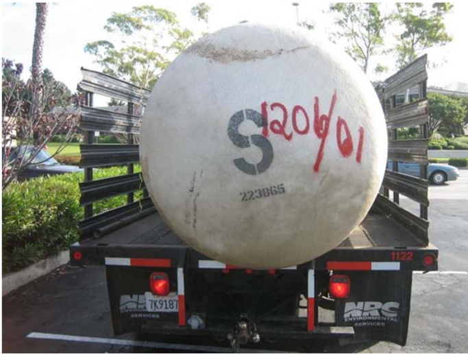
UST stenciled and numbered with CIH number prior to transportation to approved landfill.
