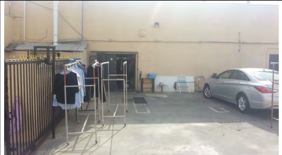
Photo No. 20: View of rear of Happy Cleaners facility from over south wall of 21521 S. Avalon Boulevard parcel. Note emission stack in left of photo.
