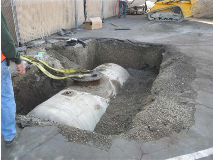
UST exposed in preparation for 2 nd triple rinse and degas.
