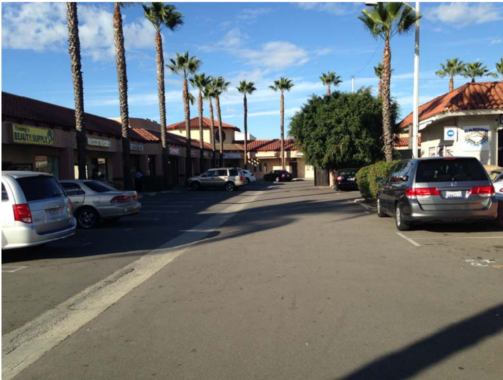
West side of the L-shaped strip center building, looking N 21609-21635 Avalon Blvd. & 645-655 E Carson St.
