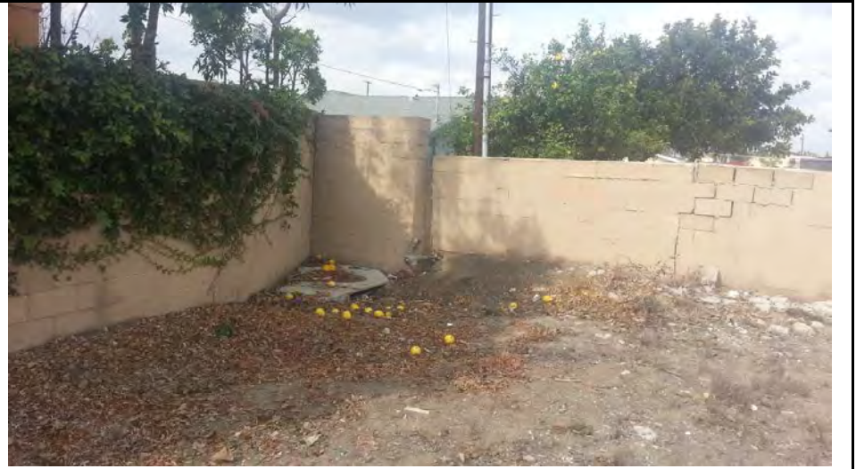
Photo No. 8: View of storm drain at northwest corner of 615 E. Carson Street parcel
