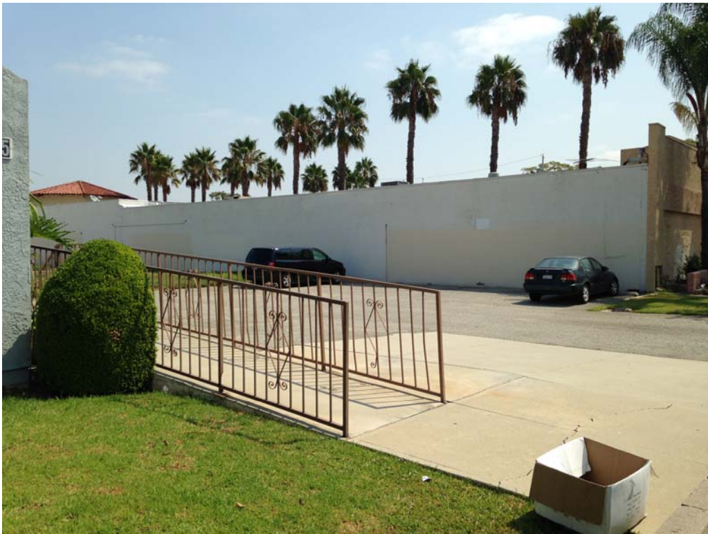
View of the subject property parking area (looking E) 625 E Carson St, Carson
