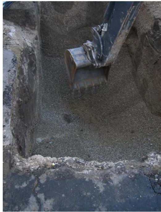
Tank cavity post tank pull.
