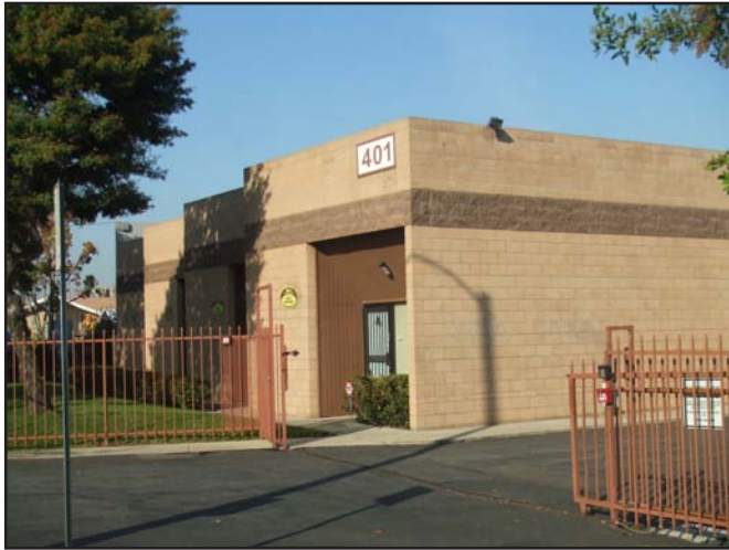
View 7: Industrial Building on Gardena Boulevard, Adjacent to Mobile Home Park.
