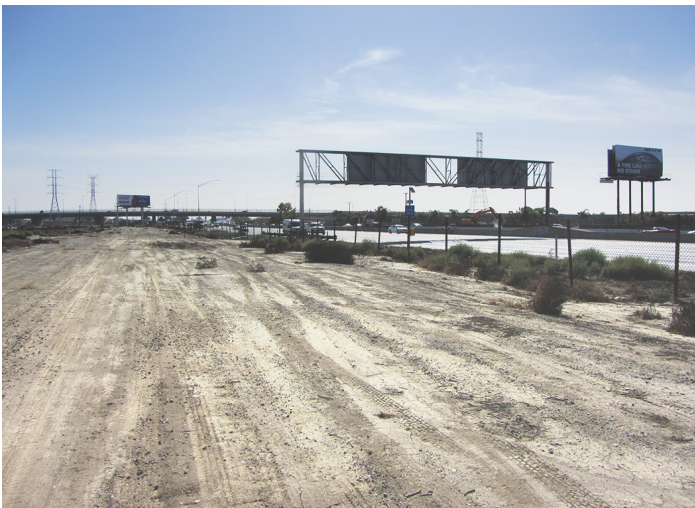
Southeastern view of the I-405 freeway and Existing Sign Numbers 3070 and 3071.
