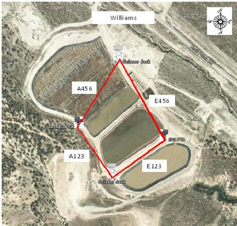
Figure 2-1. Williams Rulison Facility
