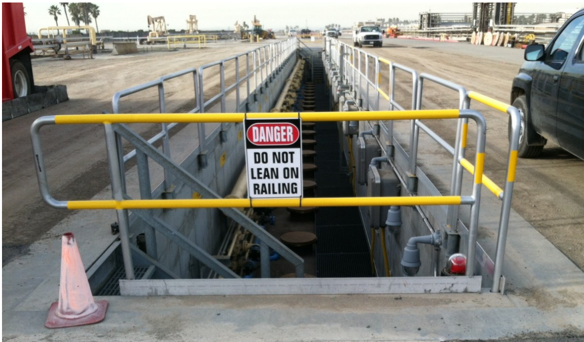
Photo 2.6-1 Typical Below-Grade Well Cellar
