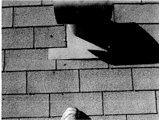
Metal flashing on the front house. In good condition.
