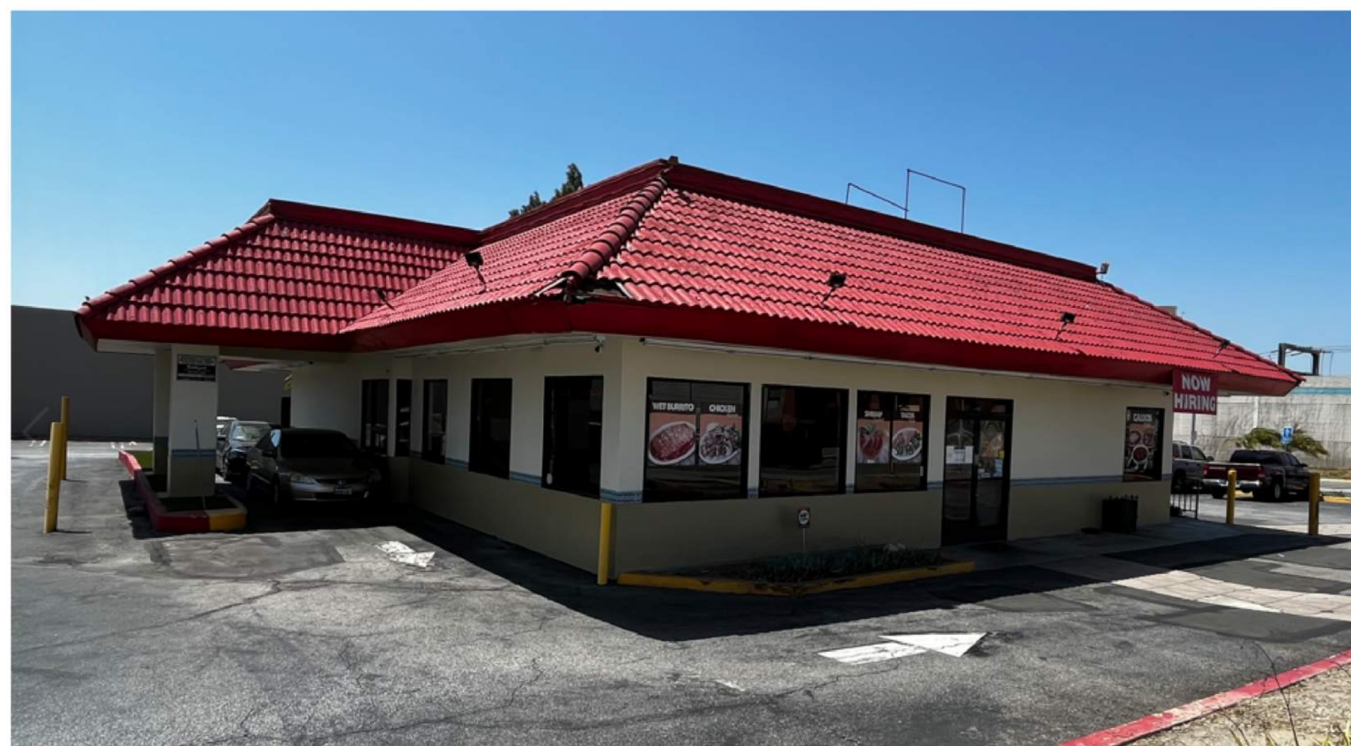
3 SITE PHOTO - VIEW FROM SOUTHEAST CORNER Scale : N.T.S.
