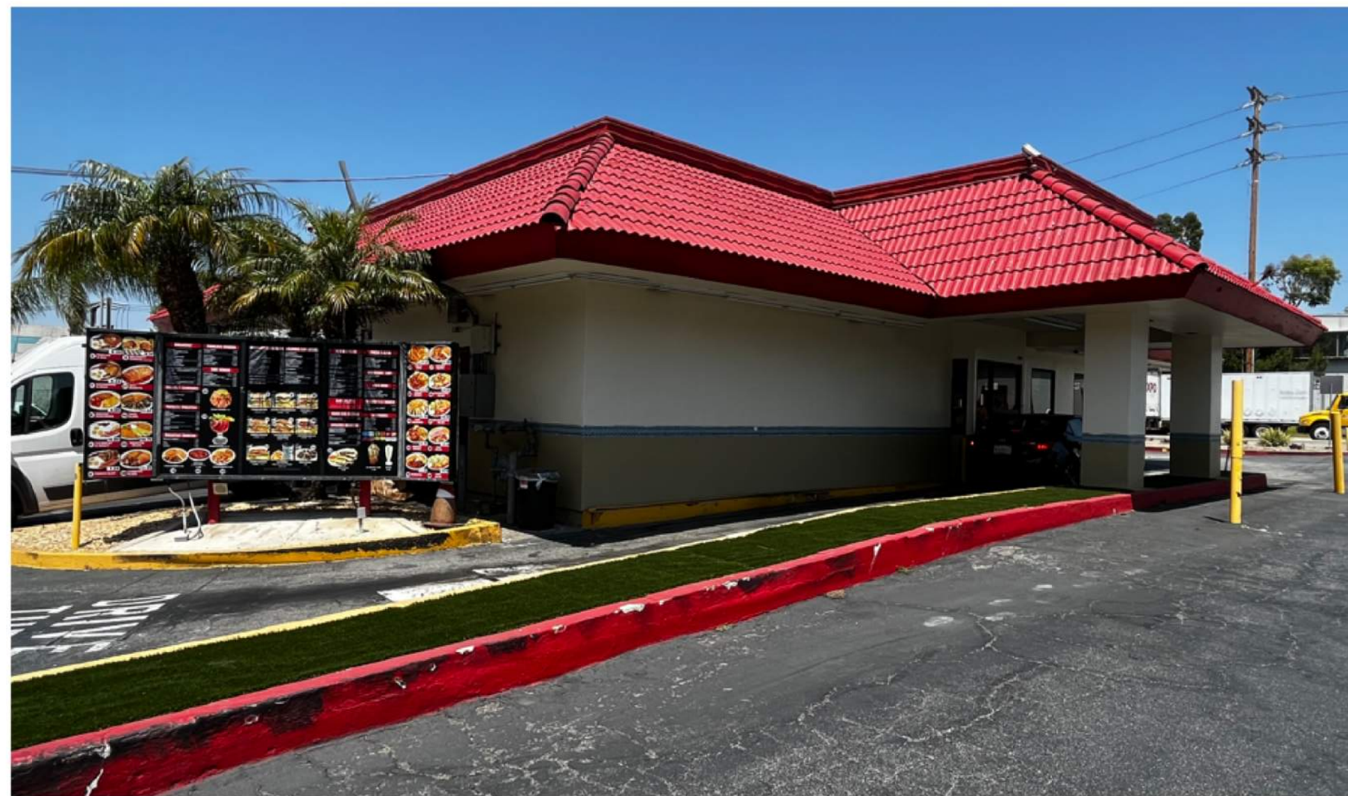
4 SITE PHOTO - VIEW FROM SOUTHWEST CORNER Scale : N.T.S.
