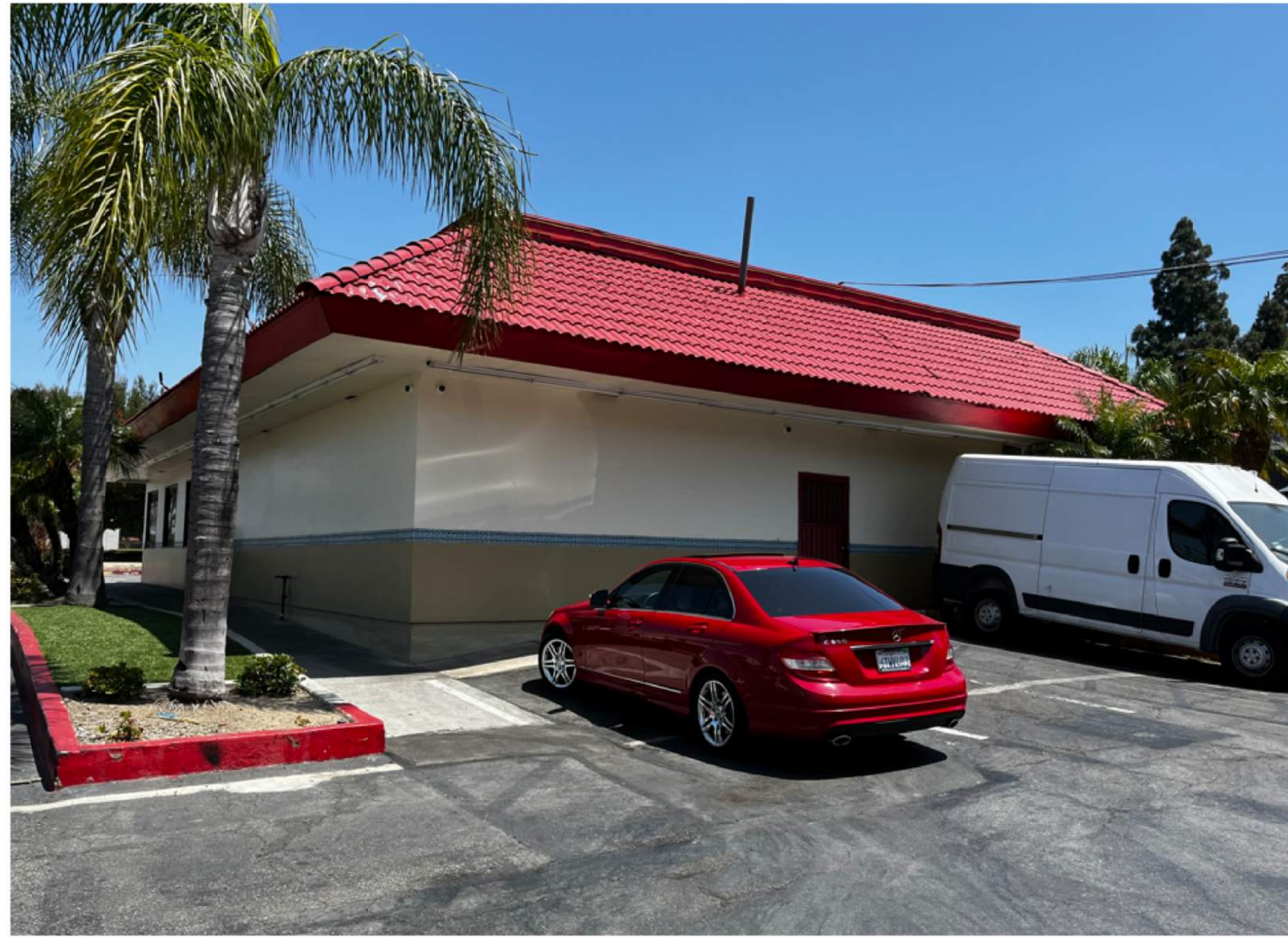
5 SITE PHOTO - VIEW FROM NORTHWEST CORNER Scale : N.T.S.
