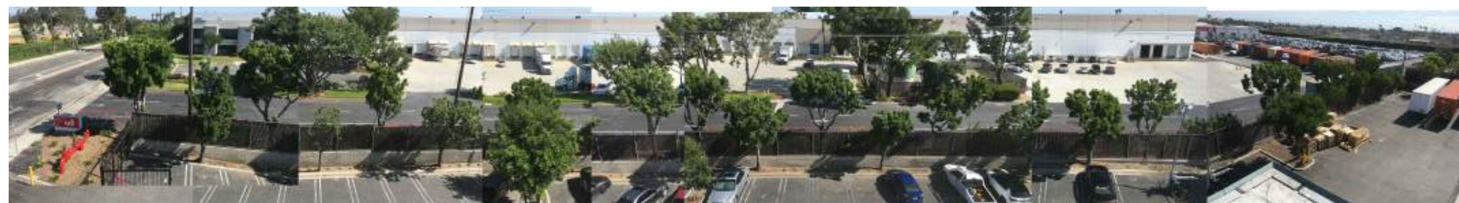
G. NORTH ROOF VIEW
