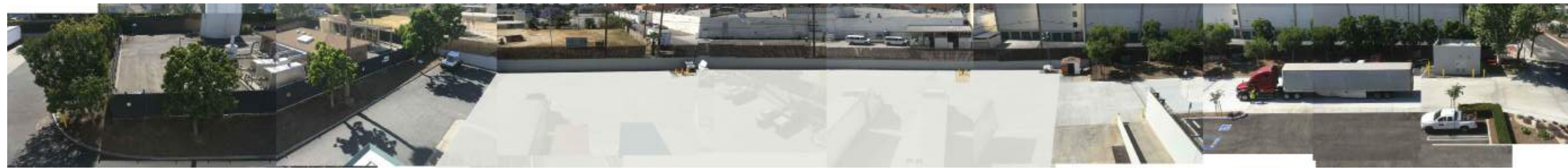
E. SOUTH ROOF VIEW
