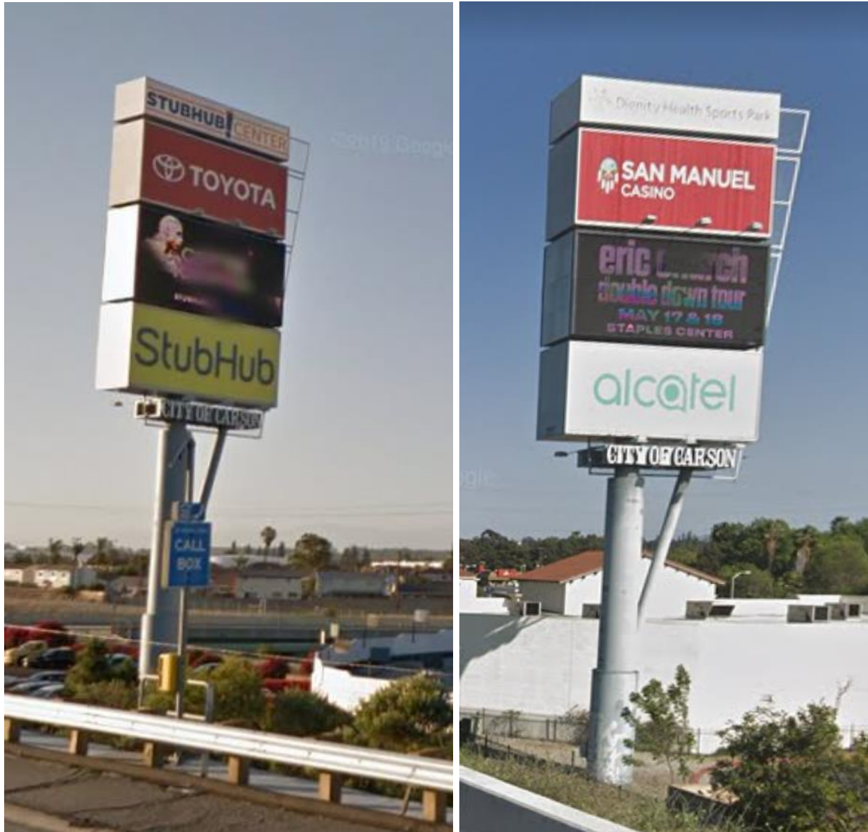
Figure 3: Existing I-405 sign (Left) Existing SR-91 sign (Right)
