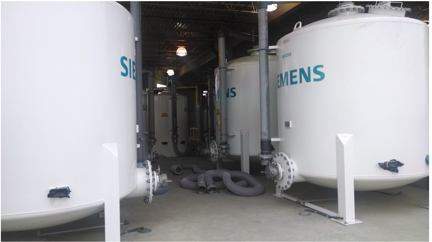
Above: Another view of the GAC tanks for vapor/air treatment to remove contaminants from the sparged process water.
