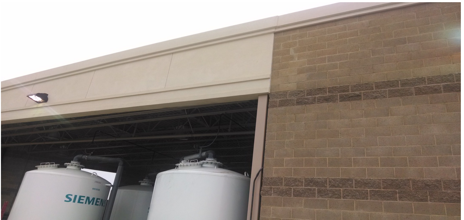
Below: Photo of the front of the building facing the Landfill Gas pad. The building and roof are completed except for the final installation of the fire water system prior to operation.
