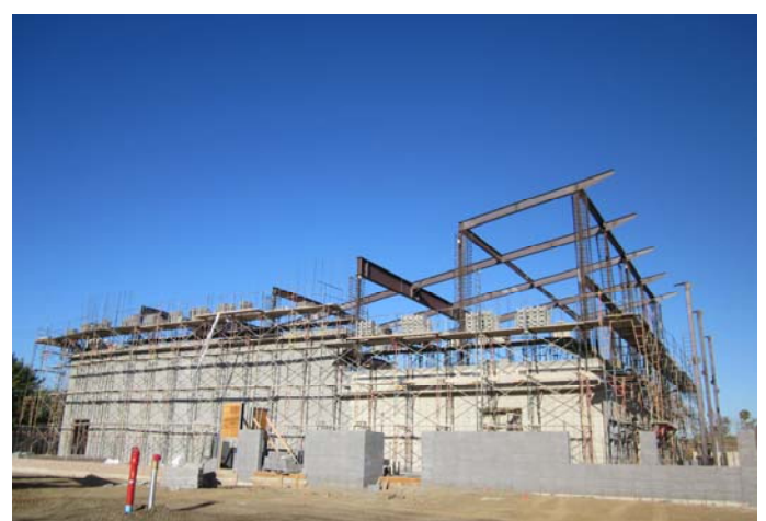
CMU Installation (Gym Area)
