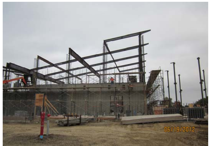
CMU Installation (Gym Area)
