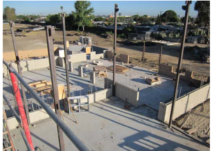
CMU Installation (Remaining Areas)
