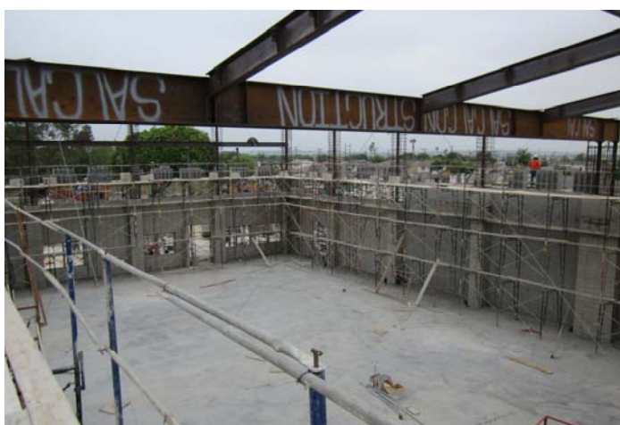
CMU Installation (Gym Area)
