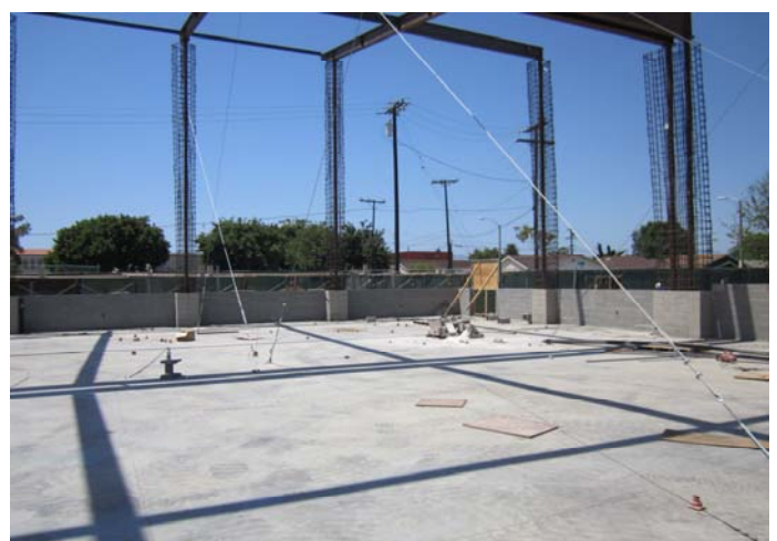
CMU Installation (Gym Area)
