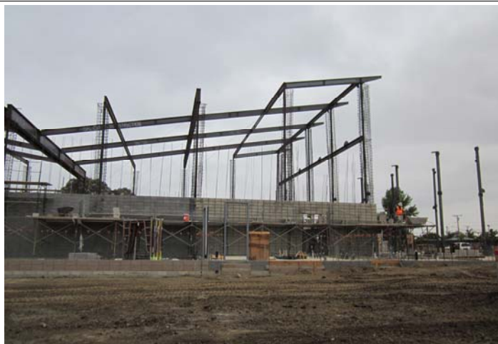
CMU Installation (Gym Area)
