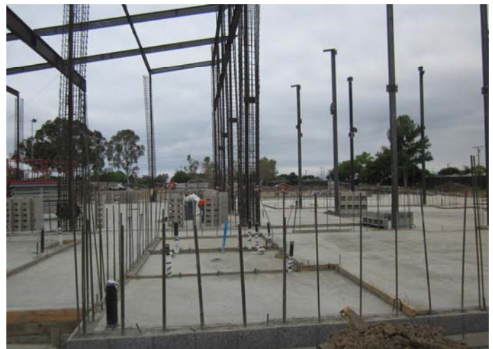
Remaining Areas — Concrete Slab Completely Poured
