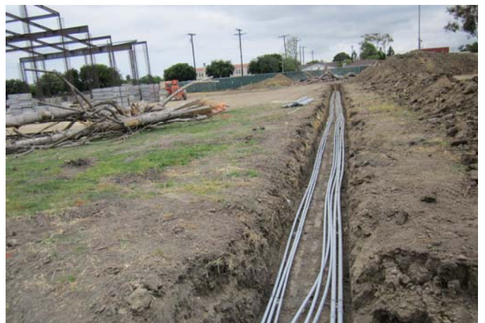
Field Underground Electrical Conduit Installation
