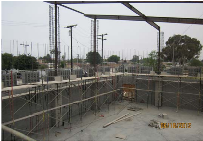
CMU Installation (Gym Area)
