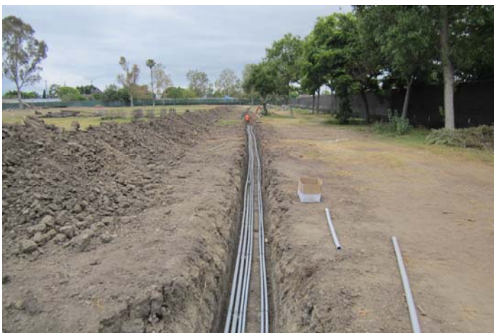
Field Underground Electrical Conduit Installation
