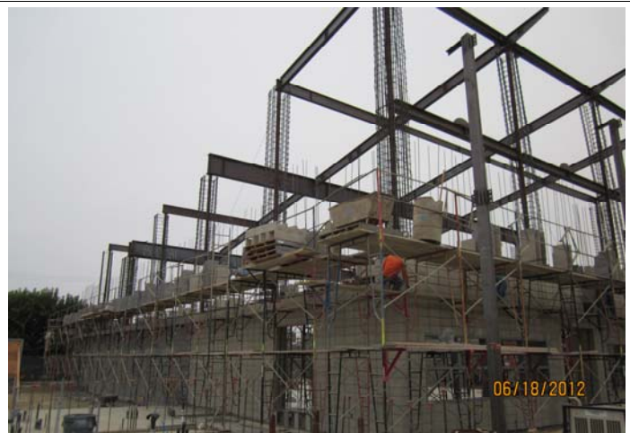
CMU Installation (Gym Area)
