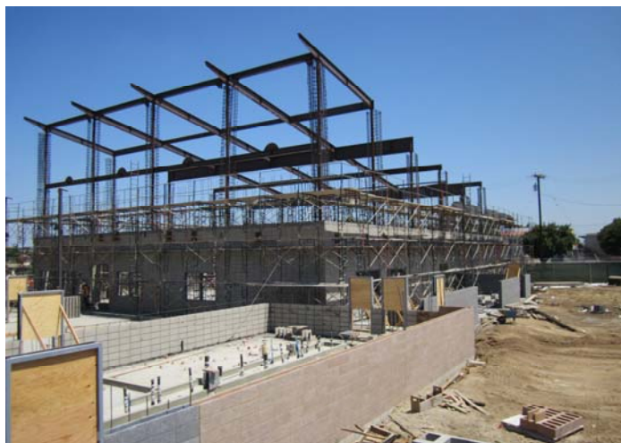
CMU Installation (Gym Area)
