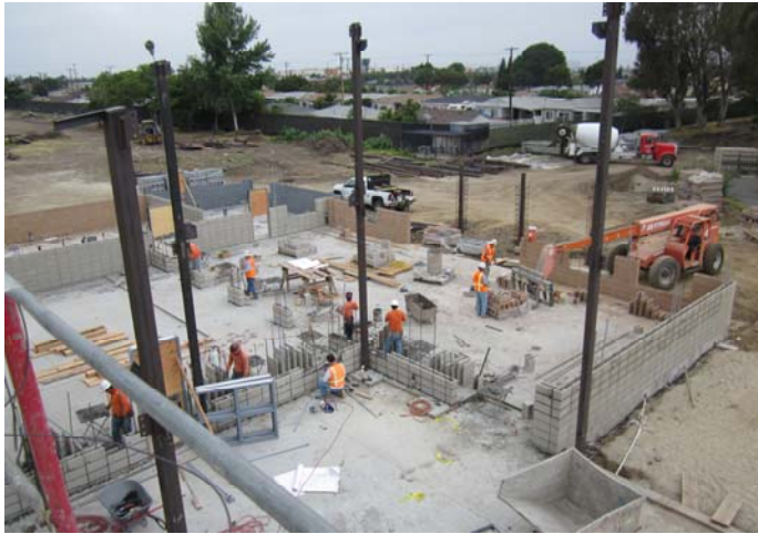
CMU Installation (Remaining Areas)
