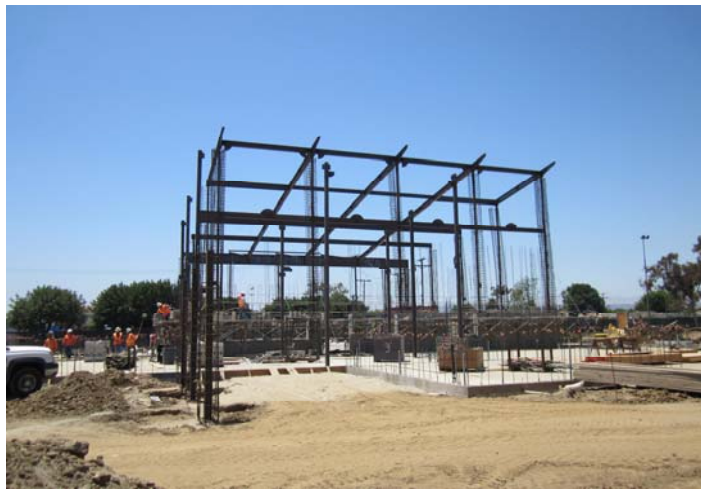
CMU Installation (Gym Area)
