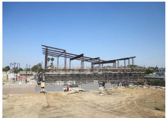
CMU Installation (Gym Area)
