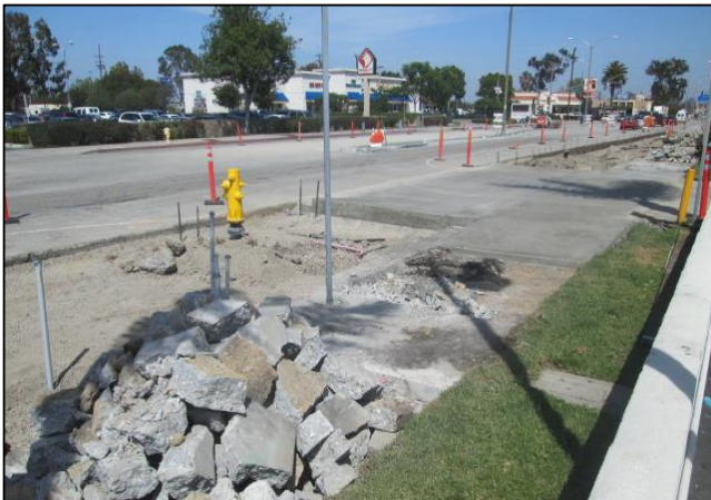
At CVS Driveway Open for Traffic
