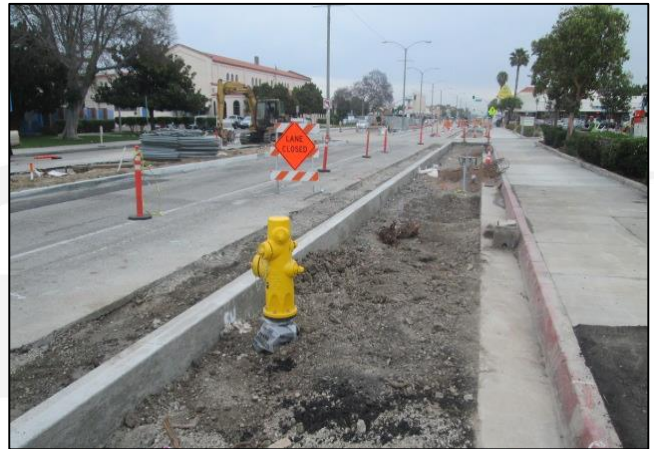
Relocated Hydrant Front of Albertsons
