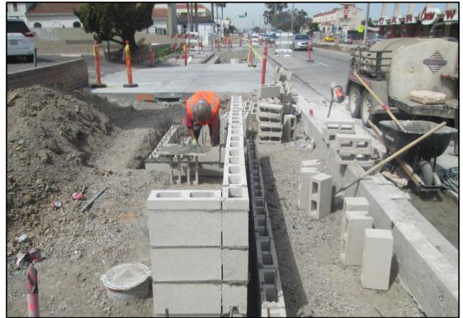
Seating Node Excavation for Footing
