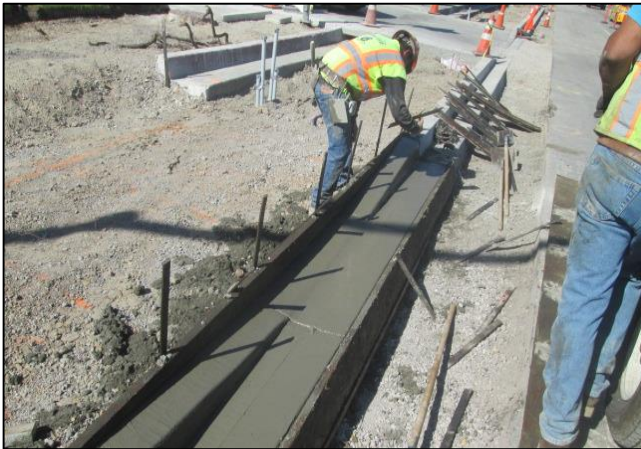
New Curb and Gutter at Orrick
