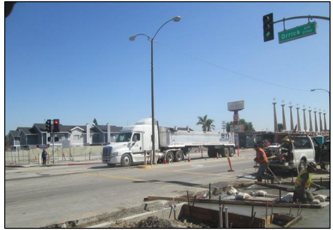
End Dumps Hauling Spoil from Water Line Excavation
