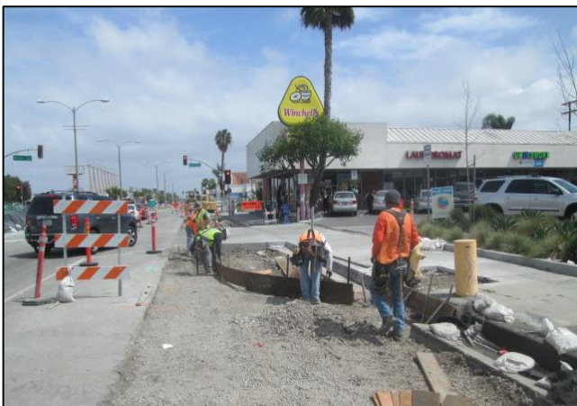
Preparing for Concrete
