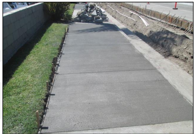
New Sidewalk at CVS
