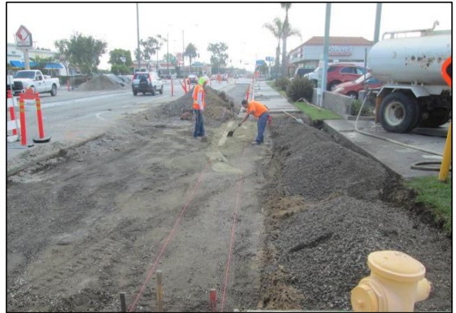
Preparing for Culvert Placement
