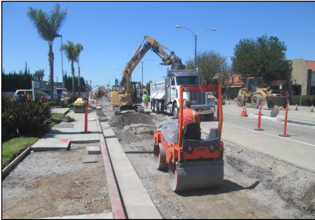
Compaction Underway
