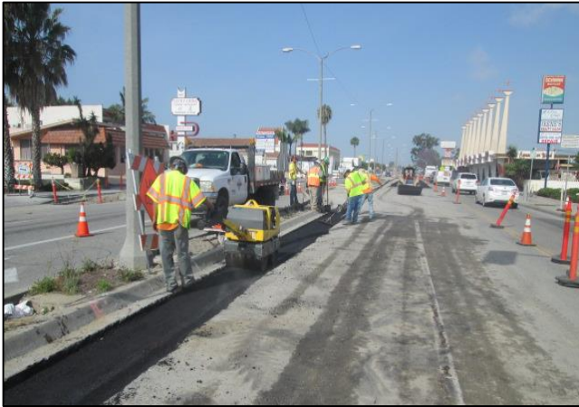
Base Paving Recycle Water Trench
