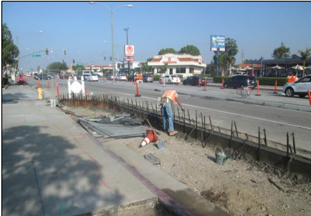
Bump Out Curb and Gutter Poured
