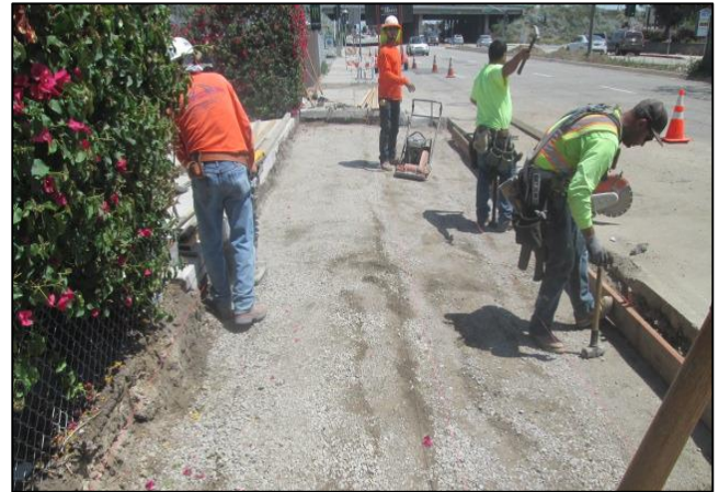
Forming Drive Way at Station 12+00
