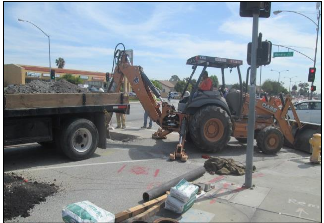
Cal Water Relocating Fire Hydrant
