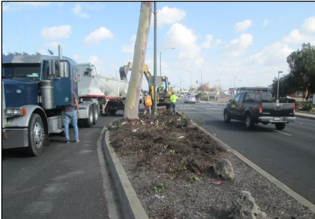
Clear and Grubbing on Avalon
