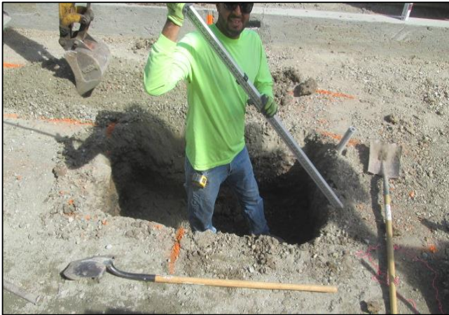
Seating Node Wall Under Construction
