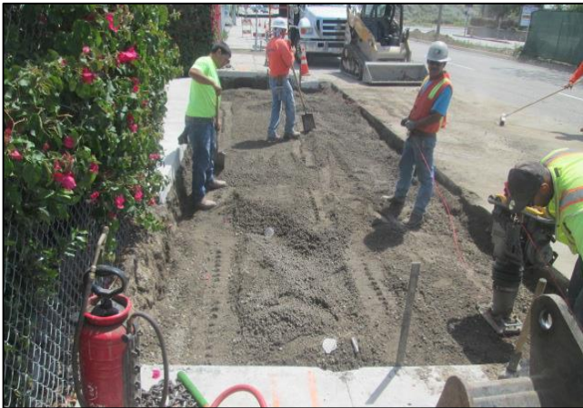
Compacting CMB at Station 12+00 Driveway
