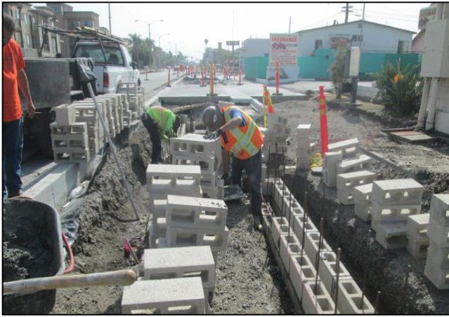
Seating Nook CMU Walls Under Construction
