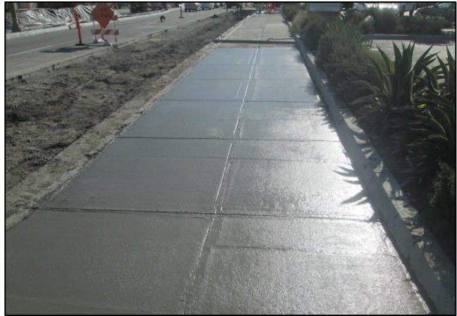
Sidewalk Paveback
