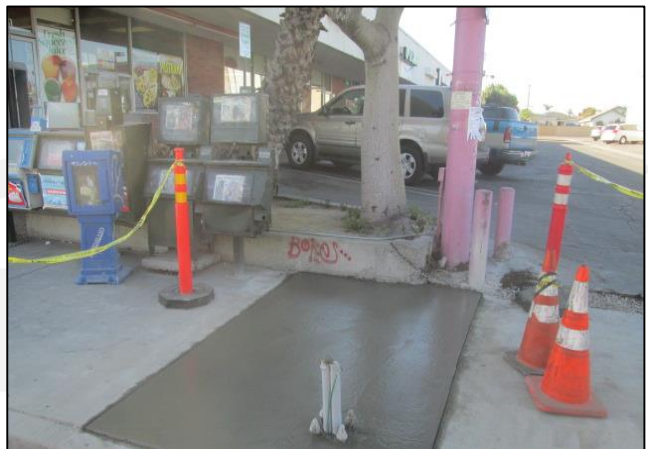
Sidewalk Pave Back at Winchell's
