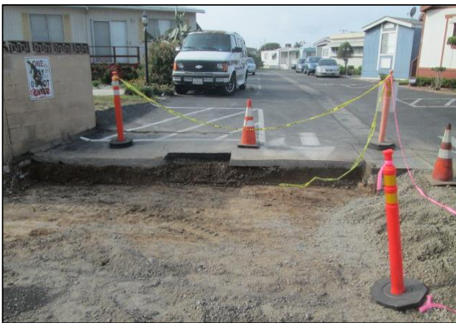
Mobile Home Park Driveway Removal
