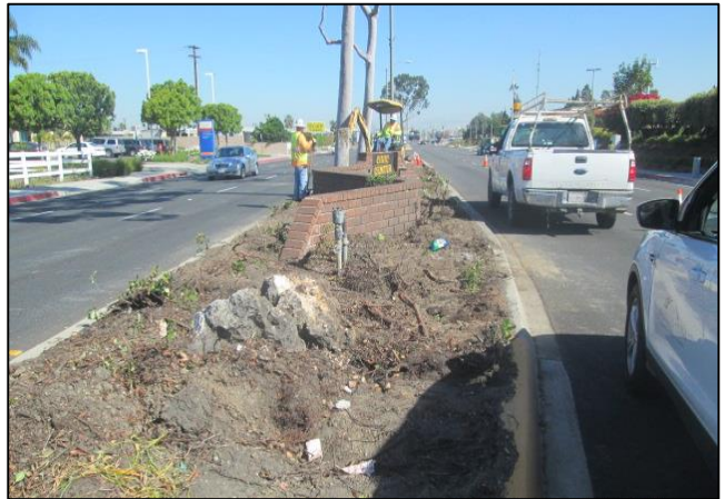
Spoil Pile to be Removed
