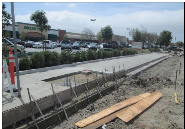
Preparing Bus Shelter
