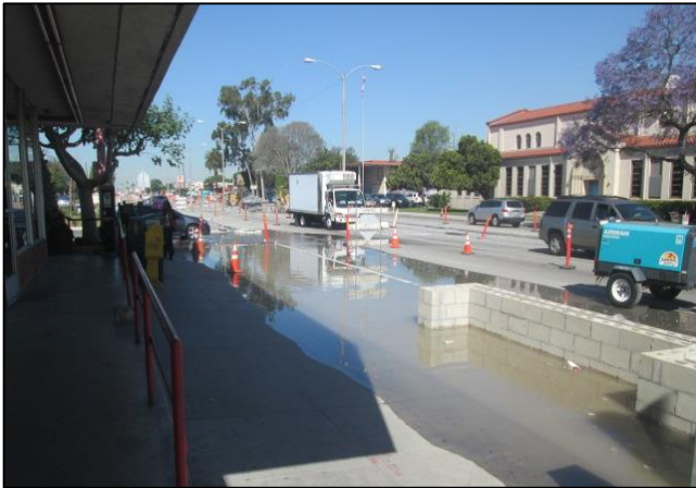
Flooding from Line Break
