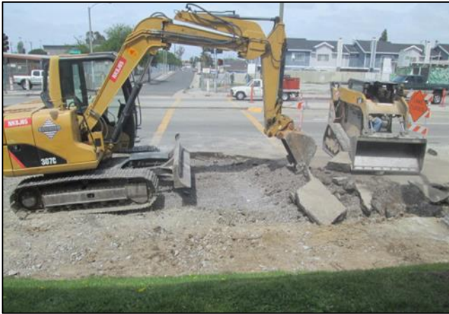
Removal for Future Bump Out
