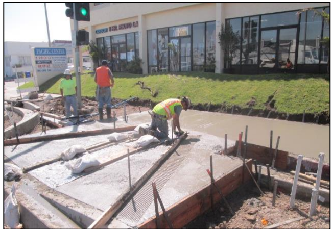
ADA Ramp at Orrick
