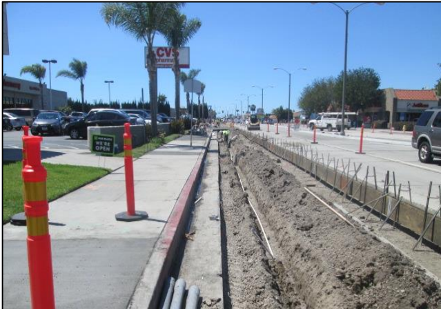
Conduit Trench at CVS for Curb and Gutter
