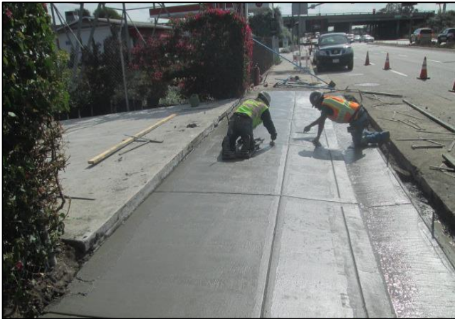
Driveway at LAPW Easement
