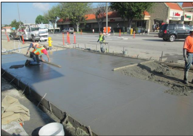
Driveway with Culvert at CVS
