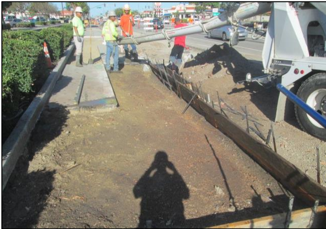
Sidewalk Placement
