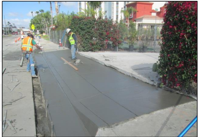
PCC Placement Drive Way Station 12+00
