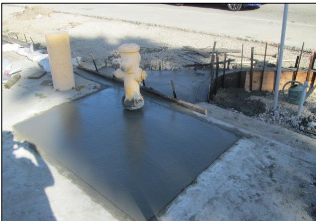
Sidewalk and New Curb and Gutter at Bump Out
