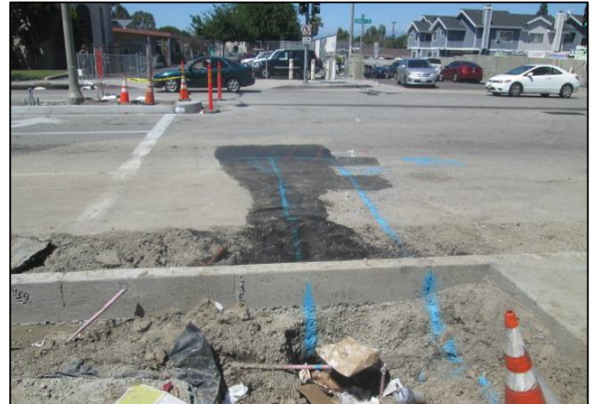
Cal Water Replaced Broken Line
