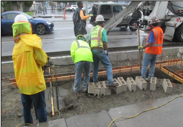
Seating Node Under Construction at Winchell's
