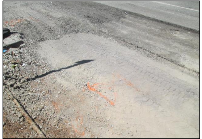
ATT Line was Marked
