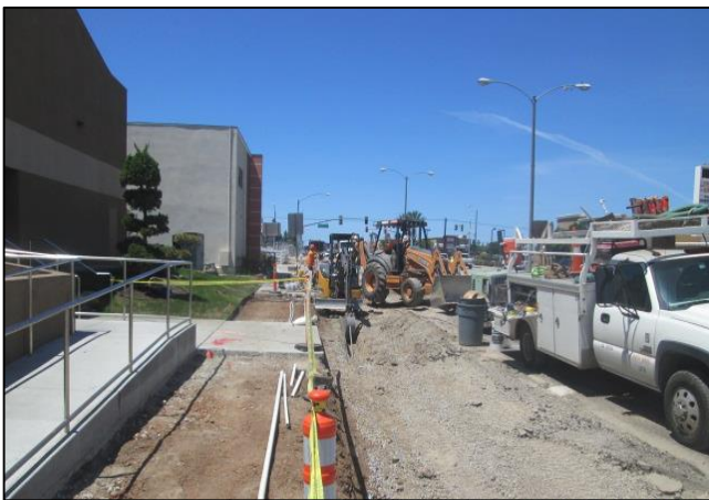
Crew Relocating Hydrant East of Fig.
