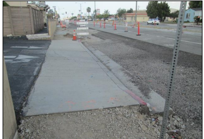
Driveway to be Removed and Replaced
