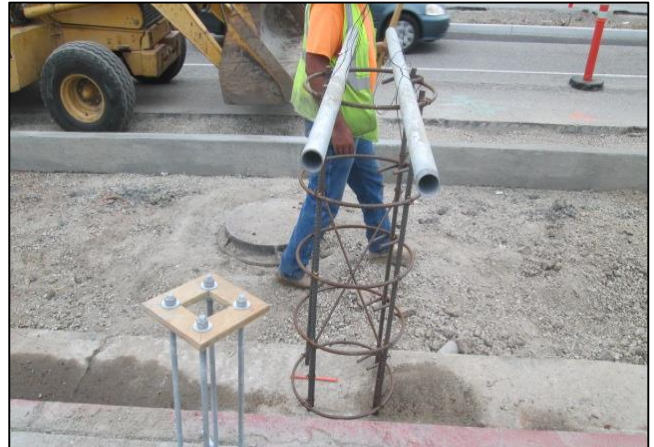
F-1 Pedestrian Light Foundation Rebar Cage
