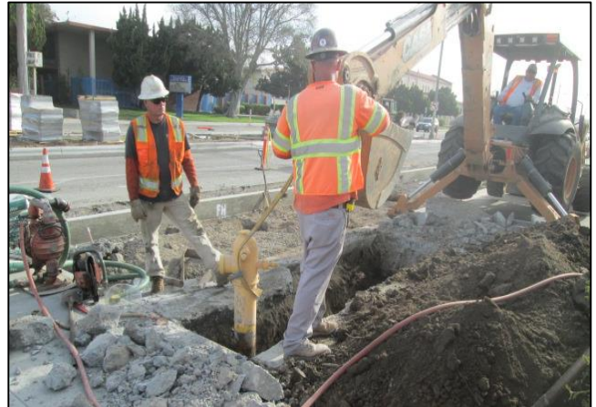
Relocating Hydrant Front of Albertsons
