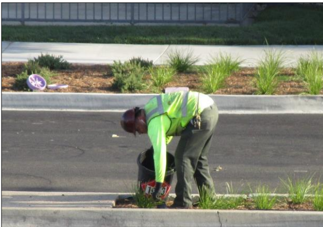
Removing trash and weeds entire site.
