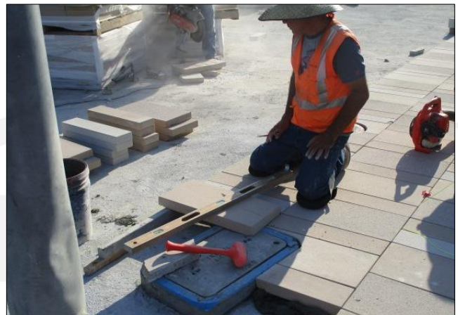
Architectural pavers installed at City Hall.
