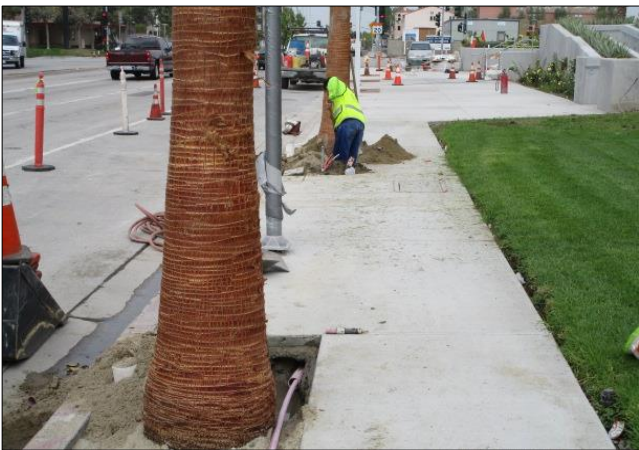
Extending irrigation lateral at City Hall.
