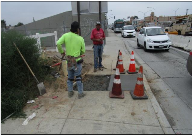
Placing sidewalk south side west of Figueroa.
