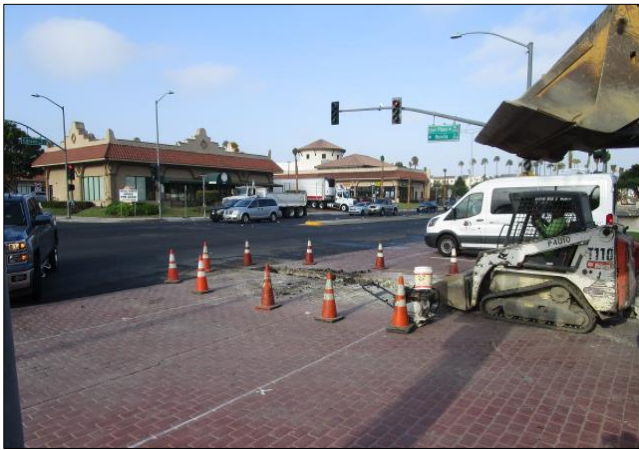
Removing asphalt concrete patch Civic Center Plaza.
