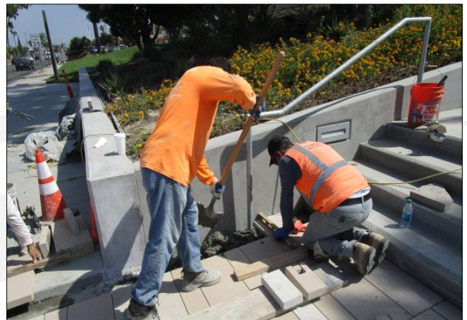
Placing Architectural Pavers at City Hall.
