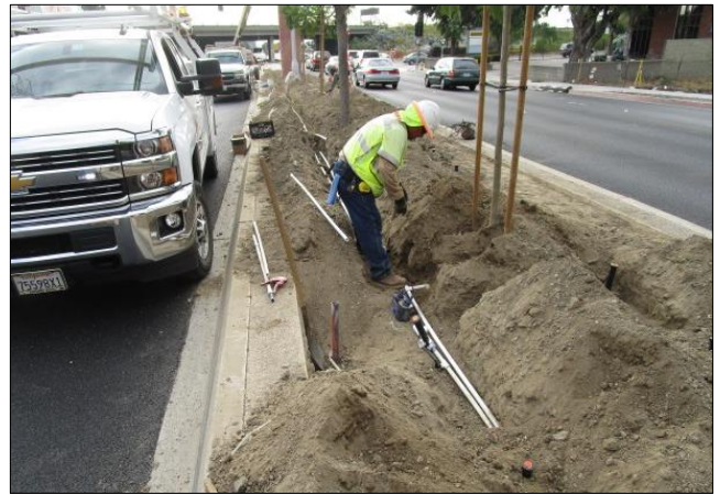
Installing irrigation in median east of Avalon.
