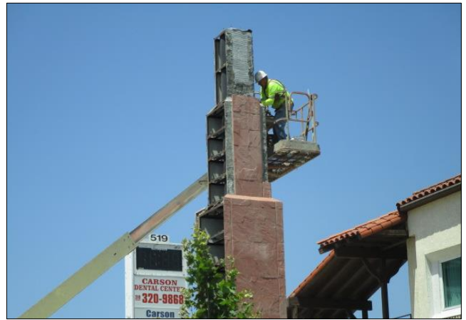
Installing tiles on monument tower.
