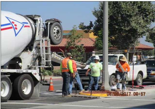
Placing red stamped curb in Avalon median nose.
