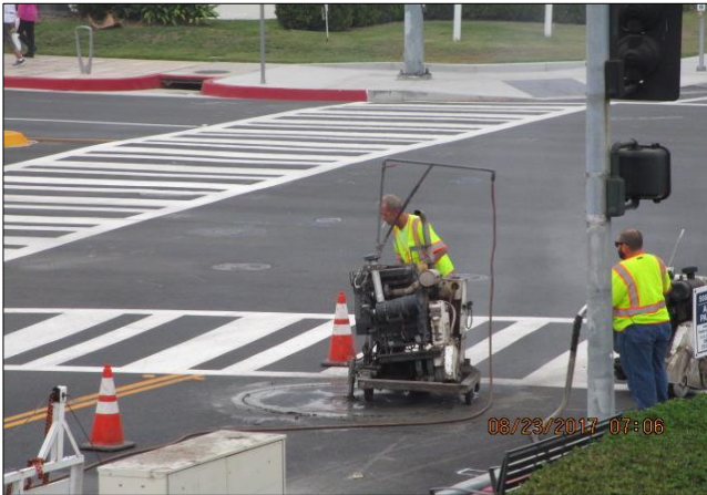
Sawcutting detector loops at Grace and Carson.
