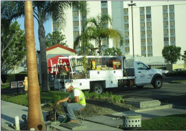
Wiring palm tree uplights east of Avalon.
