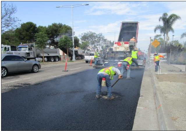
Paving westbound Carson.
