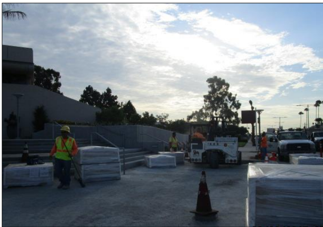
Architectural pavers delivered to City Hall.
