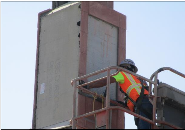
Removing tiles top tiers of monument towers.
