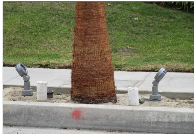
F5 uplights installed south side east of Avalon
