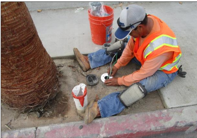
Installing F5 uplights on south side.
