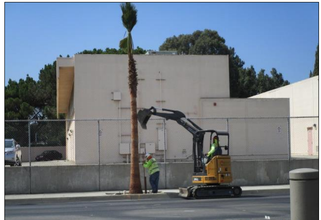
Straightening leaning palm trees on Carson.
