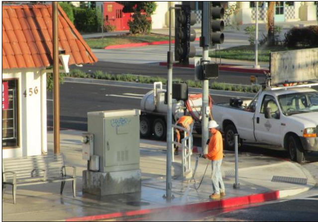
Pressure washing USA marks.
