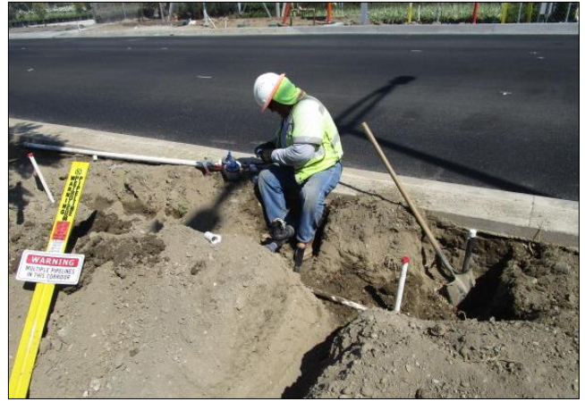
Installing sprinkler heads on Carson median east end.
