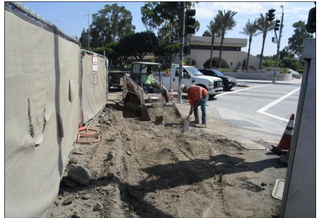
Demolition on northwest corner Avalon and Carson.
