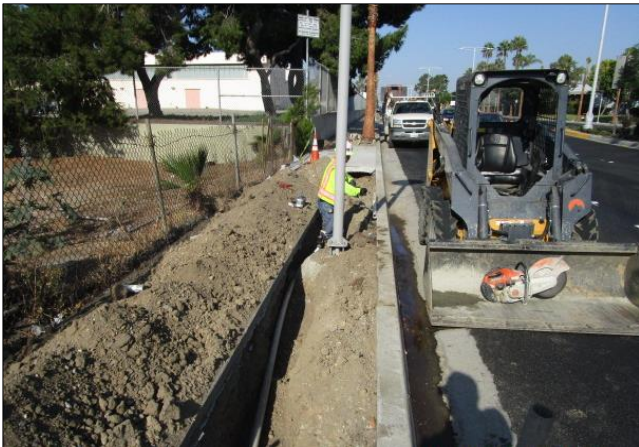
Installing irrigation south side of west of I-405.
