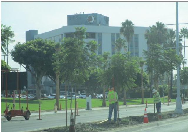
Installing sprinkler heads on Carson median.
