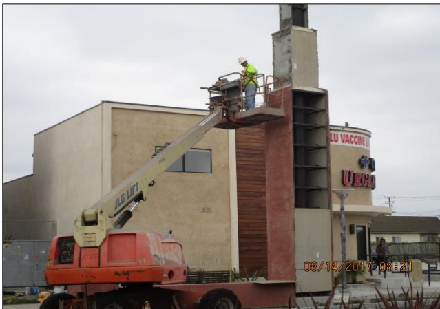
Installing tiles on monument tower south side.
