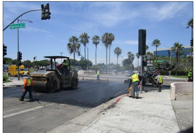
Paving Carson and Bonita intersection.
