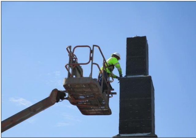
Applying scratch coat to monument west of I-405
