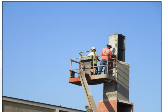
Removing tile from monument towers.
