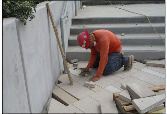
Placing Architectural Pavers in front of City Hall.
