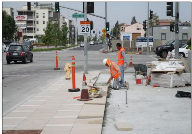
Architectural pavers installed at City Hall.
