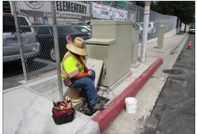
Splicing Detector Lead-in Cable (for traffic loops).
