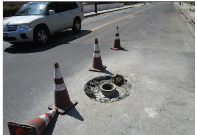
Adjusting water valve to grade.
