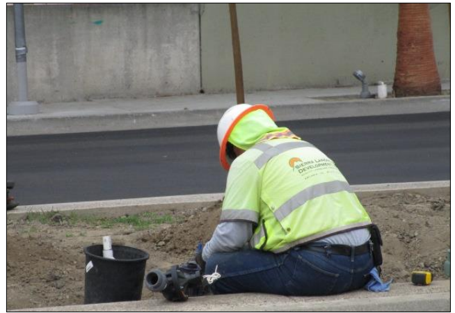
Installing remote control valve on Carson median.
