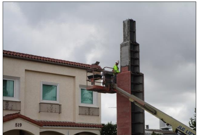
Installing tiles on monument tower north side.
