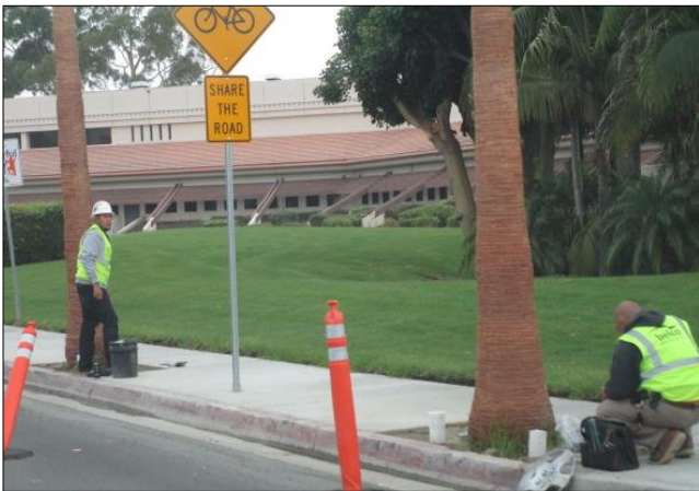
Installing wiring for palm tree uplighting.
