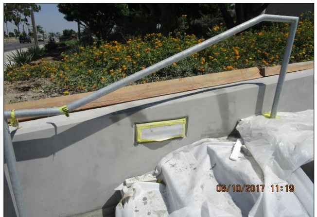
Finishing concrete work at City Hall.
