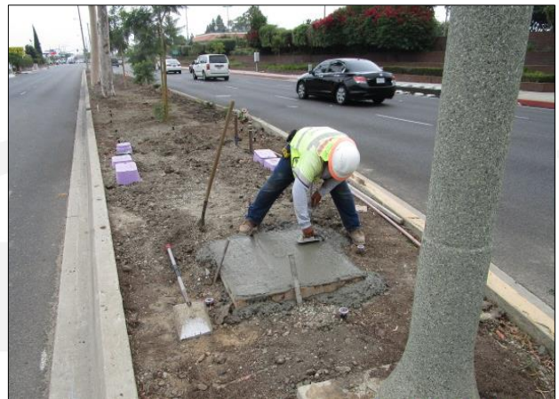
Placing foundation for solar panel pole on Avalon median.
