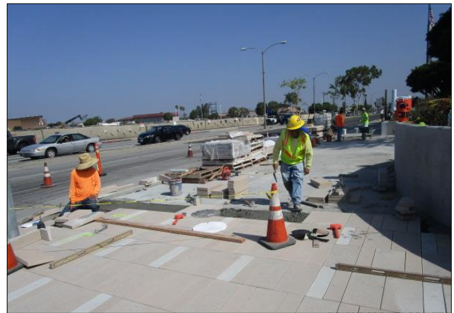
Placing Architectural pavers at City Hall.
