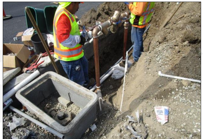
Installing flow sensor west of I-405.
