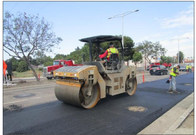
Compacting paving on Carson.
