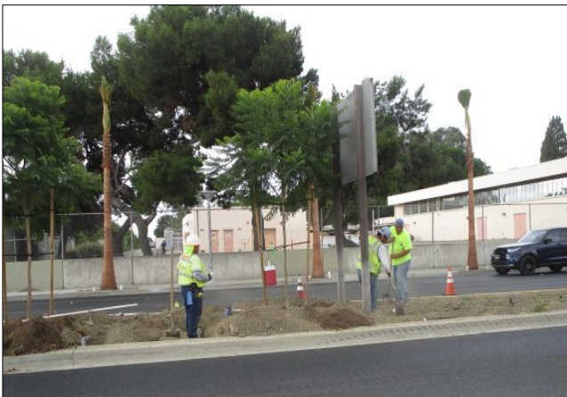
Installing irrigation Carson median east of Avalon.
