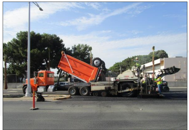
Paving eastbound Carson.
