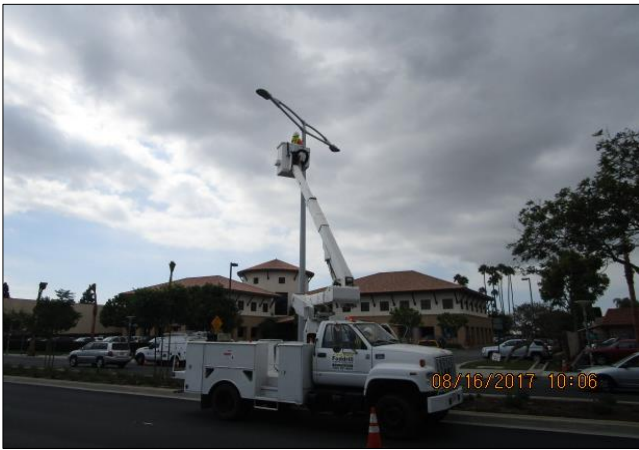
Installing receptacle covers on streetlights.
