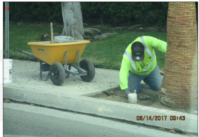
Installing F5 lighting on south side east of Avalon.
