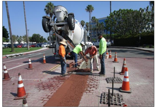
Placing red stamped concrete Civic Center Plaza.
