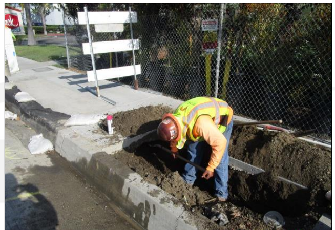
Installing irrigation lateral west of I-405.
