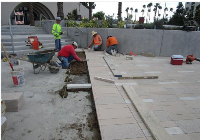
Placing Architectural pavers in front of City Hall.
