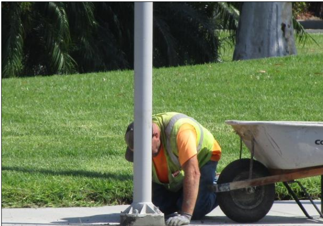
Dry packing pedestrian light poles east of Avalon.
