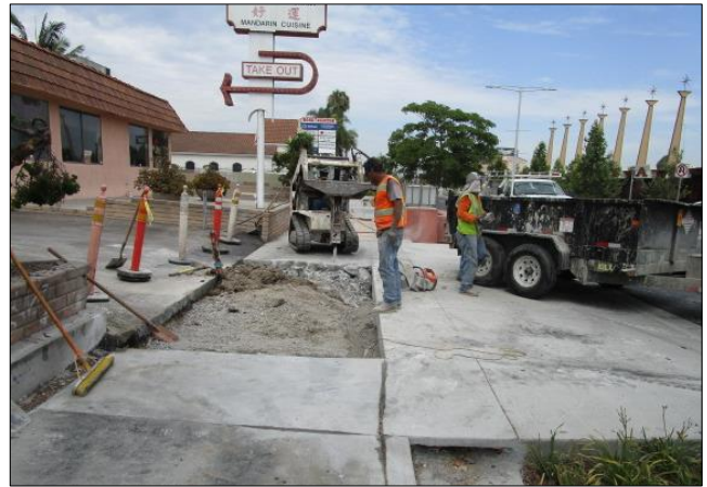
Driveway section removed west of Dolores.
