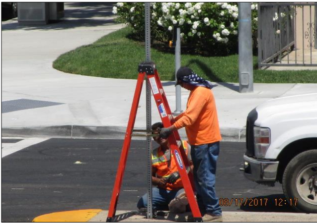
Installing "No U-Turn" signs.
