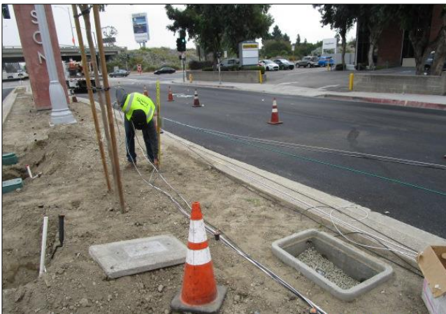
Installing wiring for pin letters on monument tower.
