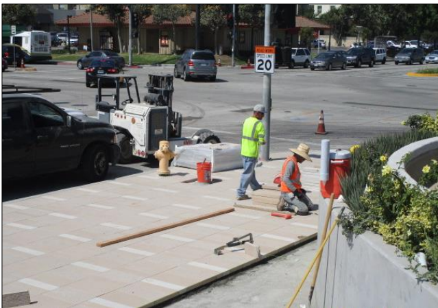
Placing Architectural pavers in front of City
