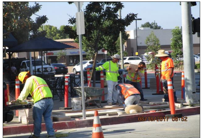
Architectural pavers on south east corner of Carson and Avalon.
