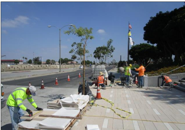
Placing Architectural Pavers at City Hall.
