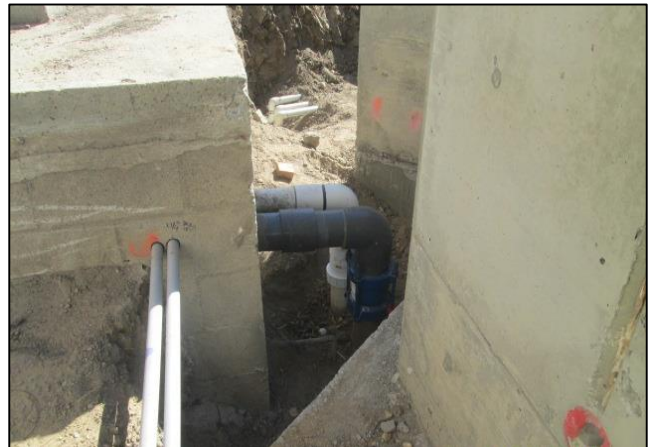
Reconnected Fountain Lines at City Hall
