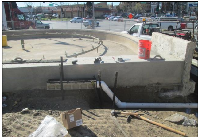
City Hall Area Drain Line Installation
