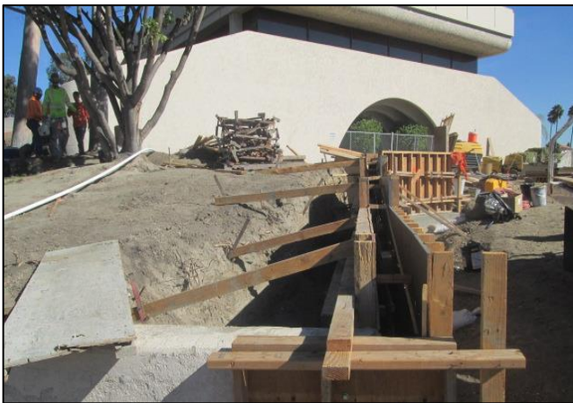
City Hall Retaining Wall Forms
