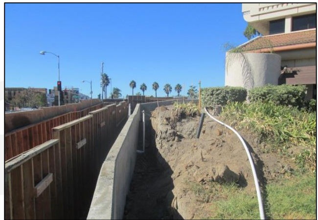
City Hall ADA Ramp Walls
