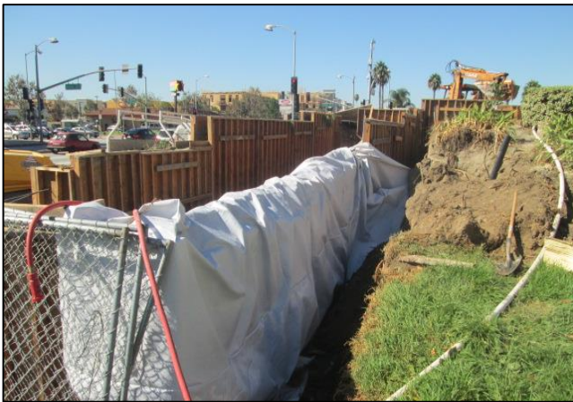
West Blanket Cure of PCC Retaining Walls at City Hall
