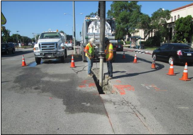
Potholing on Carson St
