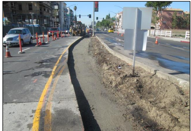
Compacted Subgrade/Base for New Median Curb/Gutter
