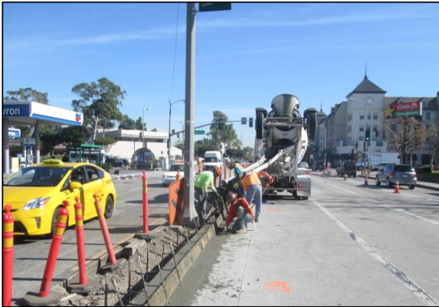
Median Curb/Gutter Placement
