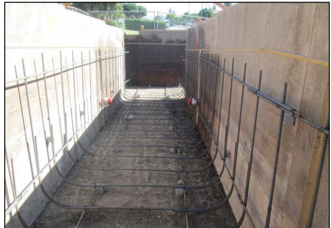
Rebar Placement Along City Hall ADA Ramp
