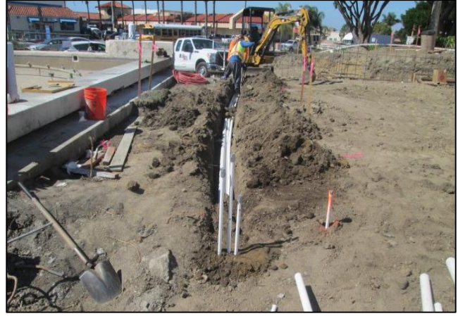
Placement of Irrigation Lines Adjacent to City Hall Fountain
