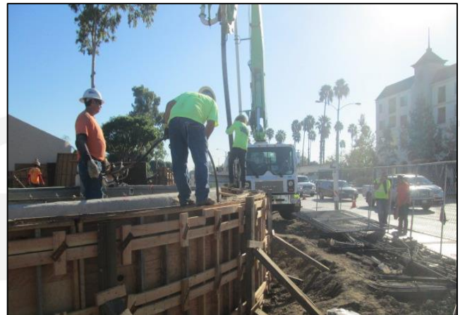
City Hall Fountain Planter Wall PPC Placement
