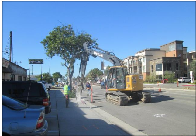
Curb/Gutter Demolition, Eastbound Carson St
