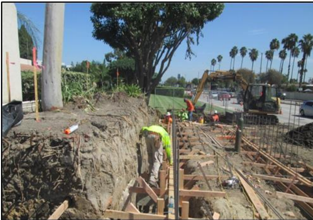
ADA Ramp Retaining Wall Rebar Placement
