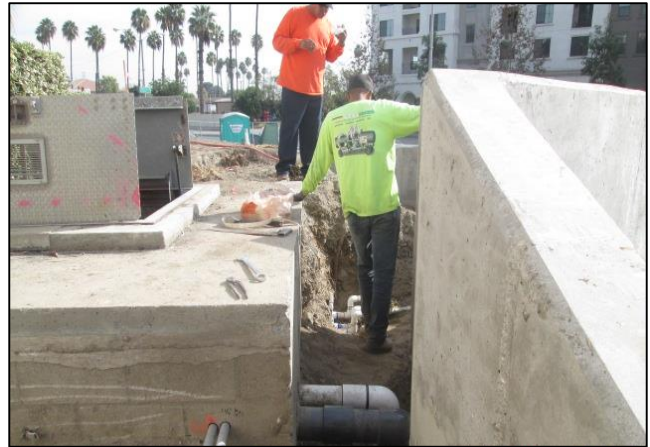
Pressure Testing City Hall Fountain Lines
