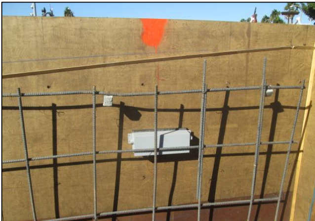
Recessed Lighting Installation in City Hall Retaining Wall
