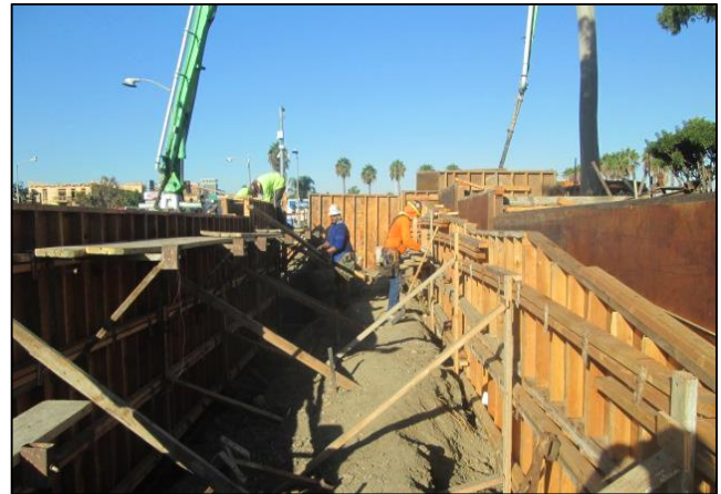
City Hall ADA Ramp Retaining Wall PCC Placement
