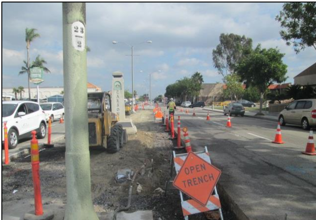
Median Clear/Grub and Traffic Control
