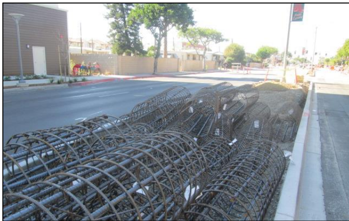
Rebar Cages for Median Street Light Foundations
