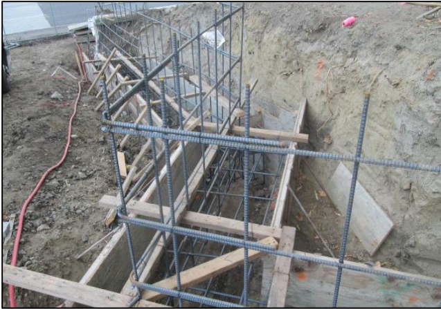
Forms/Rebar for Retaining Wall West Side of City Hall
