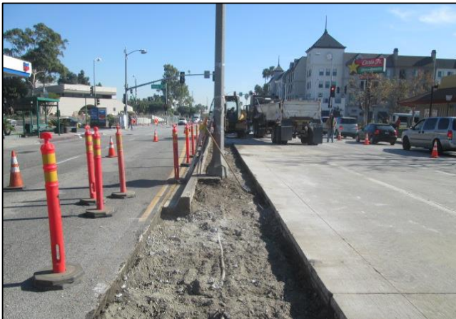
Median Curb Removals
