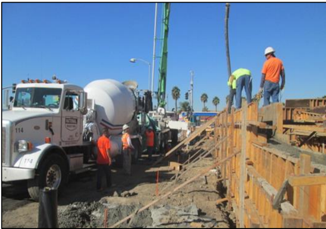
City Hall ADA Ramp Retaining Wall PCC Placement
