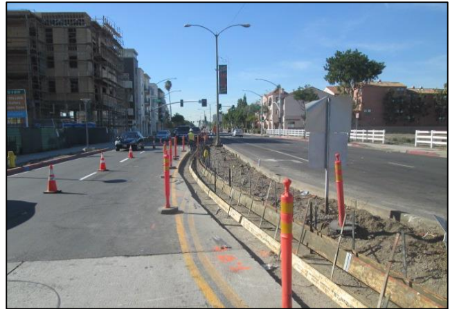
Forms for New Median Curb/Gutter
