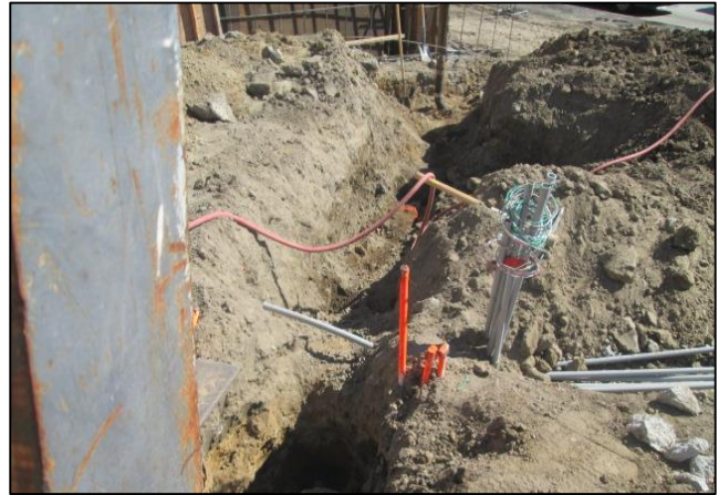
Pipe Trenches and New Conduit at City Hall
