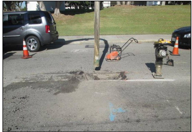
Potholing on Carson St
