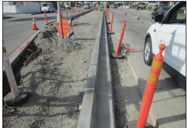
New Median Curb/Gutter
