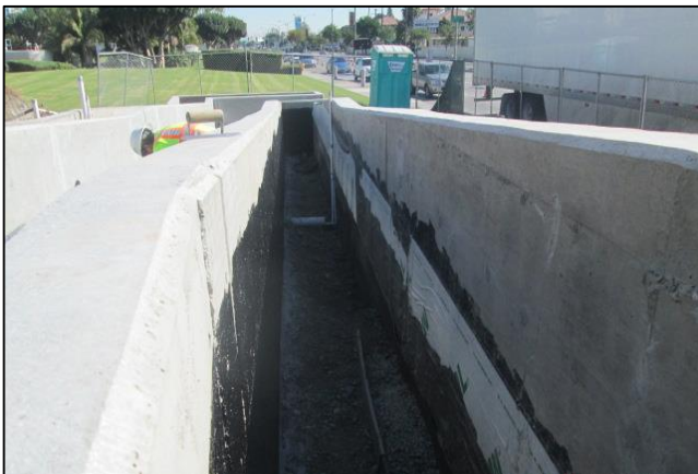
Waterproofing Membrane Installation at City Hall ADA Ramp Planters
