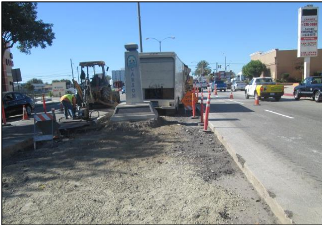
Median Clear and Grub at Carson St /Figueroa St
