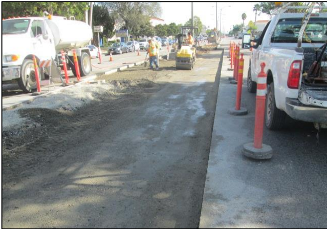
Compacting for New Median Curbs
