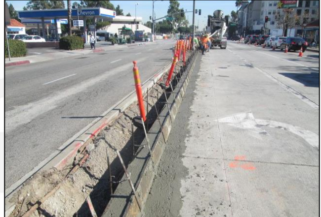
Median Curb/Gutter Placement
