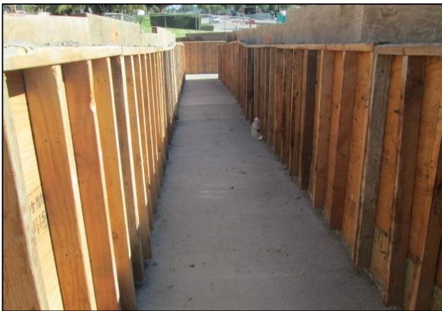
Completed City Hall ADA Ramp
