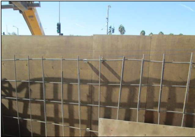
City Hall Retaining Wall Rebar Placement
