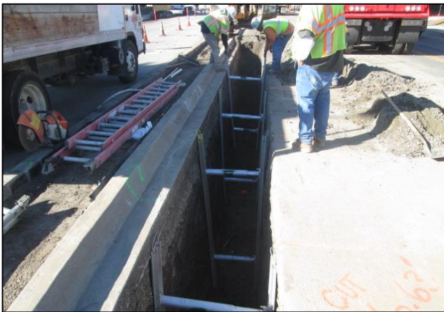
Placement of Shoring in Recycled Water Line Trench
