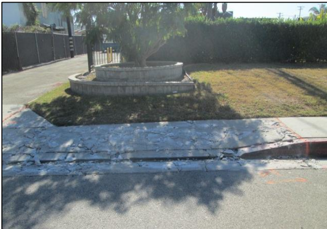
Driveway Demolition, Eastbound Carson St
