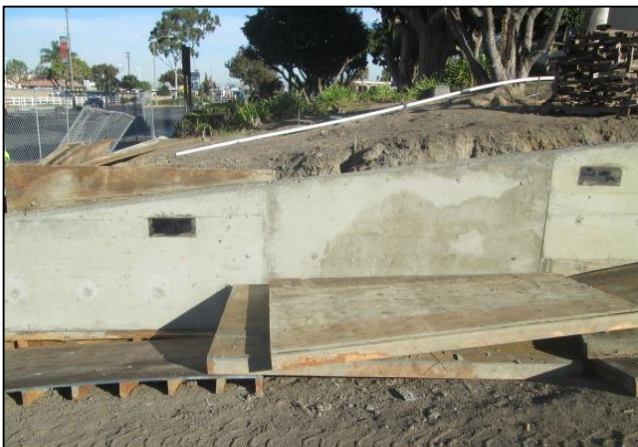
City Hall Retaining Wall and Recessed Lights
