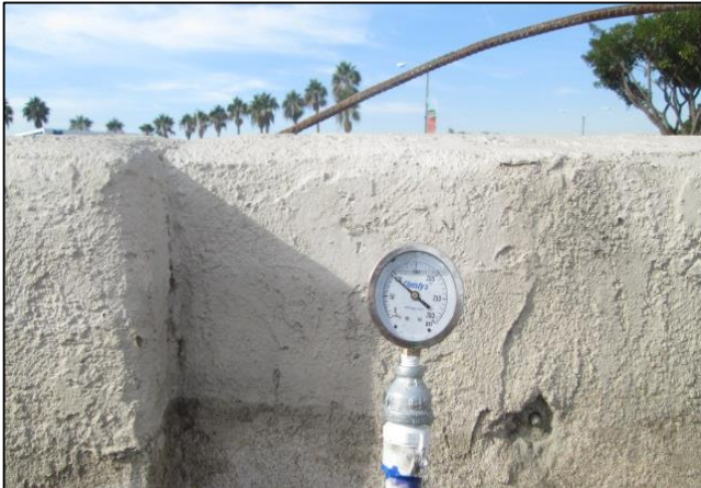
Pressure Testing City Hall Fountain Lines
