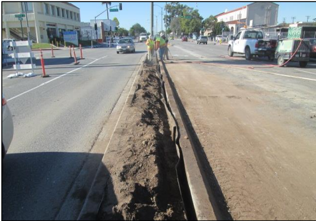
Moisture Barrier Placement Behind Median Curbs
