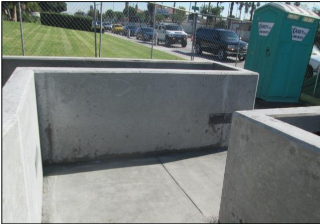
City Hall ADA Ramp
