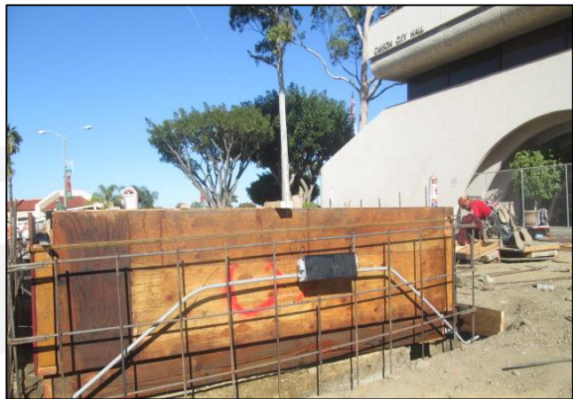
Rebar/Conduit/Recessing Lighting Placement at City Hall Planter
