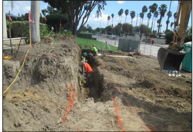
Excavation for ADA Ramp Retaining Wall
