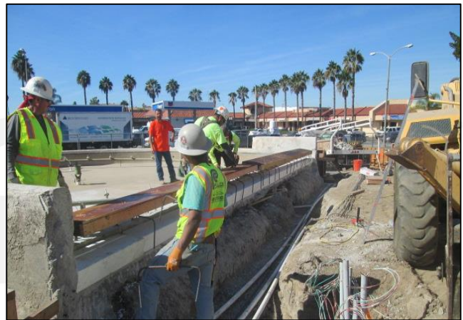
Forms/Rebar for New City Hall Fountain Bench
