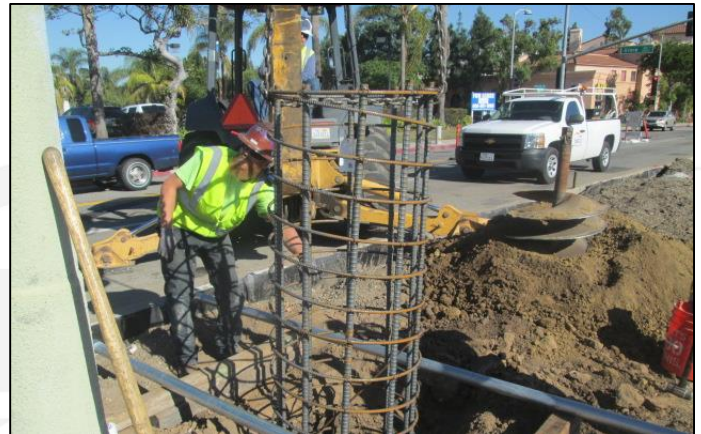
Rebar Cage Placement for Median Streetlight Foundation
