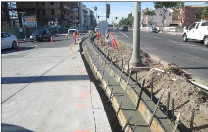
Median Curb/Gutter Placement
