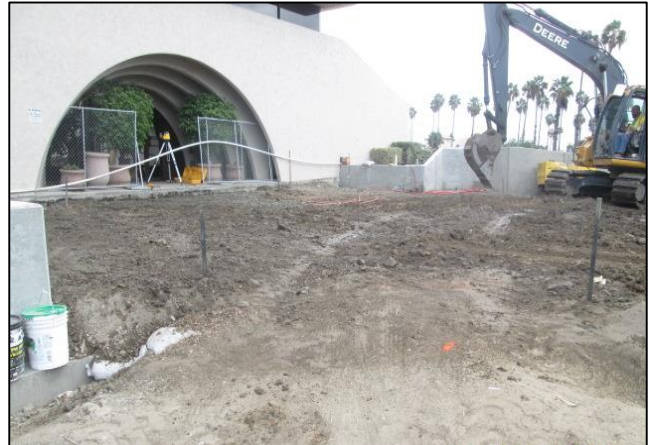
Grading at City Hall Entranceway
