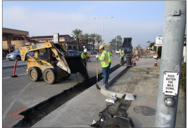
Paving slots on north side west of Moneta.
