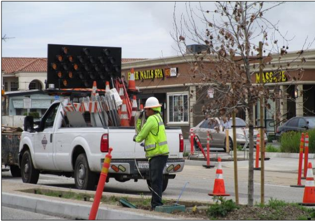
Pulling irrigation control wire.
