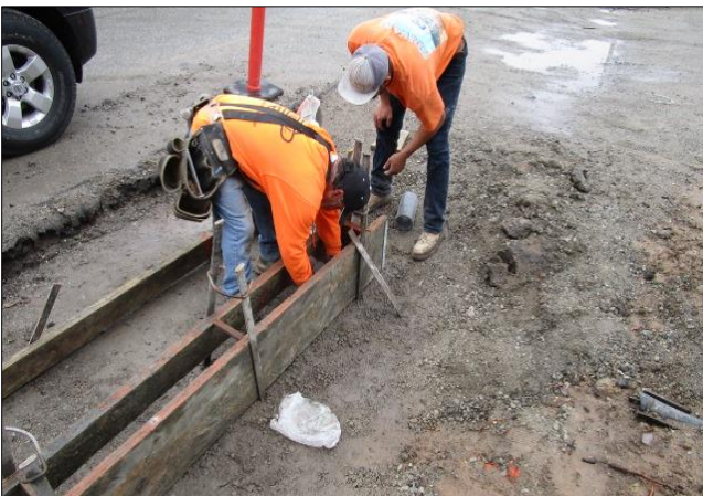
Forming curb and gutter north side east Figueroa.
