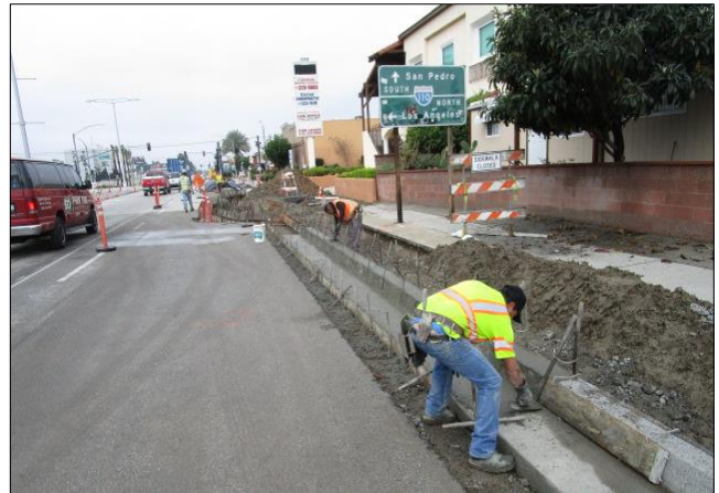
Finishing curb and gutter east of Figueroa.
