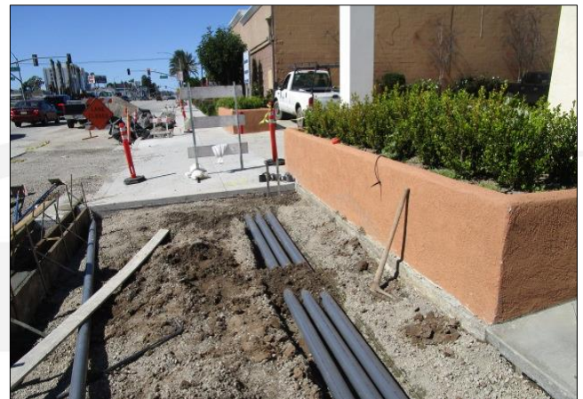
Placing drainpipes on north side east of Figueroa.
