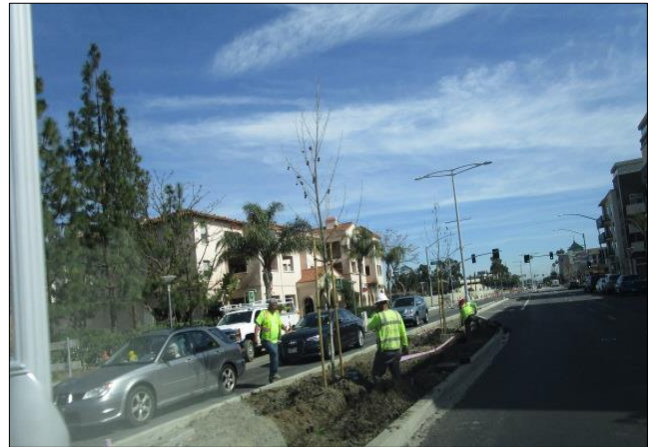
Installation irrigation control wire in median.
