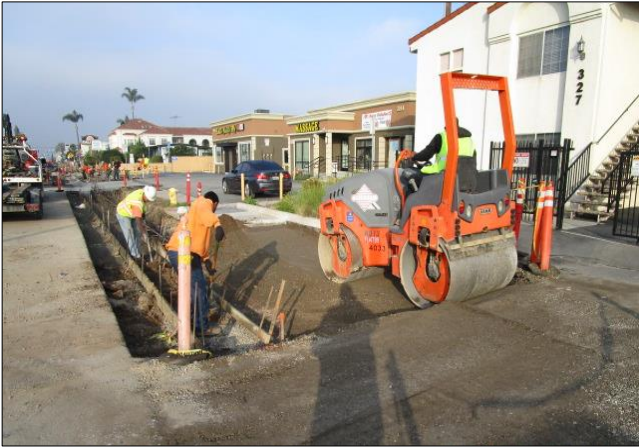
Grading and compacting base.
