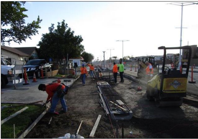
Grading and forming driveways and culvert.
