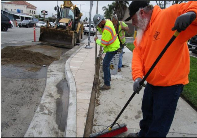
Decomposed granite test strip at Credit Union.
