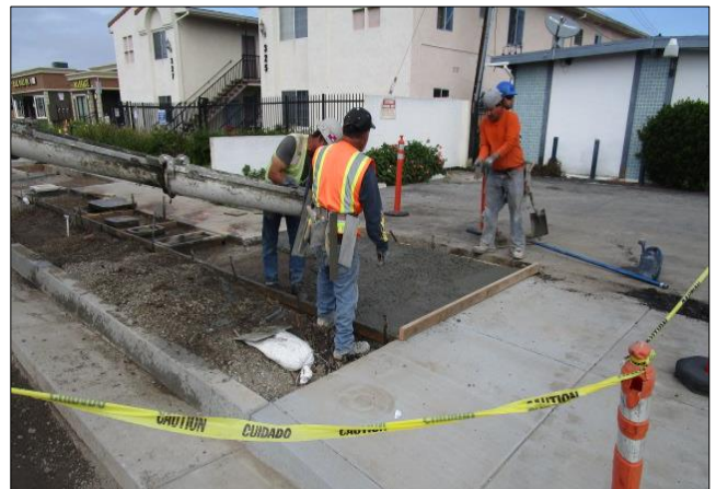
Placing sidewalk on north side west of Moneta.
