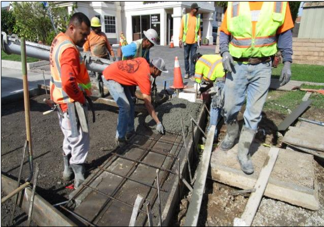
Parkway drain north side west of Moneta.
