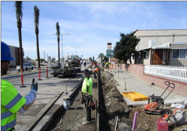
Forming curb and gutter on north side east of Figueroa.
