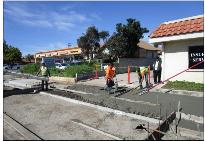
Placing driveway and culvert east Main north side.
