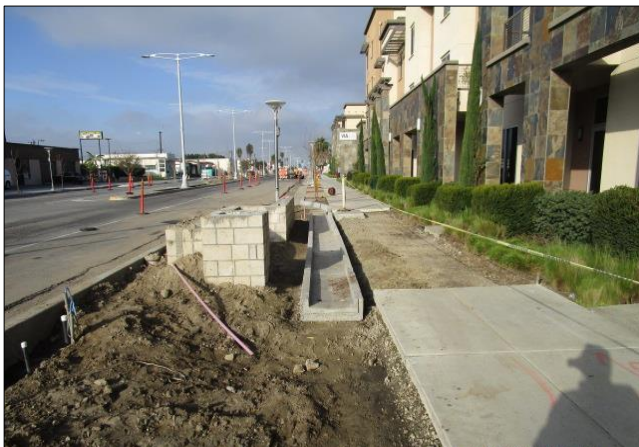
Installing pedestrian drainage culvert.
