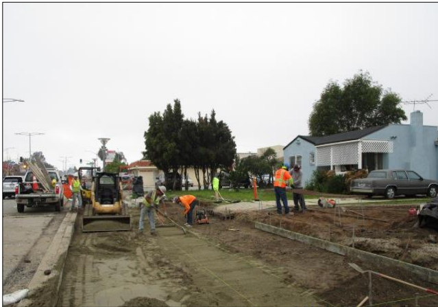
Grading and forming driveways and culvert.
