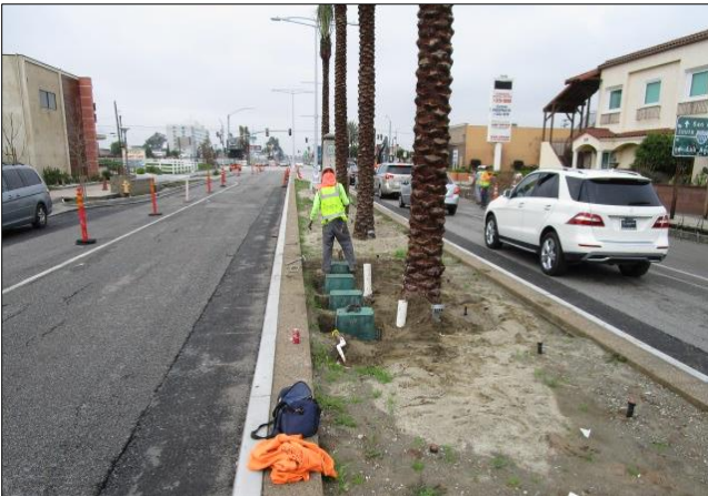
Installing remote control valve boxes in median.
