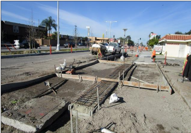
Grading and forming driveways and culvert.
