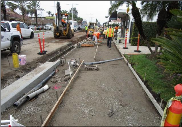
Sidewalk and driveway formed and compacted.
