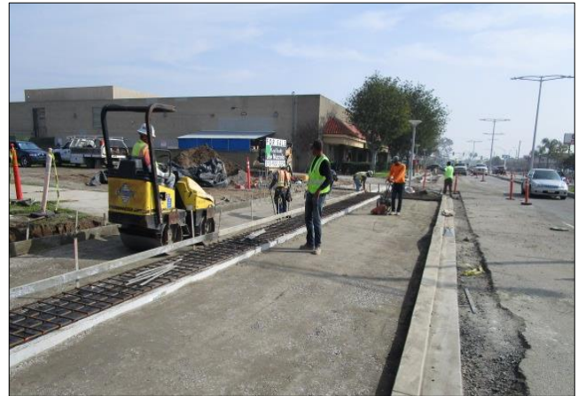
Compacting driveway on north side west of Main.
