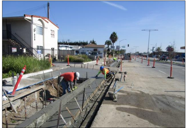
Finishing curb and gutter on north side east of Figueroa.
