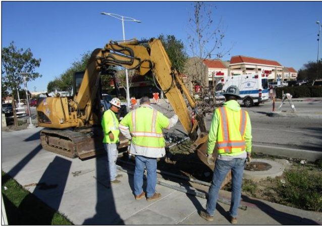
Clearing culvert of Styrofoam and debris west of Main.
