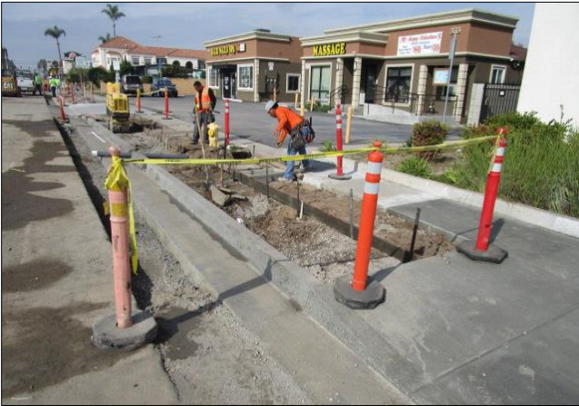
Forming sidewalk north side east of Figueroa.
