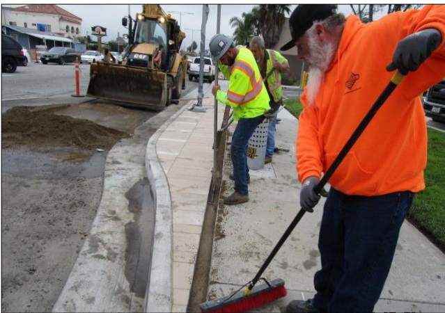
Decomposed granite test strip at Credit Union.
