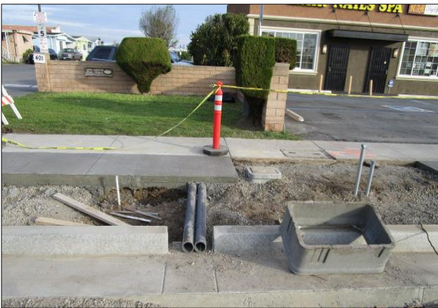
Drain pipes extended under parkway.
