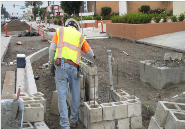
Constructing concrete masonry unit seating wall.
