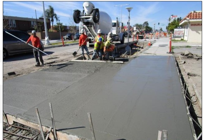
Placing driveway and culvert on north side west of Main.
