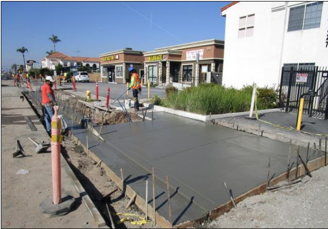
Finishing driveway and sidewalk east of Figueroa.
