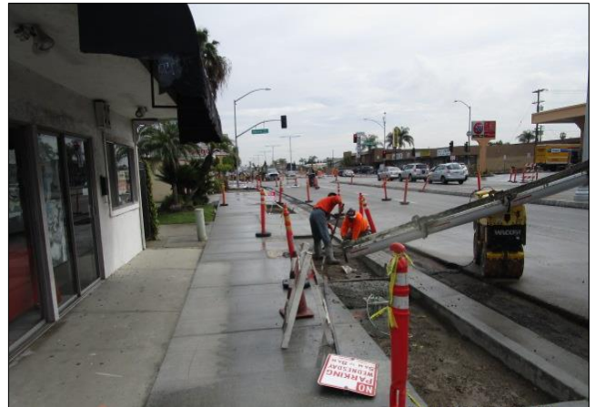
Placing underslab for pavers.
