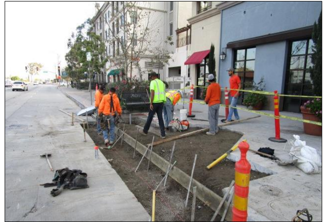
Forming curb ramp on Avalon south of Carson.
