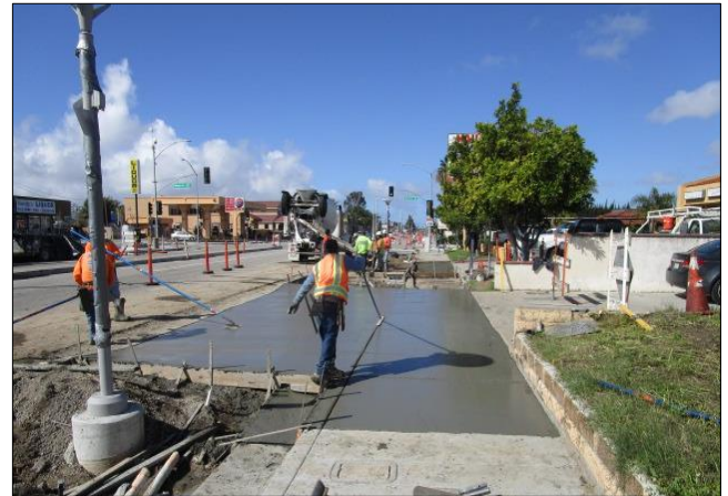
Placing driveway and culvert on north side east of Moneta.
