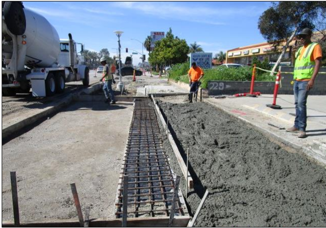
Paving driveway and culvert.
