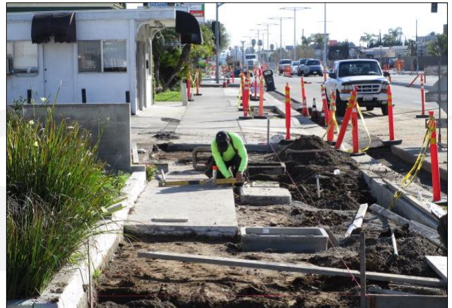
Forming sidewalk on north side west of Moneta.
