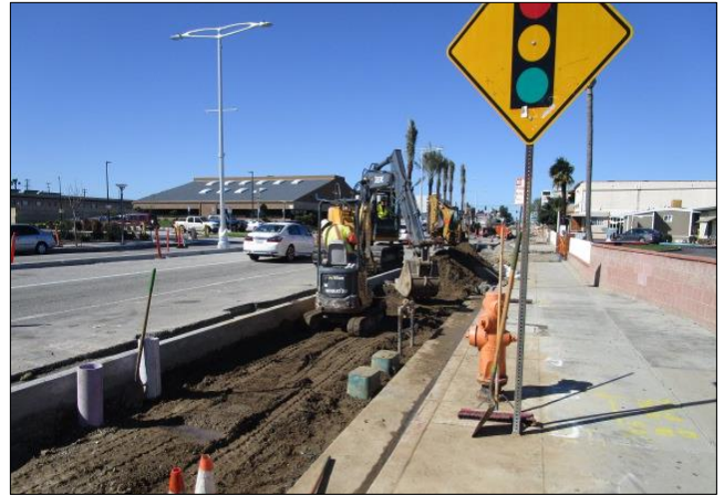
Replacing unsuitable soil on north side east of Figueroa.
