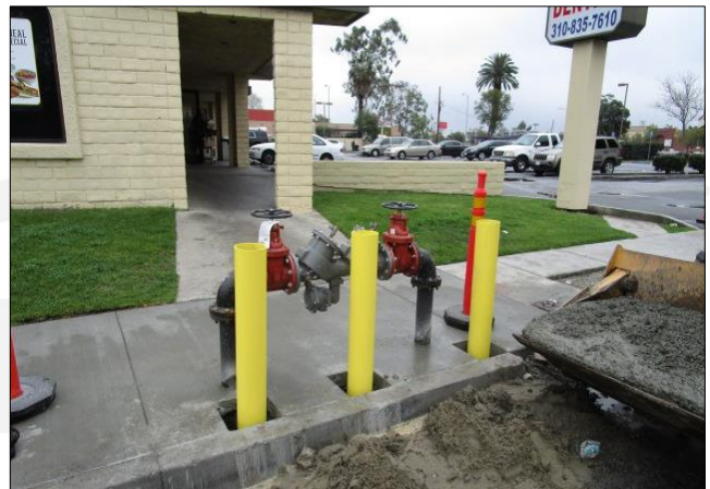
Bollards installed on Main north of Carson.
