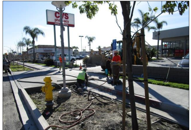
Cleaning driveway culverts.
