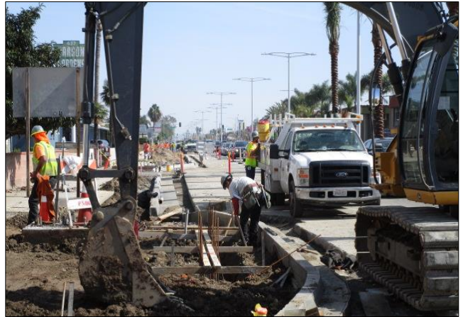
Forming foundation for seat wall east of Figueroa.
