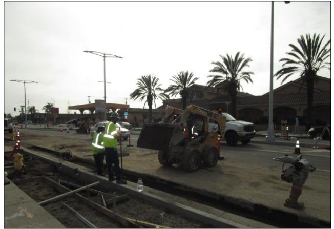
Asphalt concrete placed slots in slots Main to Moneta north side.
