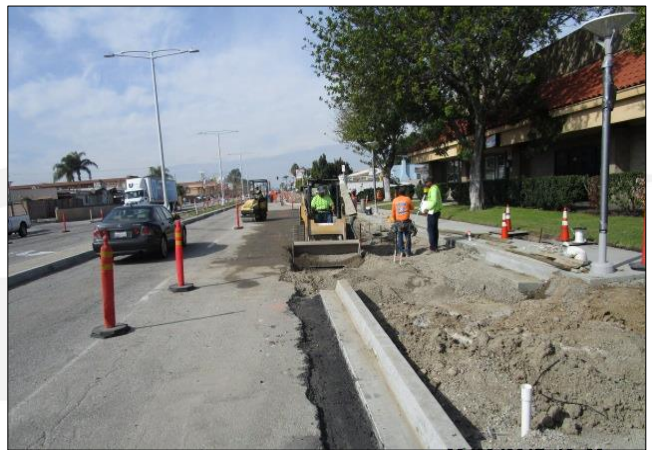
Grading and compacting parkway.
