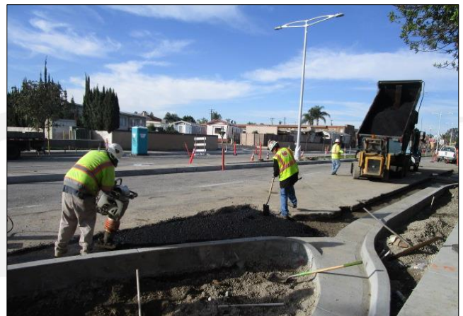
Paving curb slots west of Main.
