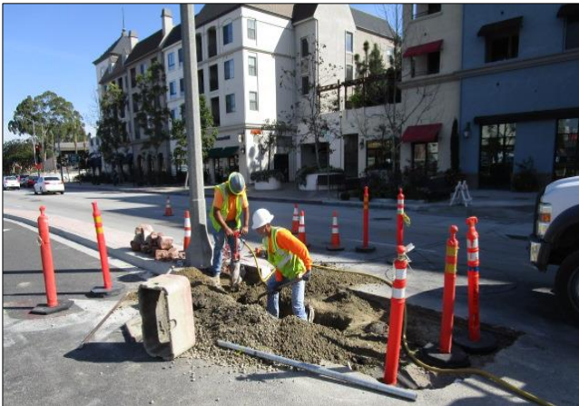
Relocating pull box on Avalon south of Carson.
