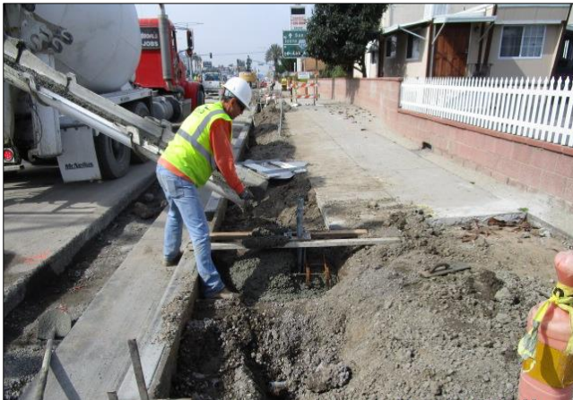
Placing pedestrian light pole foundation east of Figueroa.
