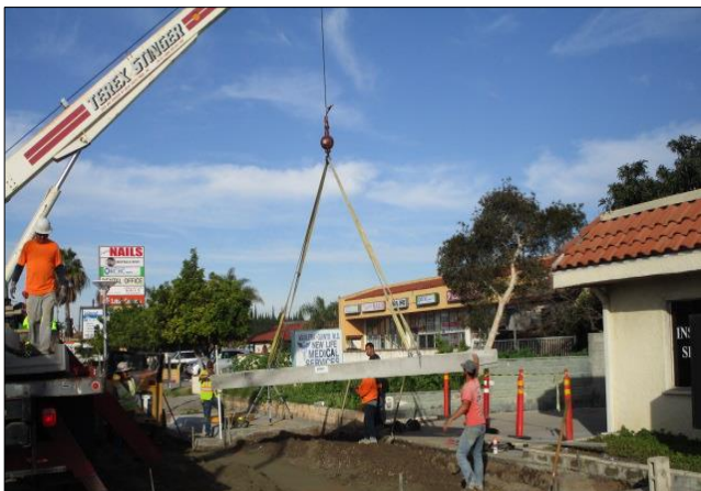
Delivering precast culvert section.
