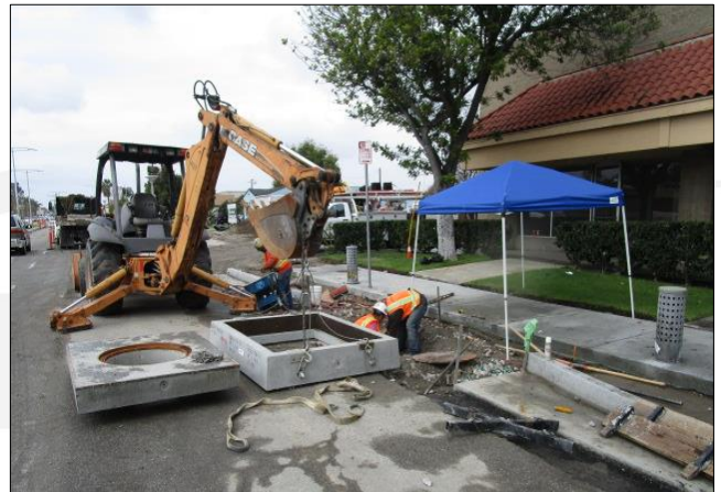
Doty Bros. rebuilding SCE vault.
