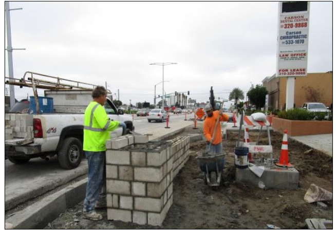
Constructing concrete masonry unit seat wall east of Figueroa.
