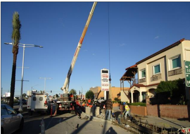
Placing culvert on north side east of Figueroa.
