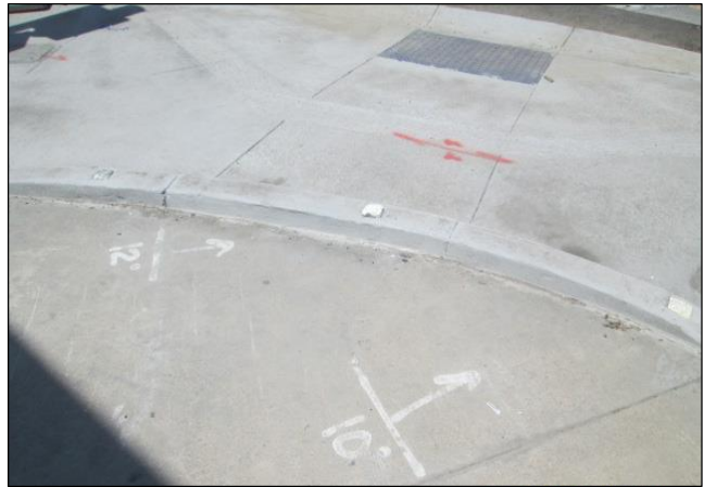
Curb at ADA Ramp Grace and Carson Ready for Hand Rail
