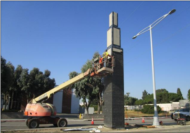
Attaching lath to monument tower.
