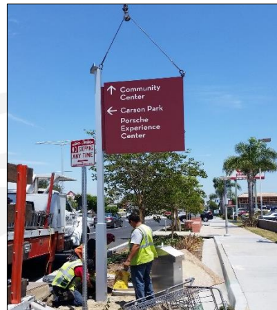
Directional sign placement.
