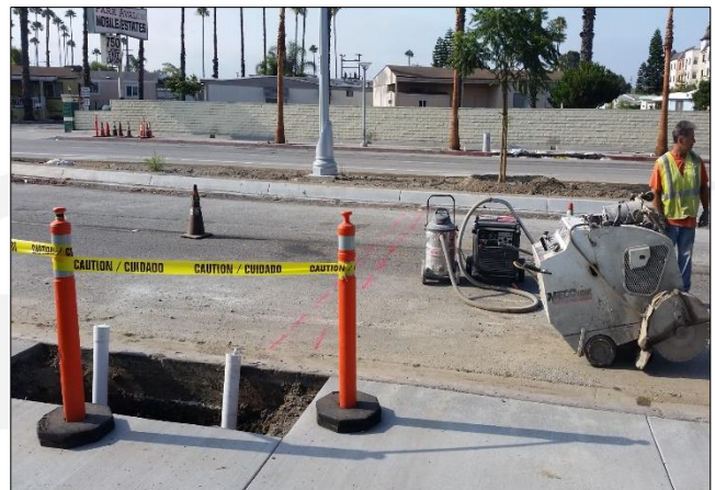
Sawcutting irrigation lateral at Carson St.
