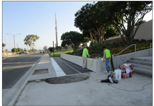
Second coat of stucco on City Hall wall.
