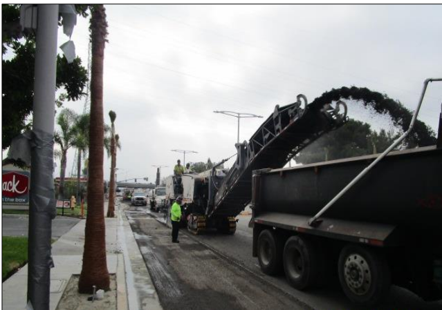
Coldmilling pavement east of Avalon.
