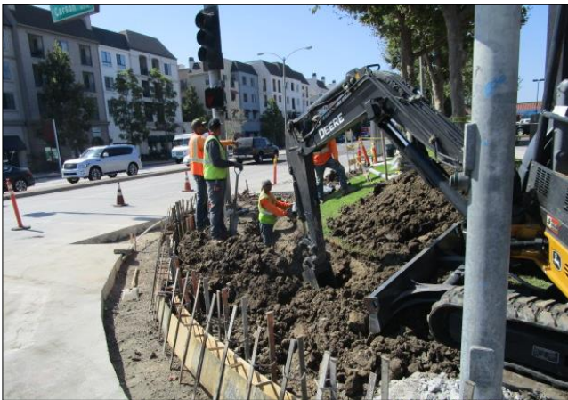
Trenching for traffic signal conduit relocation.
