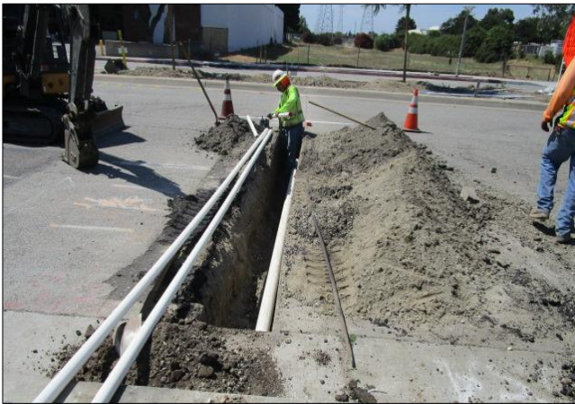
Installing irrigation mainline across Carson.
