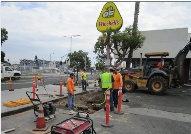
Removing section of driveway, crossgutter at Winchell's.
