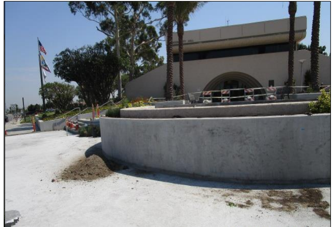
City Hall Attachment at a trench for pipe fitting installation.
