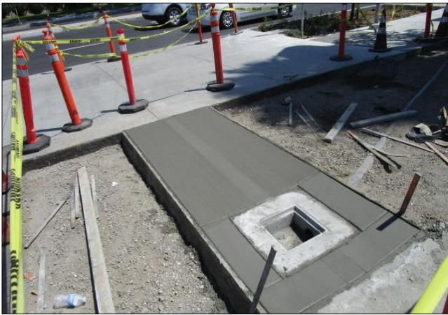
Placed crossgutter and parkway drain the driveway at Winchell's.
