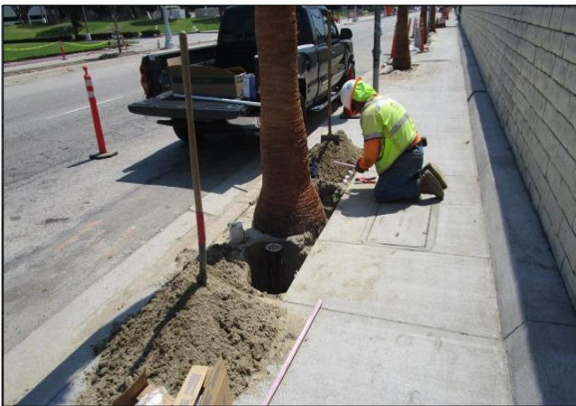
Installing a vigal foot sidewalk on sidewalk of 1405.
