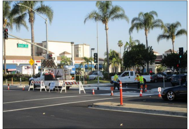
City crew painting crosswalk at Carson and Grace.
