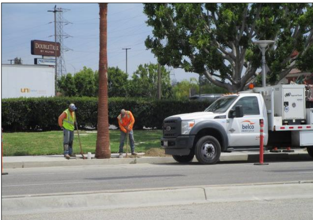
Belco installing uplighting for palm trees.
