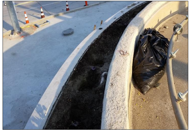
City Hall fountain excavation with pin letters conduit exposed.
