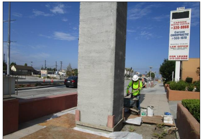
Placing corner tiles on monument tower.
