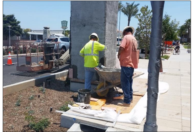
L. Johnson applies stone veneer to monument tower east bound Carson.
