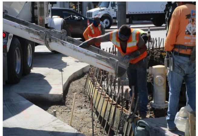
Placing curb and gutter south west corner of Carson and Avalon.
