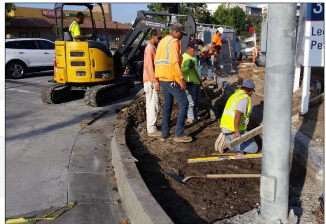
Powell formed/placed PCC curb ramp and paver slab north west corner of Carson.
