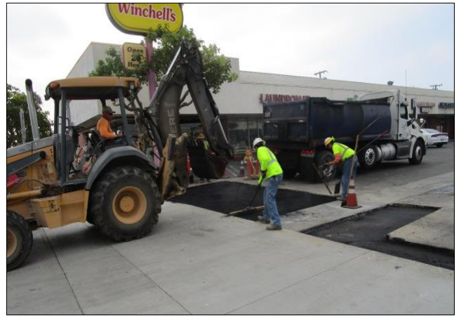
Placing asphalt driveway at Winchell's.
