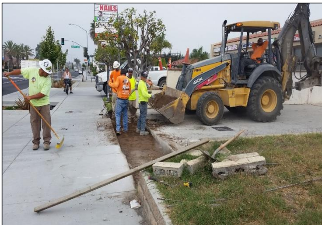
Driveway removals and grading.
