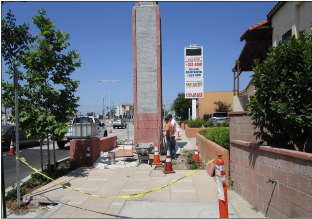
Placing stone on monument tower.
