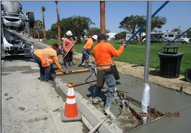
Placing decomposed granite sidewalk in front of Civic Center gaps.
