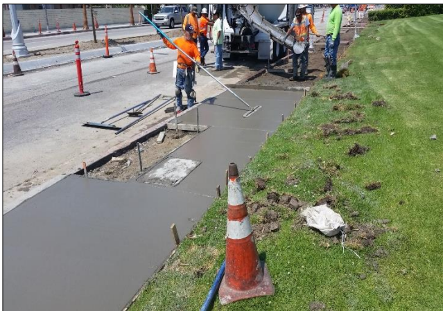
Finishing sidewalk west bound Carson.
