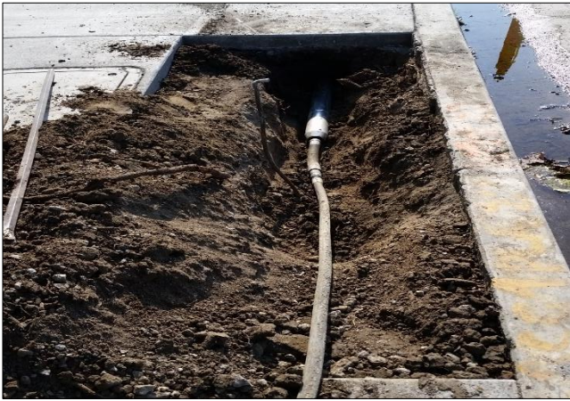
Sierra bores for irrigation sleeves west bound Carson St.
