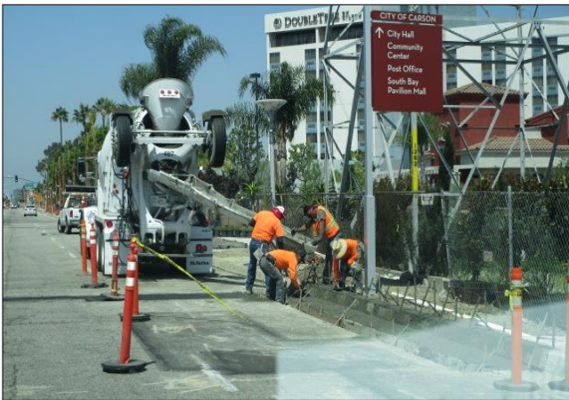
Placing curb and gutter west of I-405.
