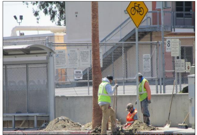
Belco installing palm tree uprights.
