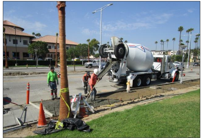
Placing sidewalk on north side at Civic Center.
