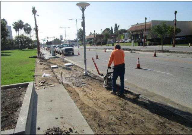
Compacting sidewalk on north side in front of Civic Center.
