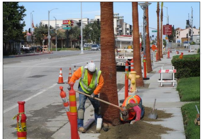
Installing uplights for palm trees east of Avalon.
