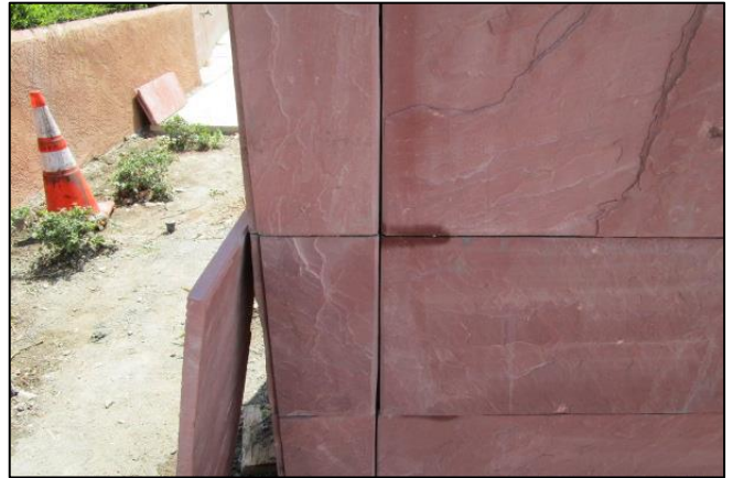
Joints between monument tower stone.
