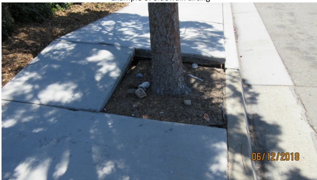
Example of Sidewalk Lifting
