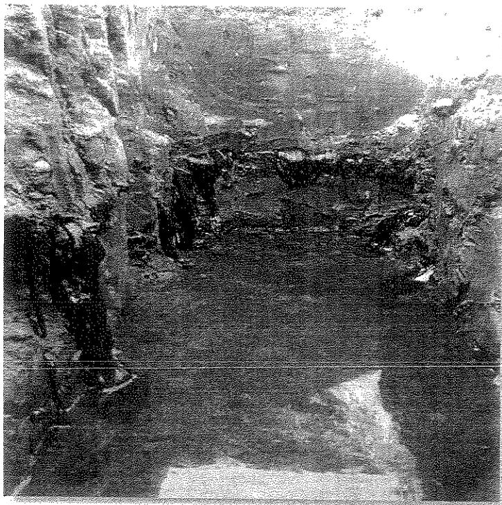
*Figure 2. Photo taken near 317 E 244th Street showing very viscous petroleum oozing out of the soil into a utility trench.*
