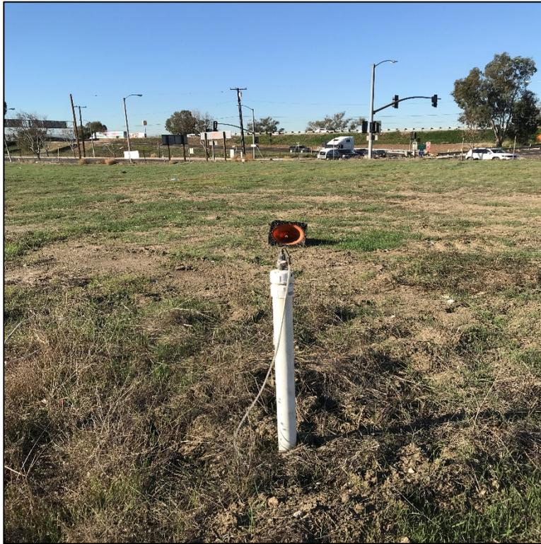
Photograph 5. View to the northwest of the subject site. One of six 2-inch diameter vapor wells can be seen.
