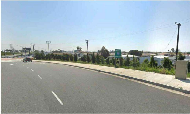
VIEW ON 405 FWY OFF-RAMP LOOKING SOUTHEAST 5
