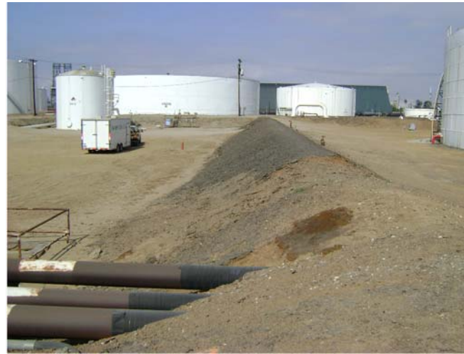
Photo 2: View of site looking west.
