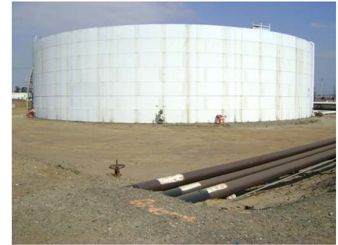
Photo 3: View of site looking northwest.
