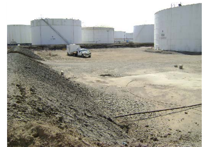
Photo 6: View of site looking northeast.
