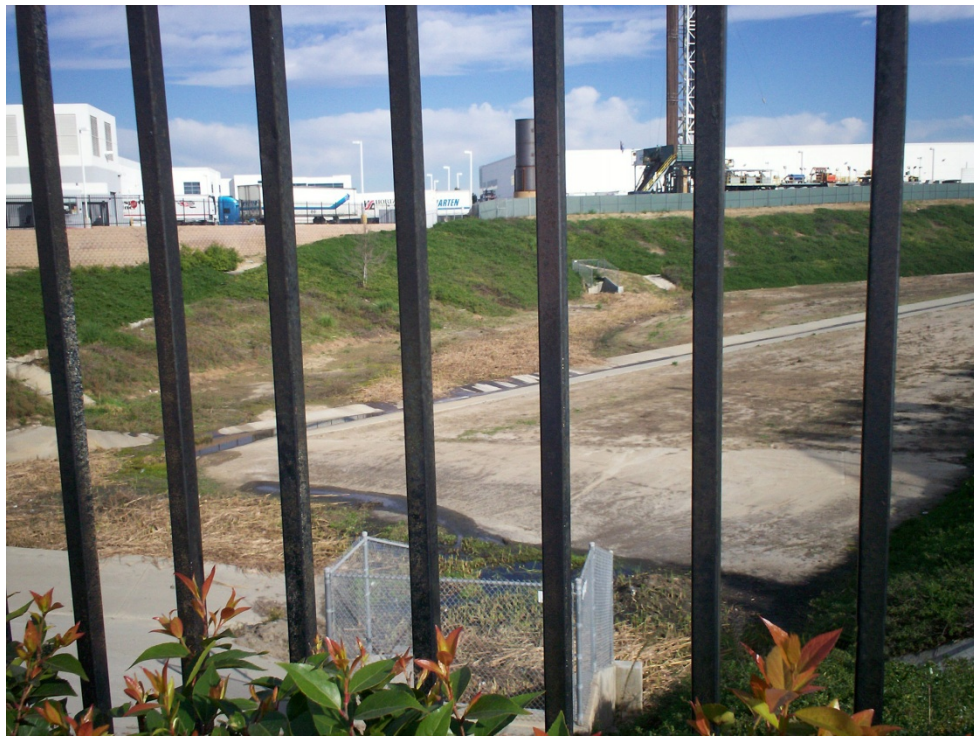
Photo 7: Outfall with ponding and cattails in stormwater basin sediment deposit, facing north-northeast from fence along Beachey Place
