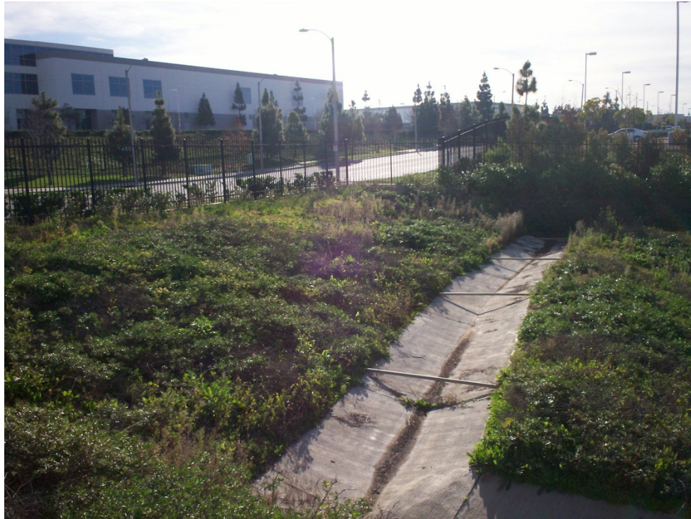
Photo 1: Stormwater basin, facing south at fence along driveway of 18030 Bishop Avenue (approximate address). Side slopes of basin are vegetated with dense, shrubby groundcover and drip irrigation.
