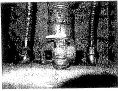
Water heater is braced by wood blocking not metal Water Heater Straps straps. The water heater is tightly secured and does not move. Recommend that a licensed plumber be consulted for further evaluation and repairs.
