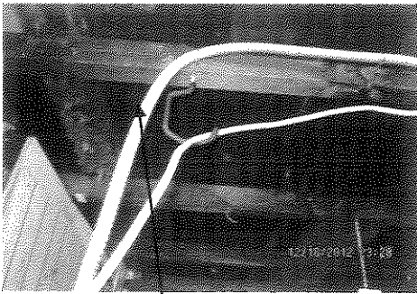
Outlet protective cover damaged Romex cable should be in a conduit
