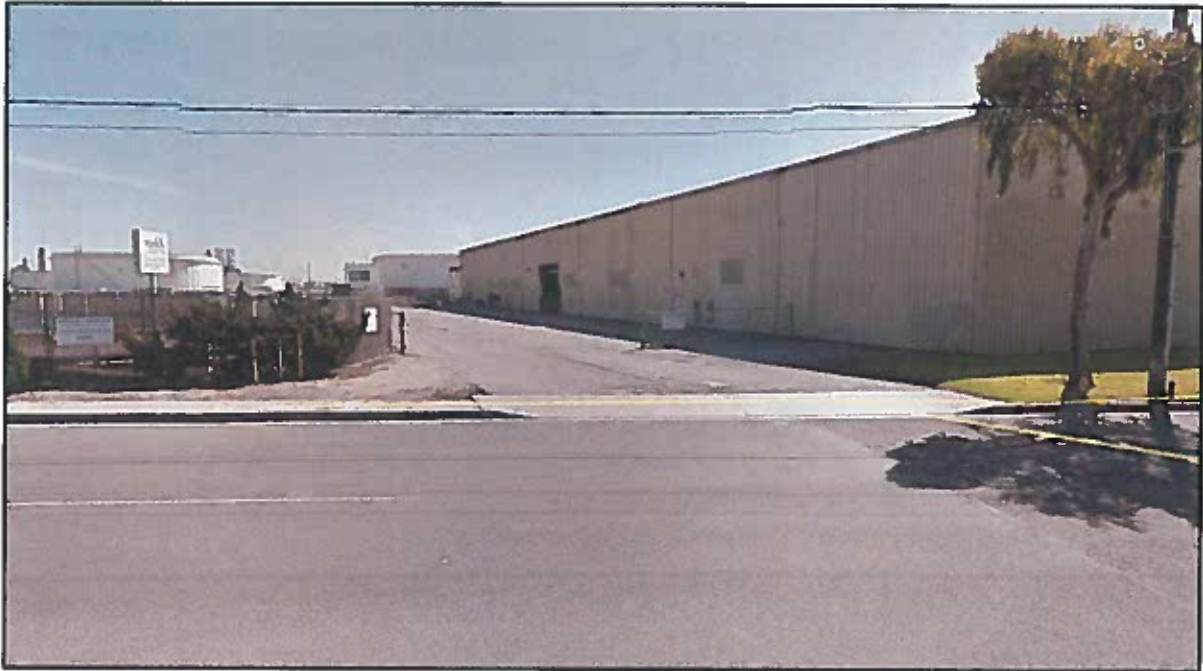
6. SE at site from across Wilmington at 24696 Wilmington Avenue
