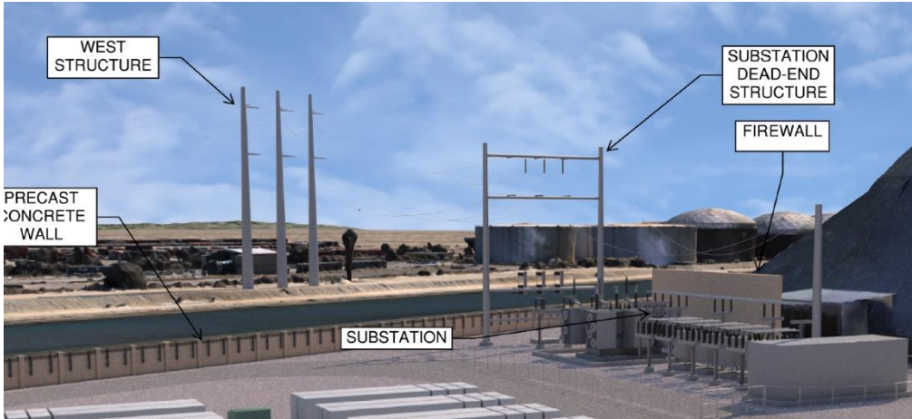
Figure 1b – East View of Project Transmission Poles and Substation
