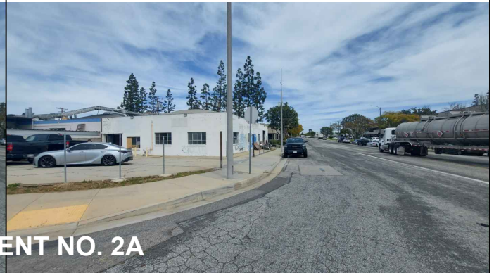
EXTERIOR BUILDING VIEW (LOOKING EAST)
