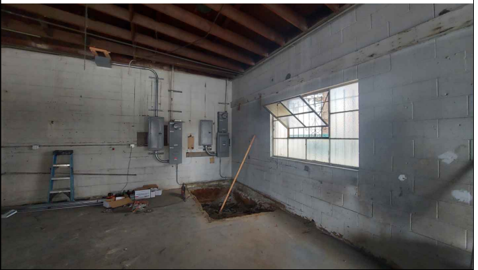
INTERIOR BUILDING VIEW
