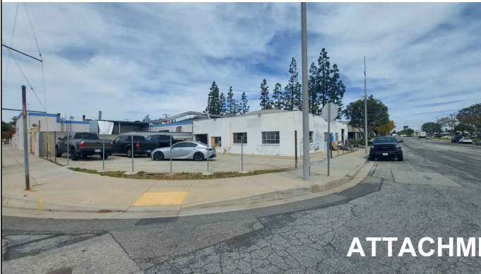
EXTERIOR BUILDING VIEW (LOOKING EAST)
