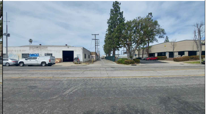
EXTERIOR BUILDING VIEW (LOOKING NORTH)
