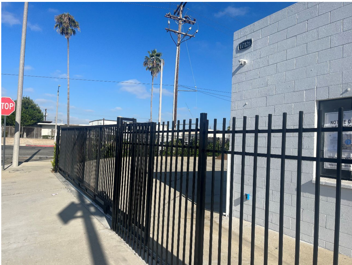
Figure 6 - Address Identification, Parking Lot Driveway Gate Facing Walnut
