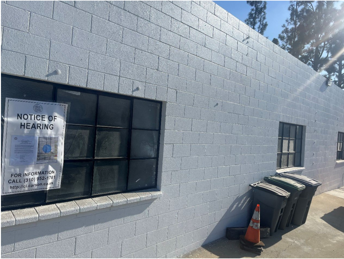
Figure 3 - Building exterior facing Walnut
