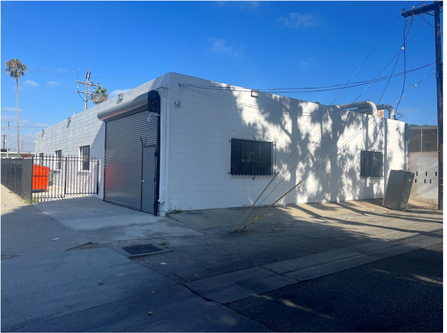
Figure 7 - Rear and Side Building Exteriors
