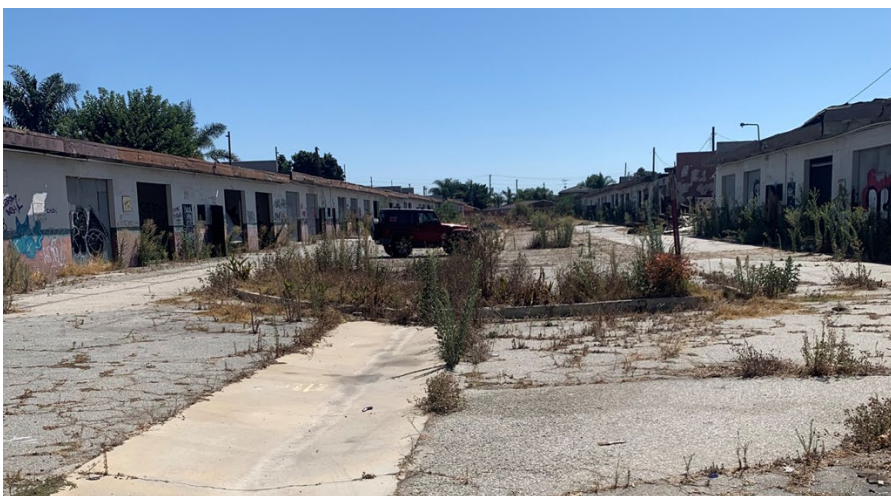
South View from Carson Street
