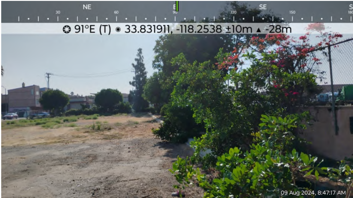
Photo 5. View from project site southwest corner, facing east.
